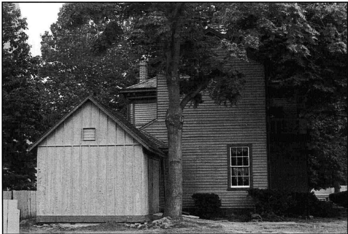
Figure 1. The Harriet Dean House as it appeared in 1991: viewed from the southeast (top) and viewed from the west (bottom).
