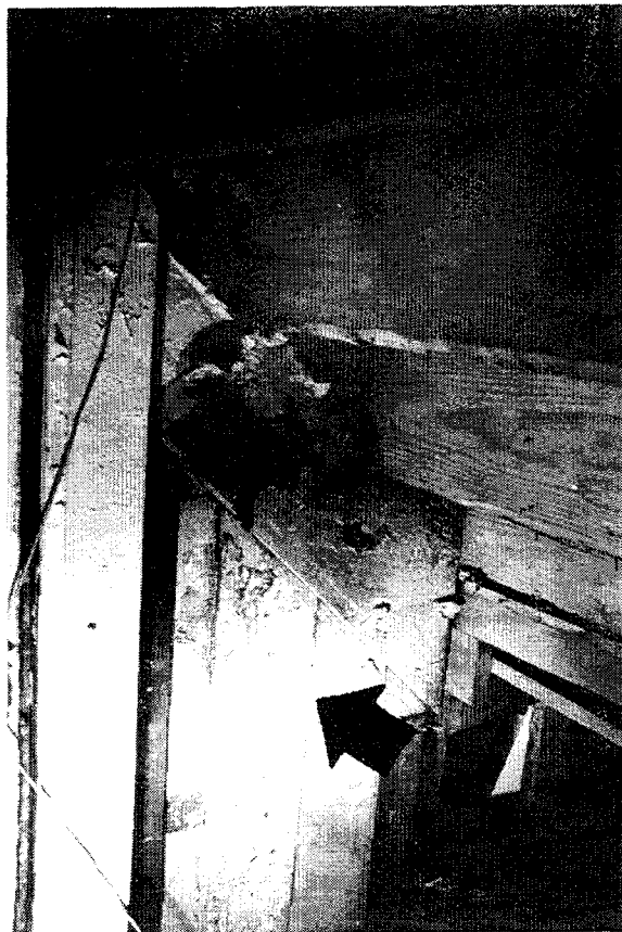
FIGURE 3.22: ORIGINAL STAIR STRINGER
