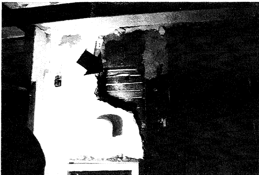
FIGURE 3.24: CUT-OUT IN THE SHEATHING
