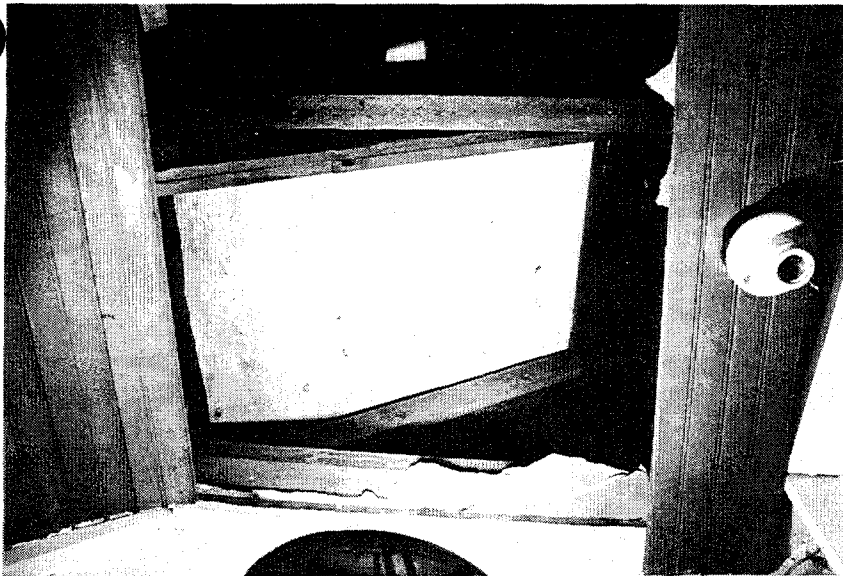
FIGURE 3.29: ROOF FRAMING AT NON-EXTANT CHIMNEY
