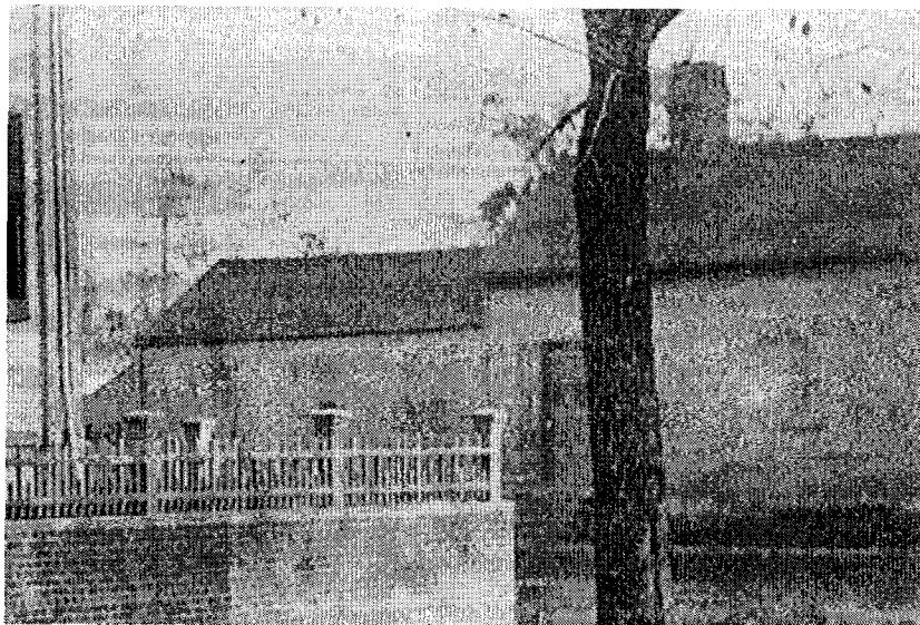
FIGURE 2.17: Circa 1888-1895 PHOTOGRAPH (FROM THE NORTHWEST) This photograph shows most of the north elevation of the Arnold House prior to its relocation on the site. At the bottom is an enlarged portion of this photograph of the Arnold House. Note the open leaf of the door shutter and the white porcelain door knob.
