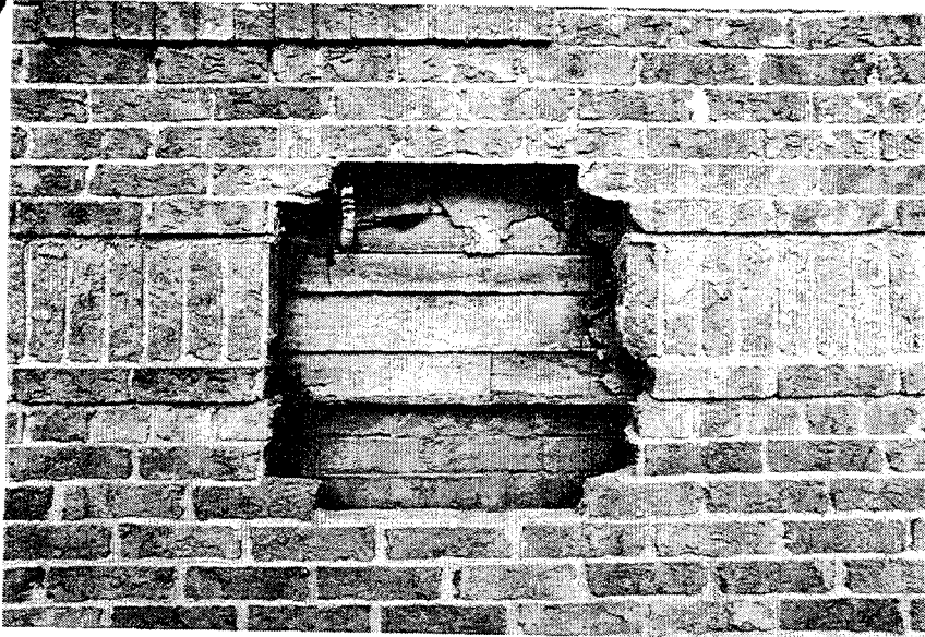
FIGURE 3.5: CLAPBOARD SIDING
