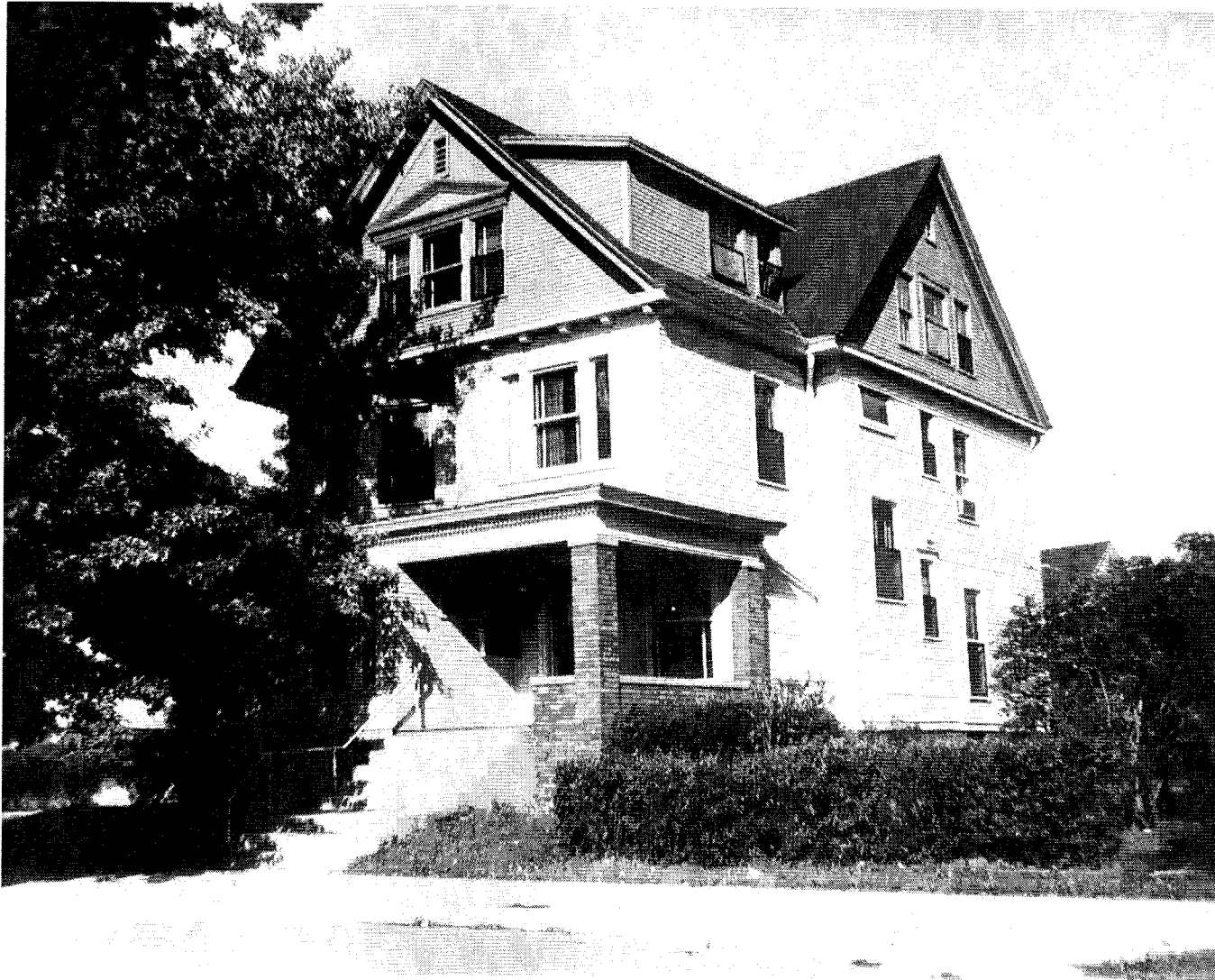
FIGURE 2.24 REBECCA COOK HOUSE AT 500 SOUTH EIGHTH STREET (FROM THE SOUTHWEST) This photograph of the Rebecca Cook House (circa 1900) was taken after the Lincoln Home National Historic Site was authorized. This house was demolished by the National Park Service after 1978.
