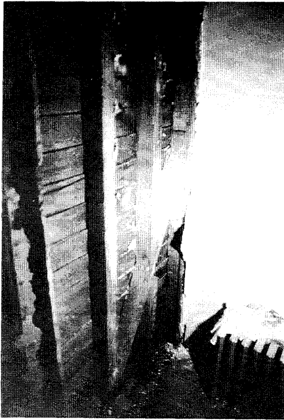
FIGURE 3.19: CORNER BRACING
