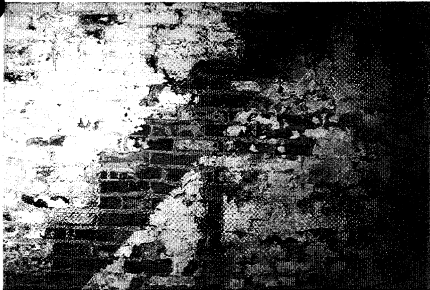
FIGURE 3.11: EVIDENCE OF BASEMENT STAIR
