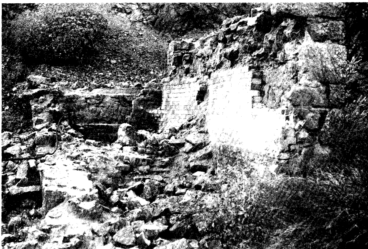
Plate 12. Homestake Mine. Boiler foundation.
