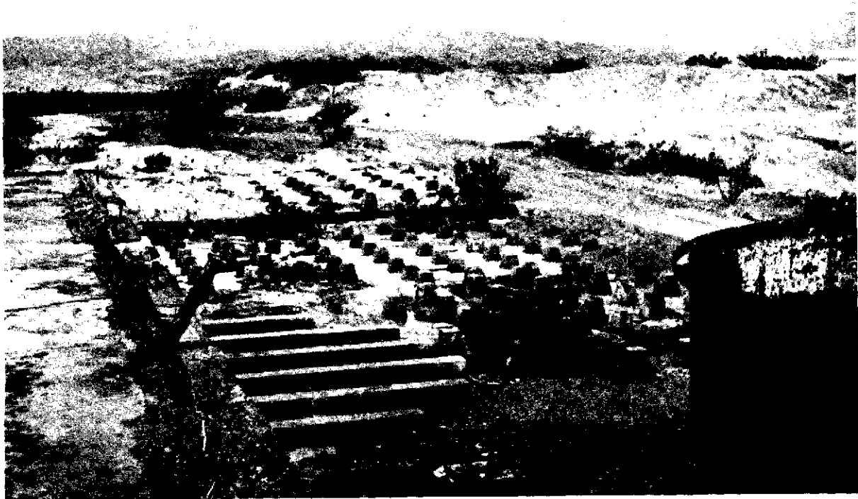
Plate 10. Katherine Mill Site. Foundations for tanks and vats.
