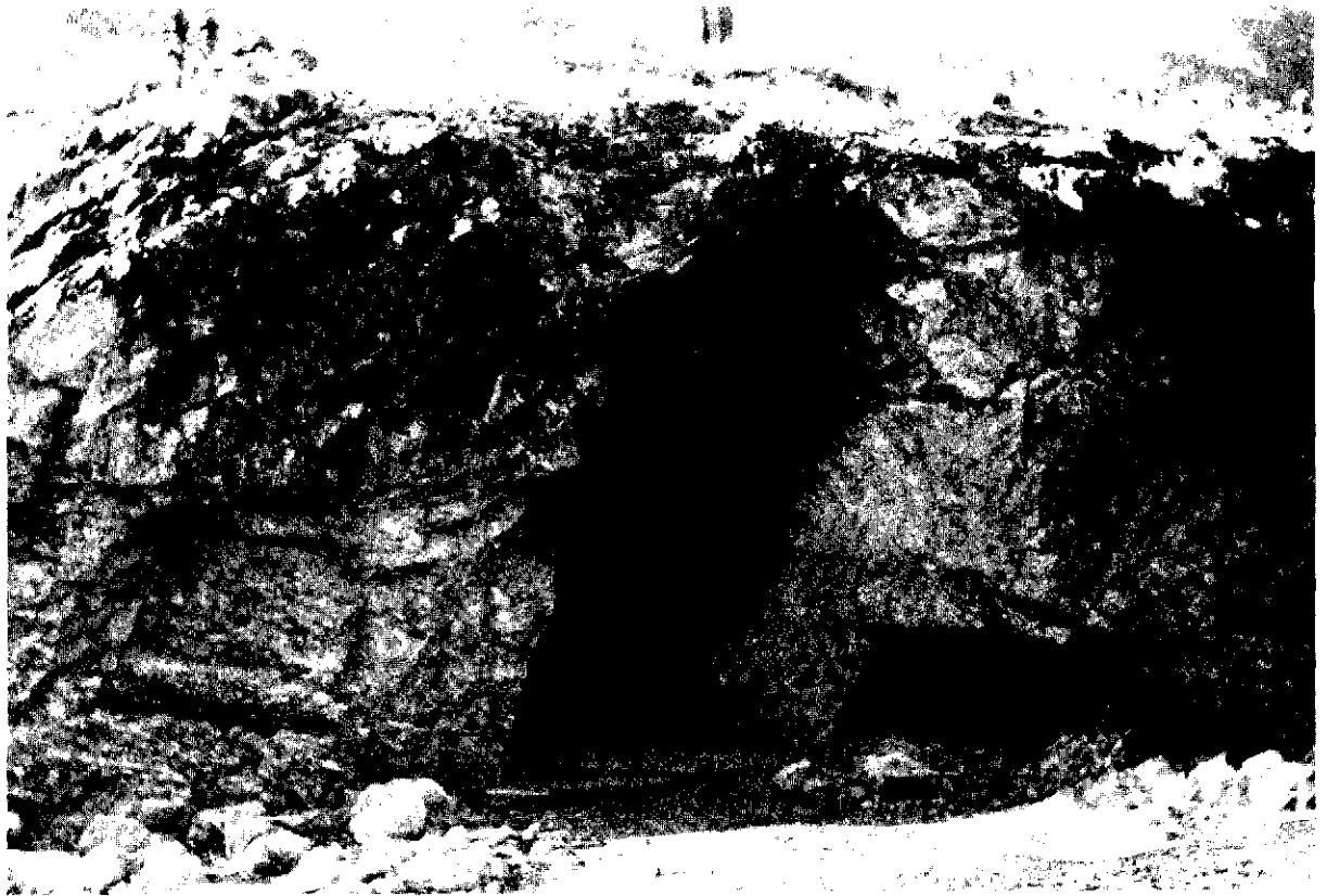
Plate 4. Unidentified Mine. Short tunnel excavated with two rooms. Flue extends above. Evidence of coal oil fire.
