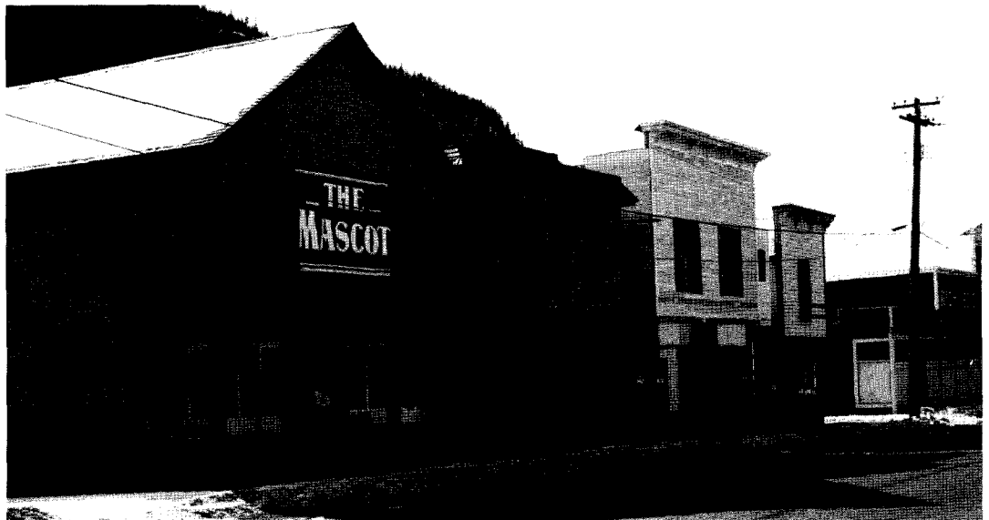
Figure 2. Photograph of the National Park Service buildings on the north half of Block 35. The Mascot Saloon Group is the three buildings on the left: the Mascot Saloon, the Pacific Clipper Line Office, with the second story bay window, and Hern's Liquor Store next door. Boas Tailor and Furrier Shop is the larger, two story structure to its right, and the smaller building next to the alley is the Verbauwhede Cigar Store and Confectionery (April 1986).
