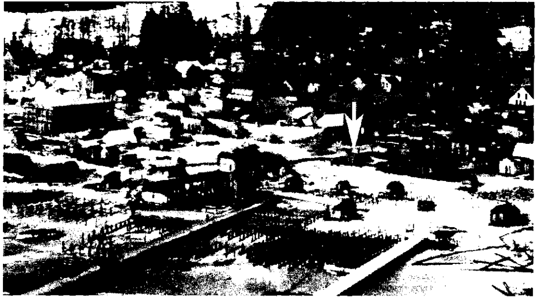
Figure 24. Photograph dated by the photographer to January 1898, taken from above Moore's Wharf. Note the distance from Broadway to the small NT & TC ticket office building (indicated by the white arrow). The Klondike Trading Company is under construction at the corner of Third and State (Credit: University of Washington, Special Collections Division, Seattle, Washington / Hegg 141 / Webster & Stevens 282.a; KLGO SO-17-256).
