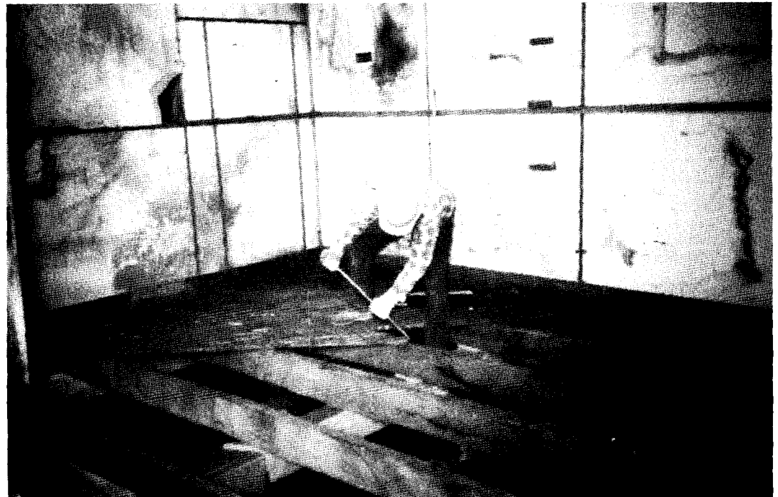
Figure 64. Photograph of a workman removing the floor in a back room of the Mascot Saloon Group
