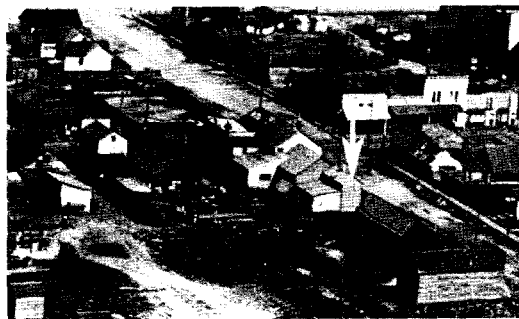
Figure 46. Photograph taken on May 31, 1905. The icehouse added by Reinert in the fall of 1904 (arrow) is probably the northern-most and taller of the two outbuildings, the better to trap cold and to vent heat (Credit: Sheldon Museum & Cultural Center, Haines, Alaska / Case & Draper 195; KLGO 50-54-1018).
