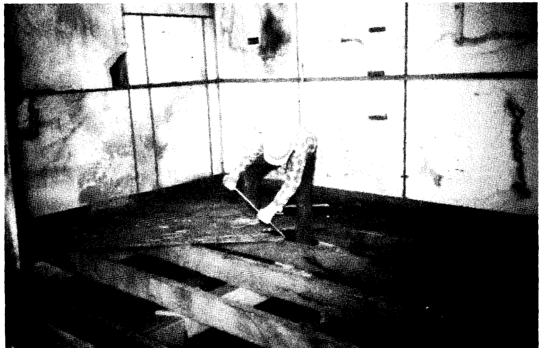
Figure 64. Photograph of a workman removing the floor in a back room of the Mascot Saloon Group
