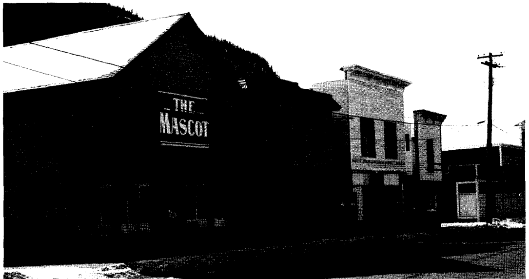
Figure 2. Photograph of the National Park Service buildings on the north half of Block 35. The Mascot Saloon Group is the three buildings on the left: the Mascot Saloon, the Pacific Clipper Line Office, with the second story bay window, and Hern's Liquor Store next door. Boas Tailor and Furrier Shop is the larger, two story structure to its right, and the smaller building next to the alley is the Verbauwheide Cigar Store and Confectionery (April 1986).
