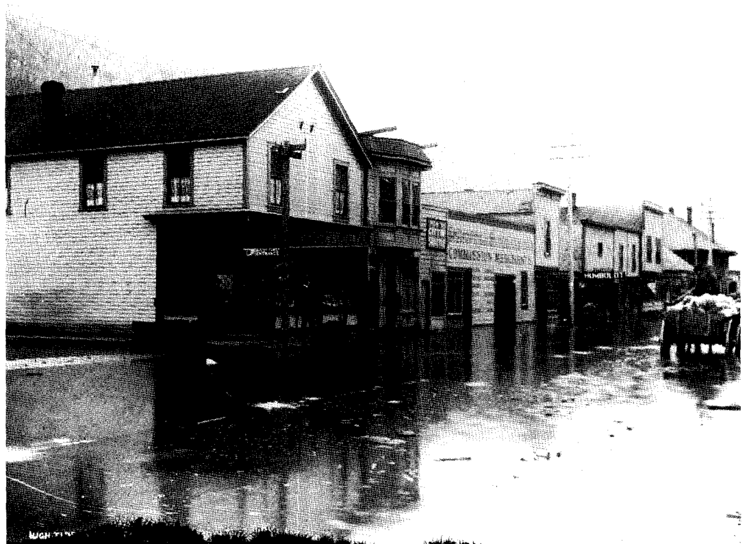
Figure 41. A photograph of the front of the Mascot Saloon during the high tide of October 28, 1901. Note the ripple lines indicating that water is running downwards under the buildings along the east side of Broadway, rather than along the length of Broadway (Credit: Alaska State Library – Historical Collections, Juneau, Alaska / PCA-01-1703; KLG0 B1-36-1638).
