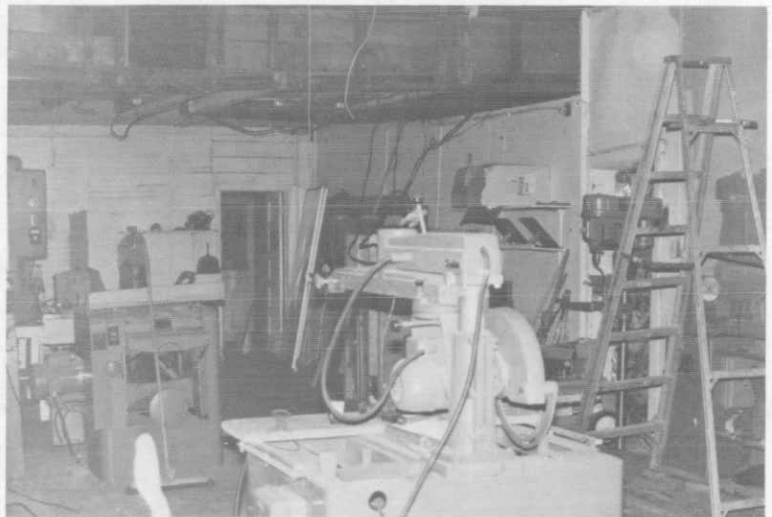
Photograph 47. Room 102, northwest corner.
