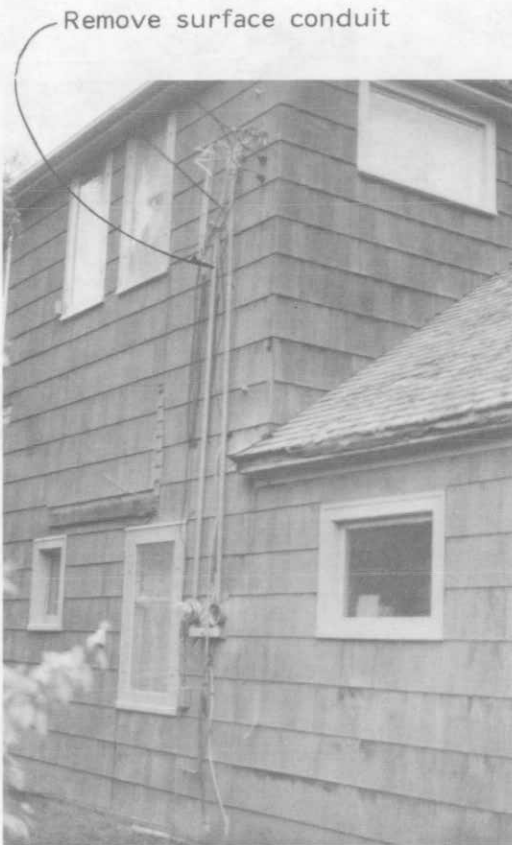
Photograph 8. West wall detail.
