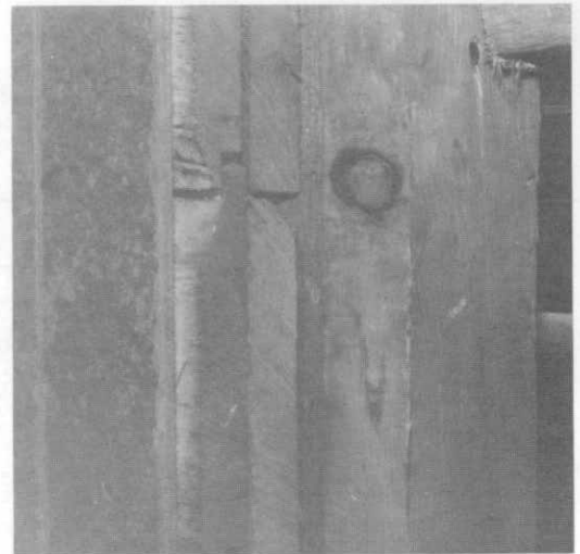
Photograph 37. South addition/main building wall joint.
