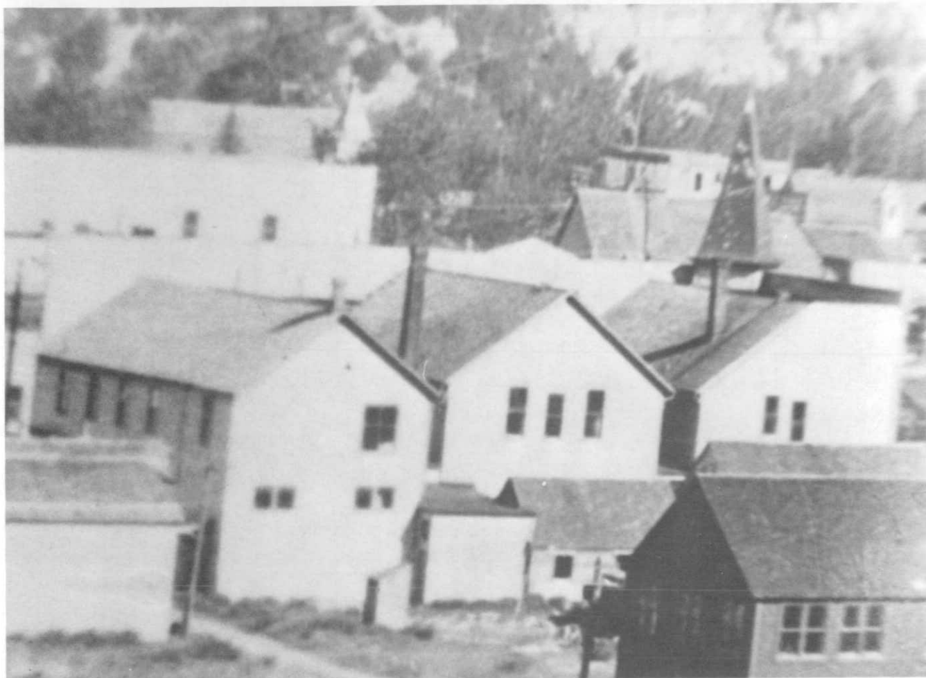
Photograph 7. Detail from a ca. 1916 photograph. Note modification of east first floor windows and addition of second floor window.
