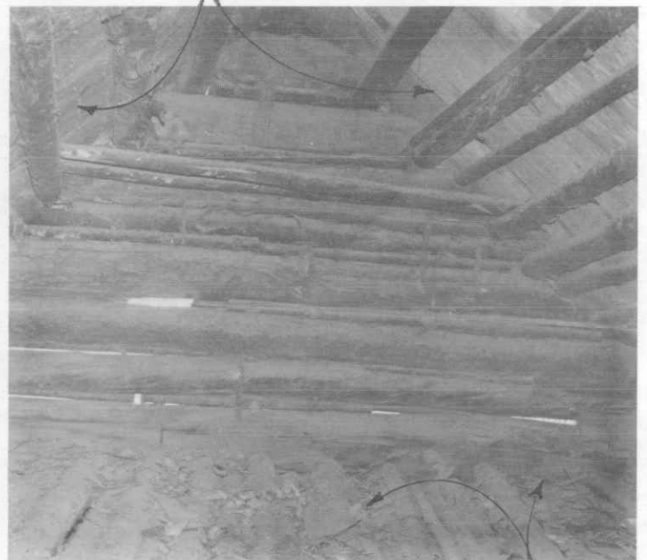
Photograph 78. Attic, south end.
