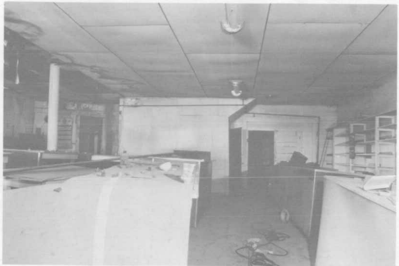
Photograph 35. East wall, as found conditions, 1978.
