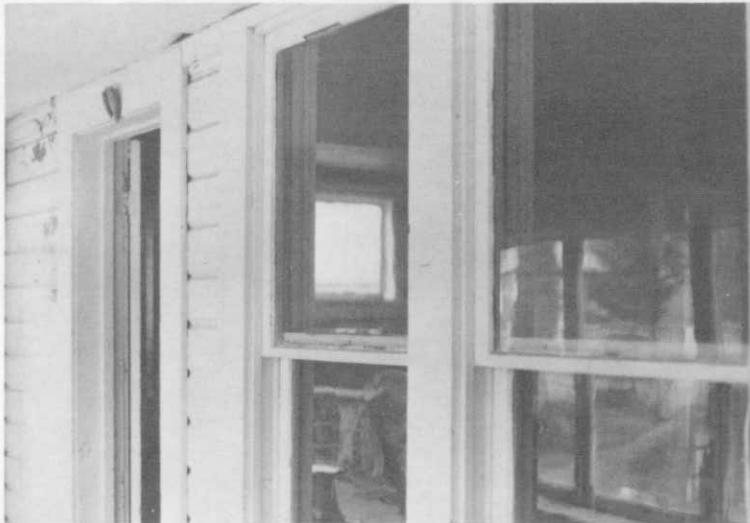
Photograph 49. South porch, north wall.
