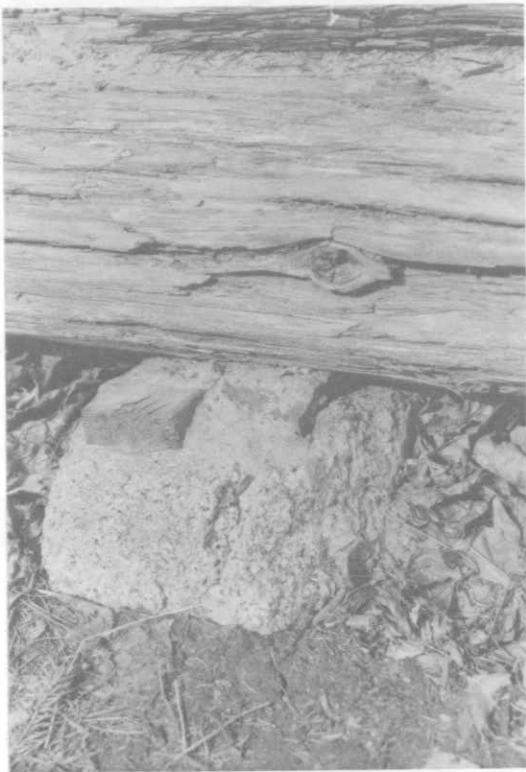
Photograph 68. Moore Cabin, east wall stone support. April 1981.
