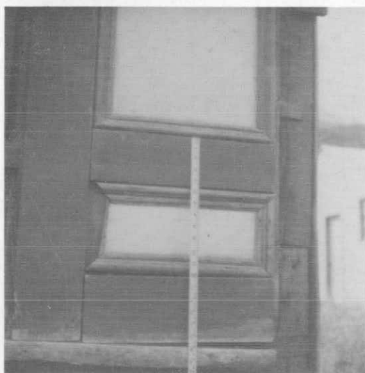
Photograph 23. Southwest panel detail.
