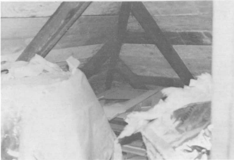
Photograph 36. South addition attic.
