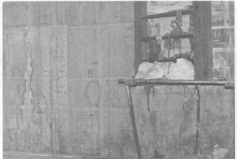
Photograph 74. Interior, east wall.
