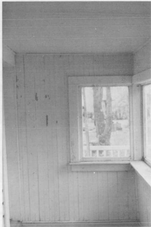
Photograph 51. South porch, east wall. June 1981.
