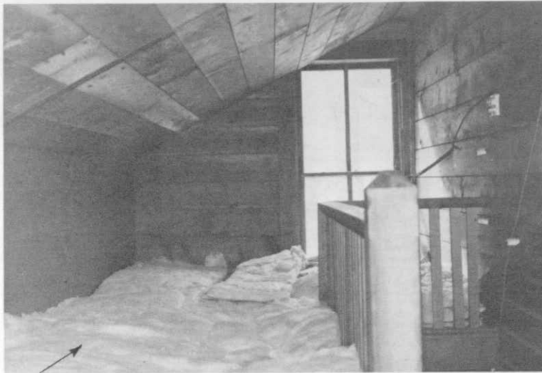
Photograph 56. Attic hall, east end.
