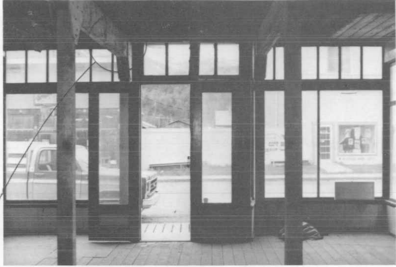
Photograph 19. Main room, first floor.
