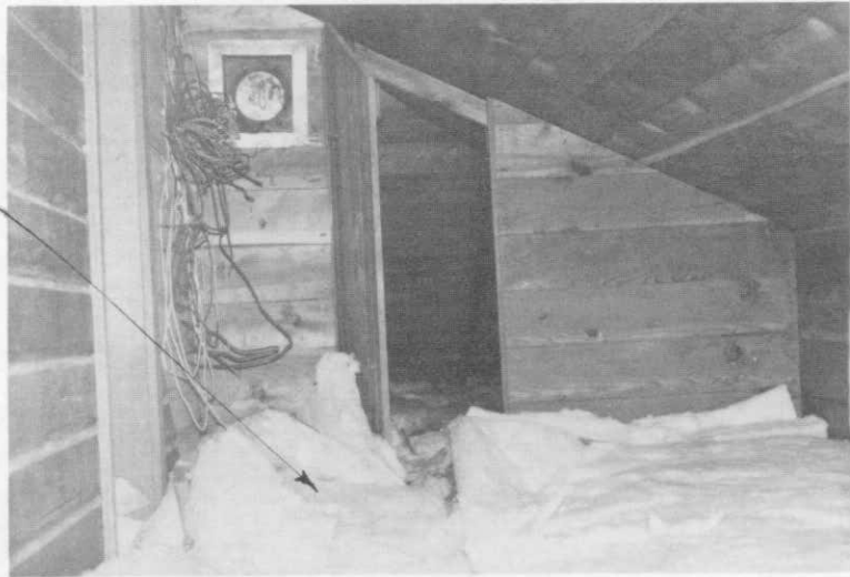
Photograph 57. Attic hall, west end.
