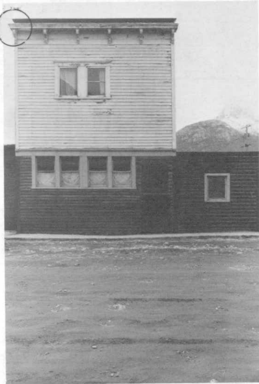
Photograph 32. Ca. 1905 and 1943 additions. North elevation. N.P.S. photograph by T. Busch, Oct. 1977.
