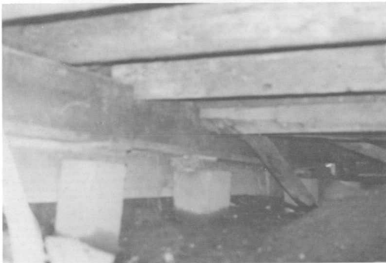
Photograph 38. Crawlspace, west portion.
