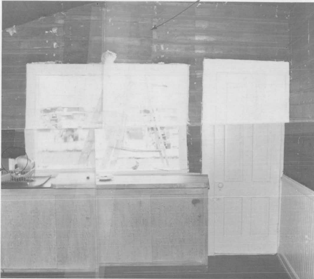
Photograph 38. South wall of kitchen. June 1981.
