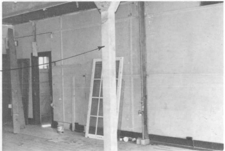
Photograph 23. Main room, view toward southeast corner.
