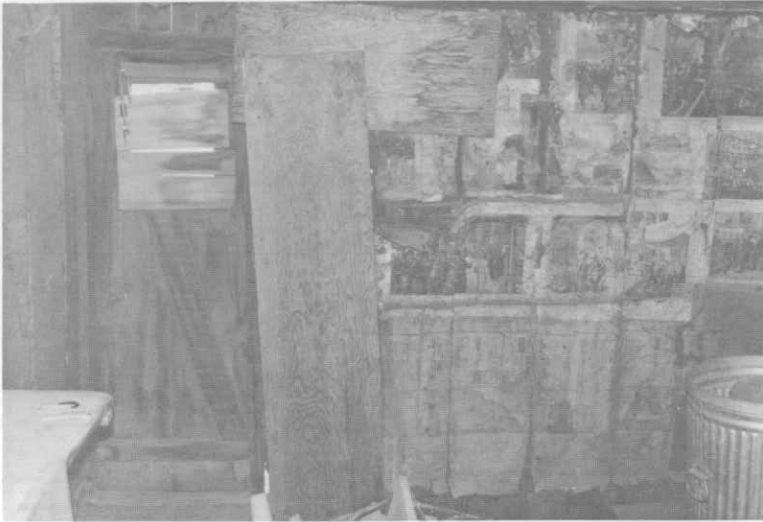
Photograph 73. Interior, south wall.
