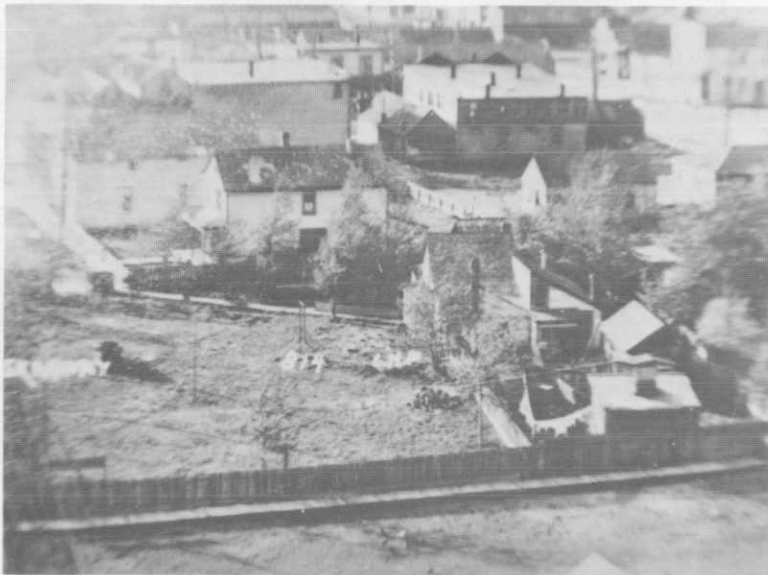
Photograph 16. Detail from a ca. 1910 photograph. View from east. Note corbelled chimney cap at the southeast chimney and two additional flues extending from east end of roof.
