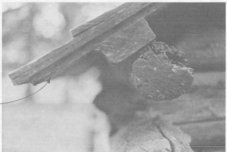
Photograph 72. Moore Cabin, northeast eave detail.
