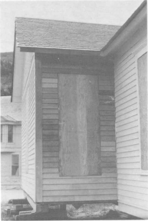
Photograph 12. Partial west elevation.
