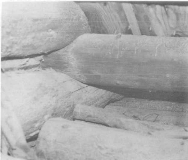
Photograph 77. Attic joint detail, northeast corner.
