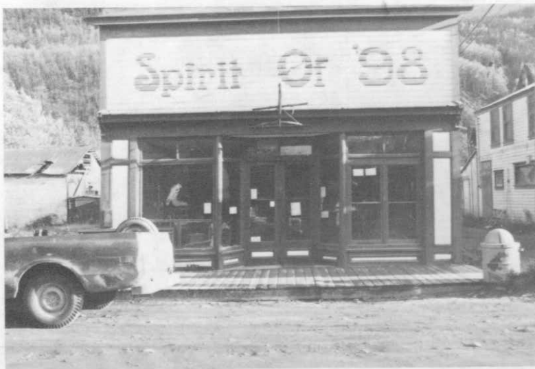
Photograph 16. 1977. West elevation on original site.
