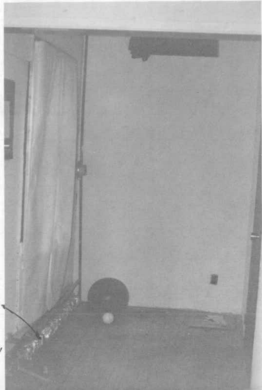
Photograph 30. Northwest bedroom, second floor.
