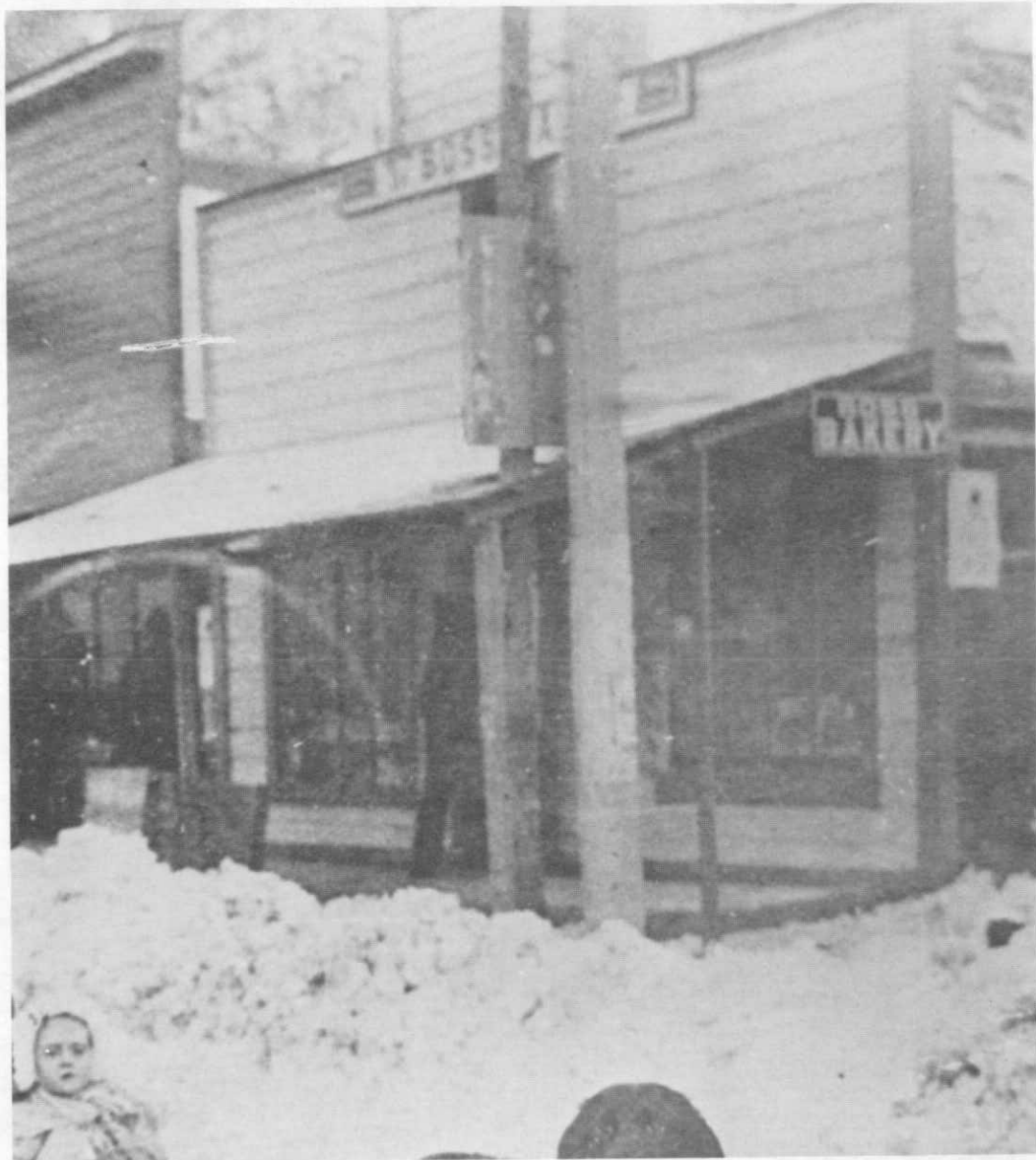
Photograph 7. Detail from a ca. 1900 photograph.
