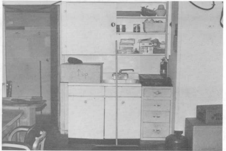
Photograph 51. Room 104, south wall.
