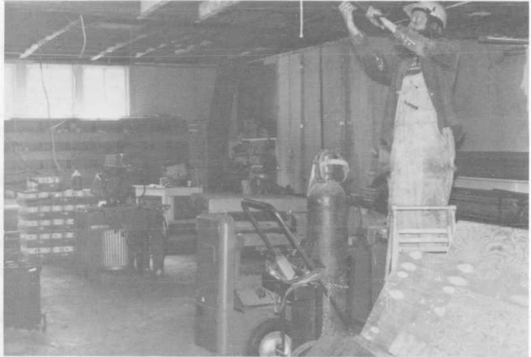
Photograph 45. Southeast portion, room 102.
