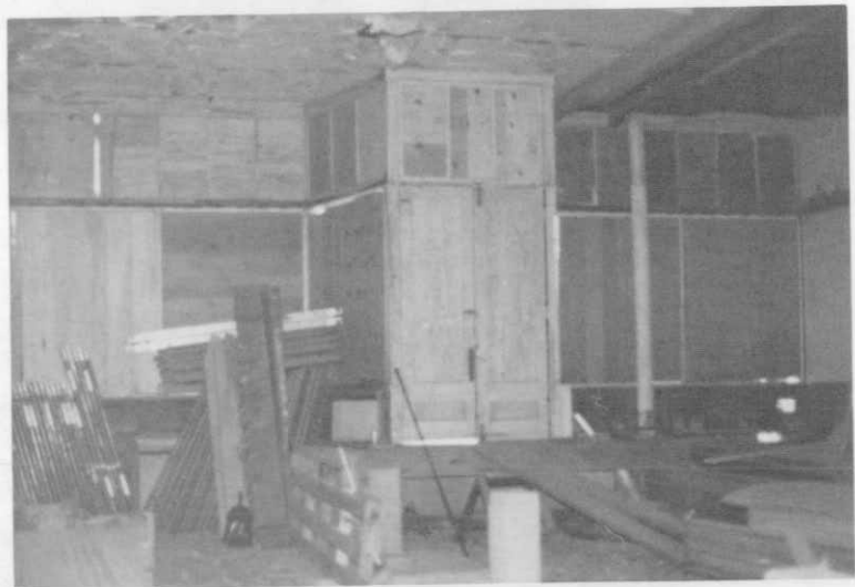
Photograph 28. 1981. After floor removal.
