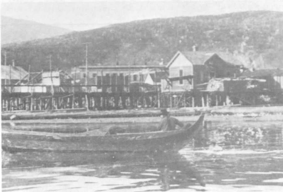
Photograph 1. Ca. 1901. East elevation (now west) prior to addition.
