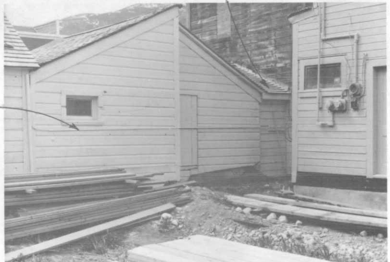
Photograph 19. Partial north elevation.
