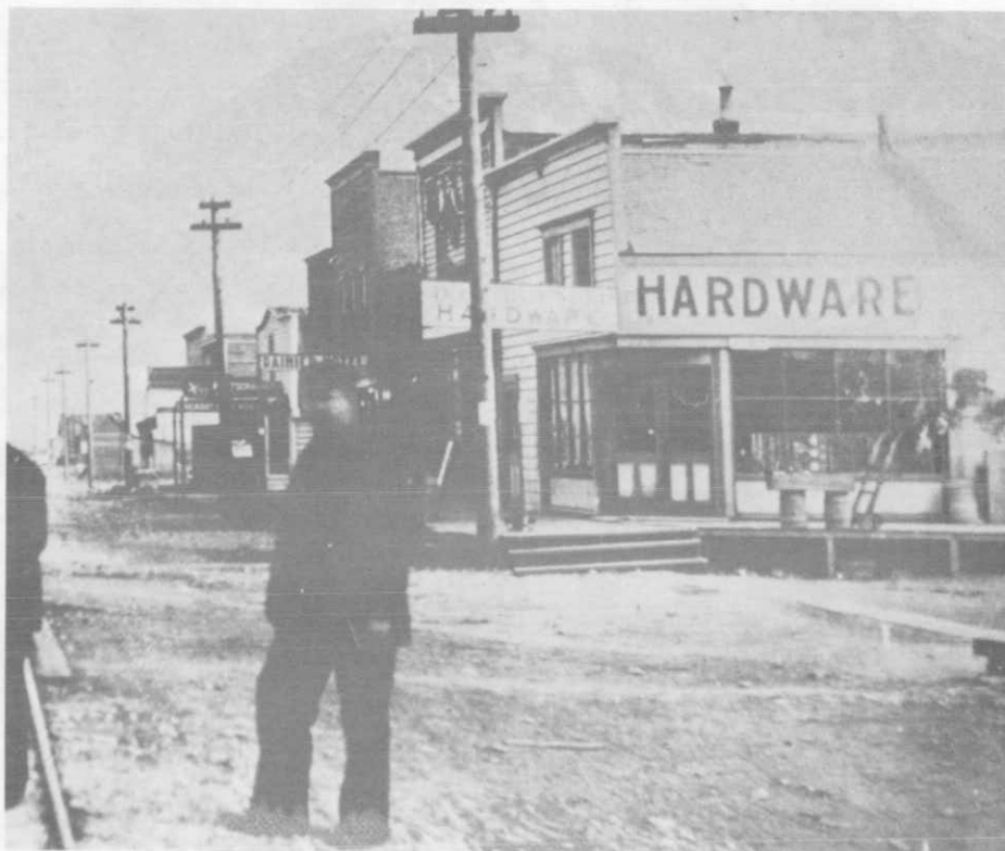
Photograph 7. Detail from a ca. 1900 photograph. View from northeast.
