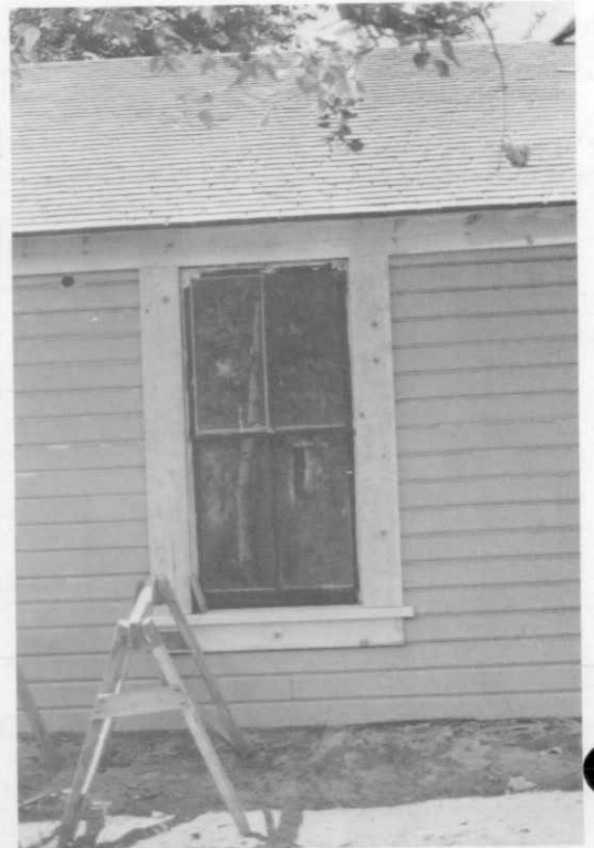
Photograph 29. Restored window trim detail.
