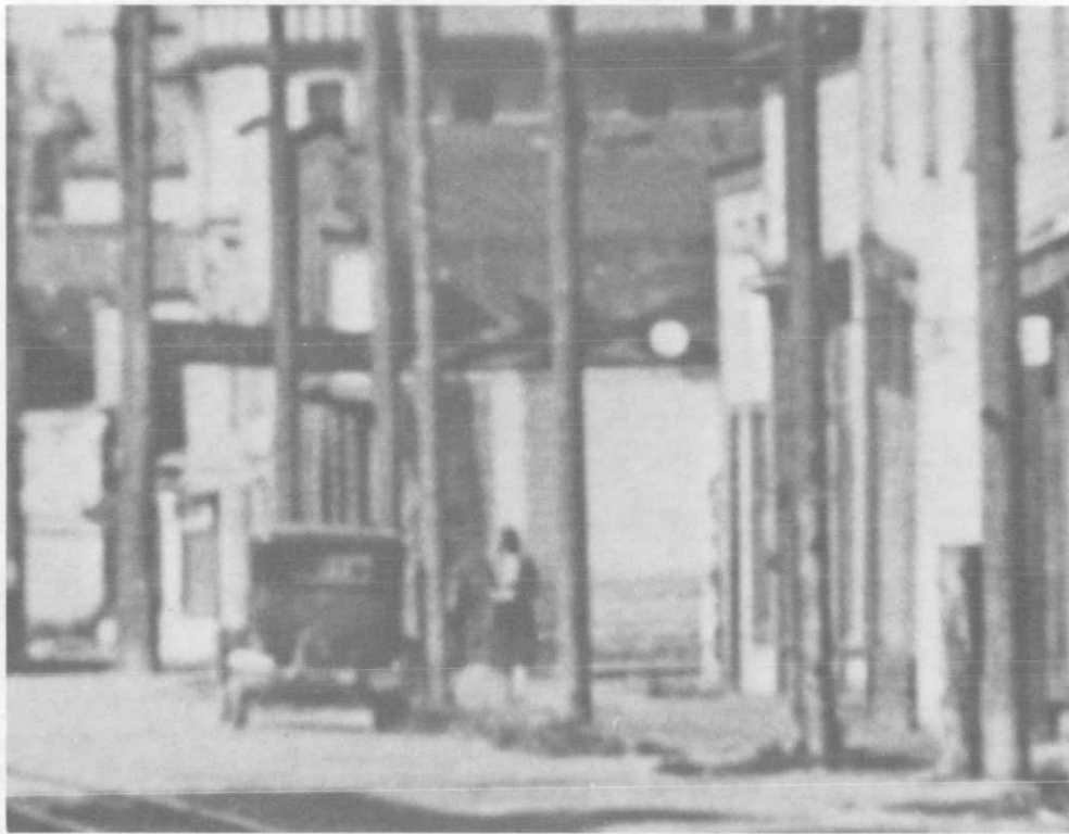
Photograph 18. Detail from a ca. 1920 photograph. Note whiskey advertisement had been painted over.
