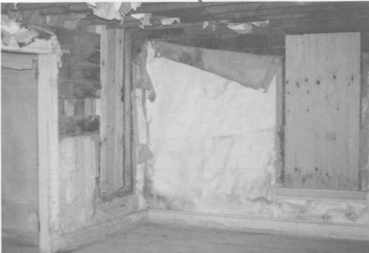
Photograph 20. Northwest corner, room 1.
