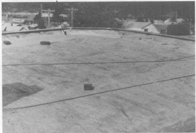
Photograph 39. Second story roof, ca. 1905 addition. View toward southwest.
