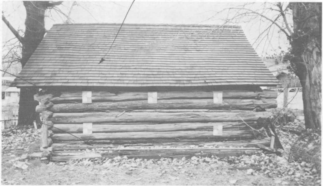
Photograph 66. Moore Cabin, east elevation.
