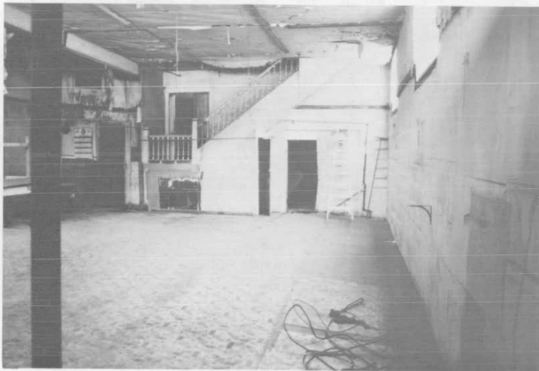
Photograph 36. 1978. East wall after removal of debris and fiberboard finishes.
