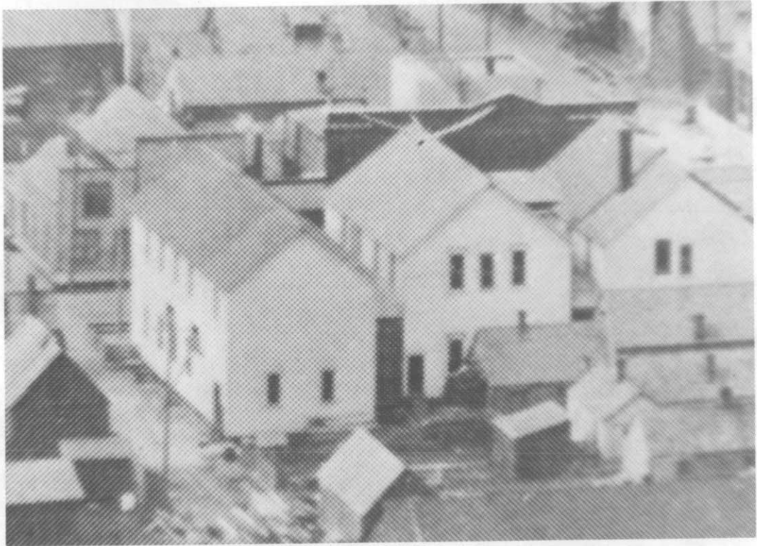
Photograph 2. Detail from a summer 1908 photograph.
