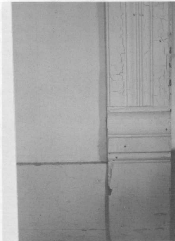
Photograph 45. Trim detail, parlor, east wall.
