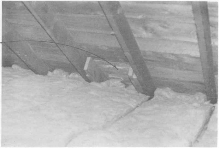
Photograph 40. East central portion.
