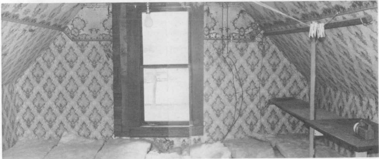
Photograph 53. Attic room, south wall. June 1981.
