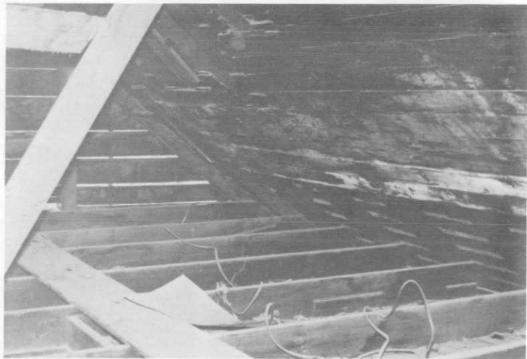
Photograph 34. Attic, southeast corner.
