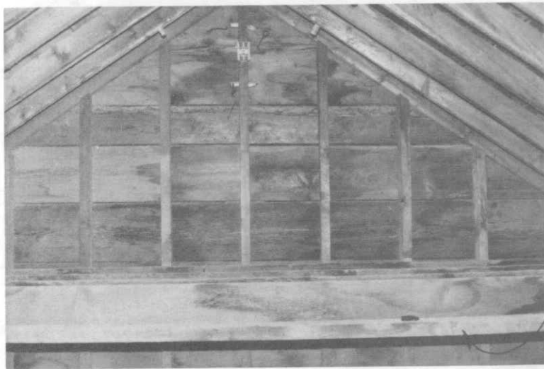
Photograph 25. East attic, south end.
