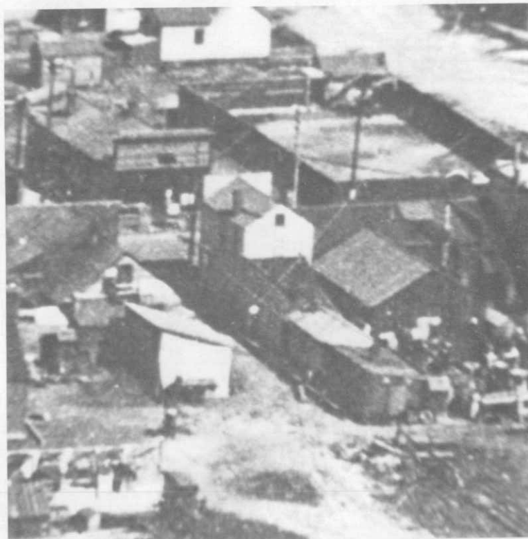
Photograph 4. Detail from a May 31, 1905 photograph. View from southeast.
