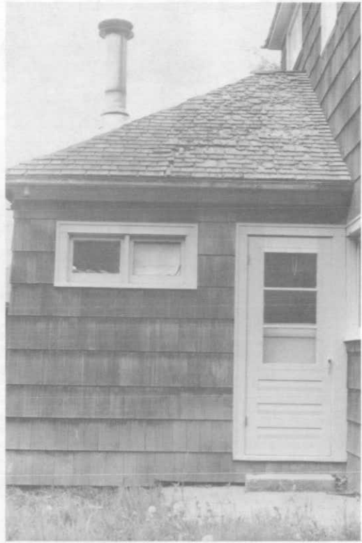
Photograph 14. East wall, south addition.
