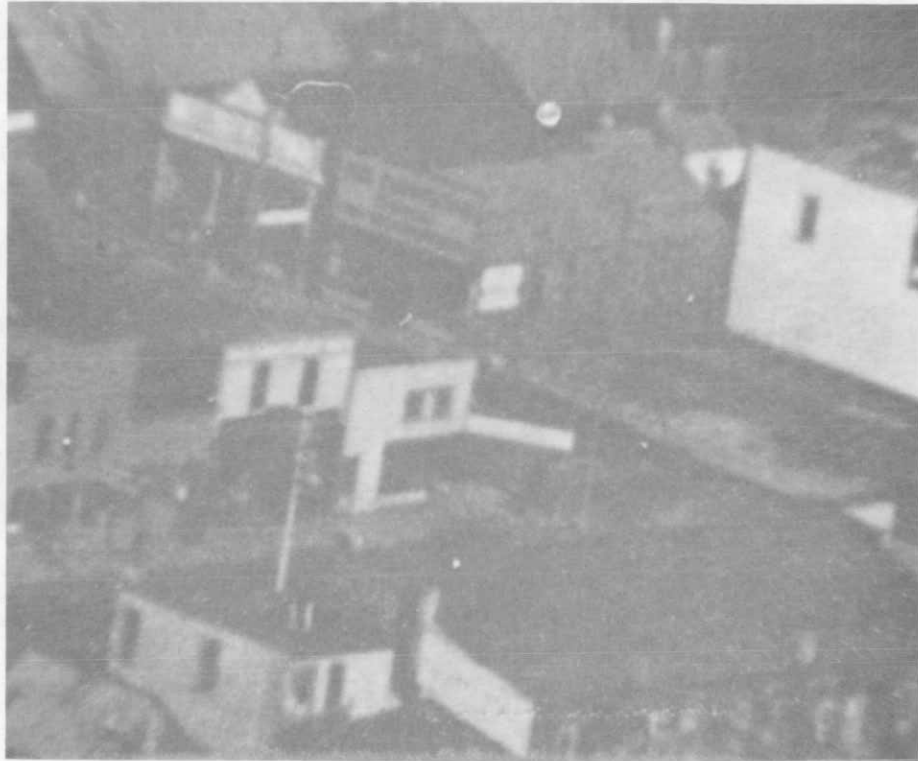
Photograph 6. Detail from a ca. 1900 photograph. East elevation with false front and display window in place.
