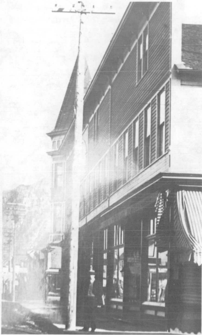
Photograph 5. Detail from a ca. 1910 photograph.
