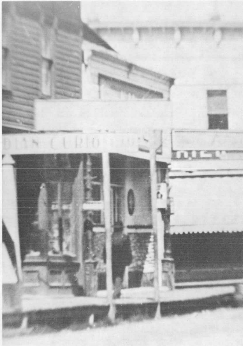
Photograph 14. Detail from a 1908 photograph. East elevation.
