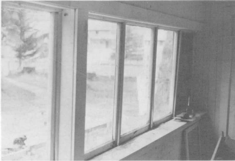
Photograph 48. South porch, south wall.
