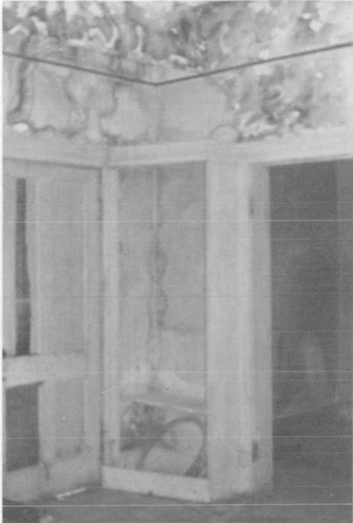
Photograph 21. Southwest corner, room 2.
