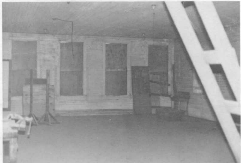
Photograph 46. June, 1981. West wall.
