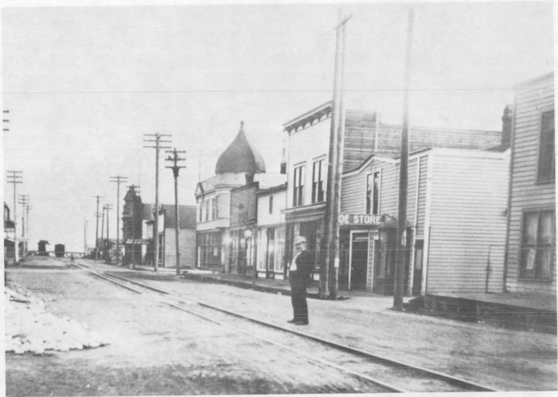
Photograph 6. From a ca. 1908 photograph. Note ramping of grade and boardwalk. North elevation of building was unpainted. Yukon Archives, Barley Collection.
