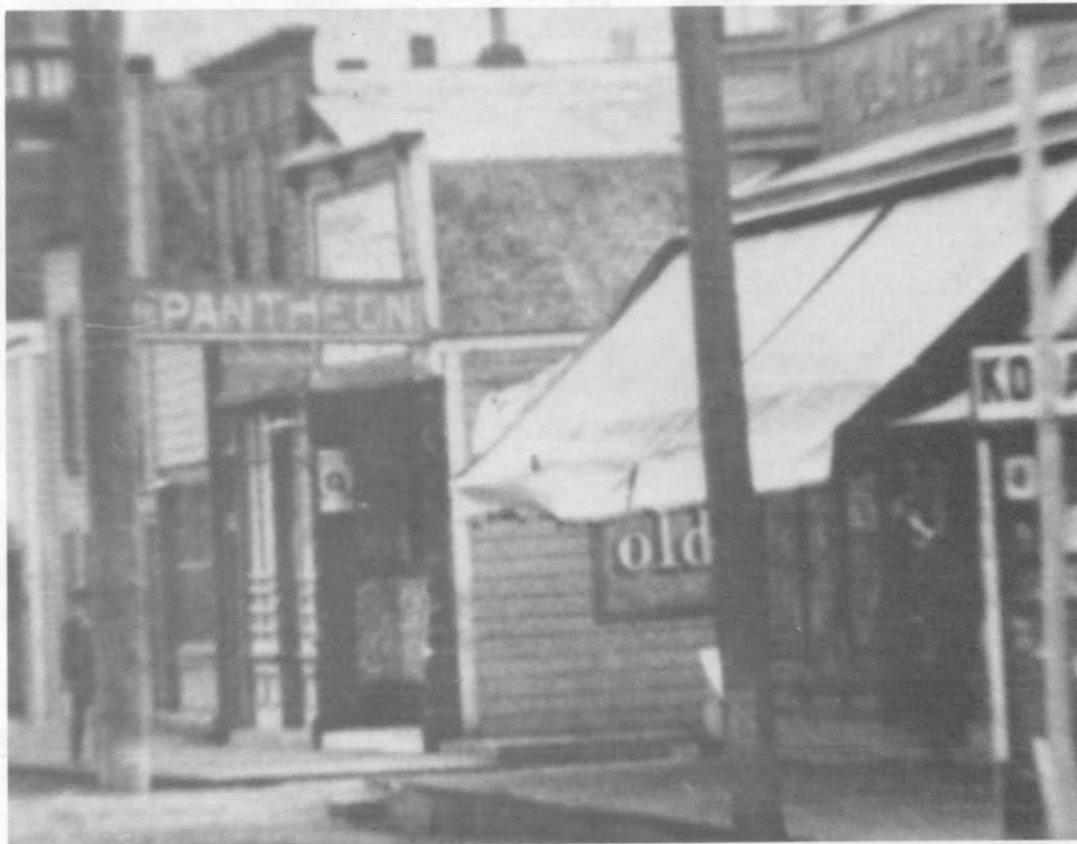
Photograph 16. Detail from a ca. 1914 photograph. View from northeast.
