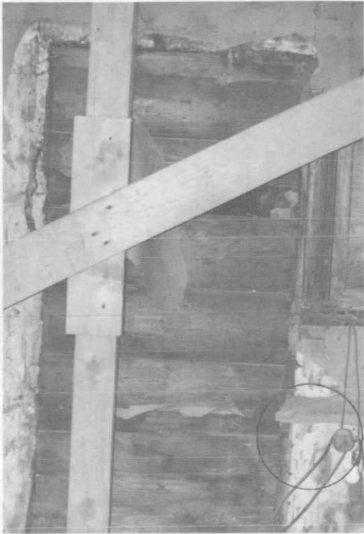
Photograph 12. South door (originally west) infill.
