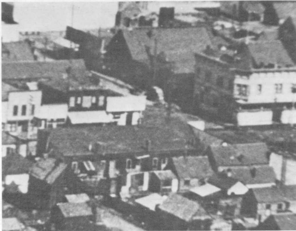
Photograph 12. Detail from a ca. 1905 photograph.
