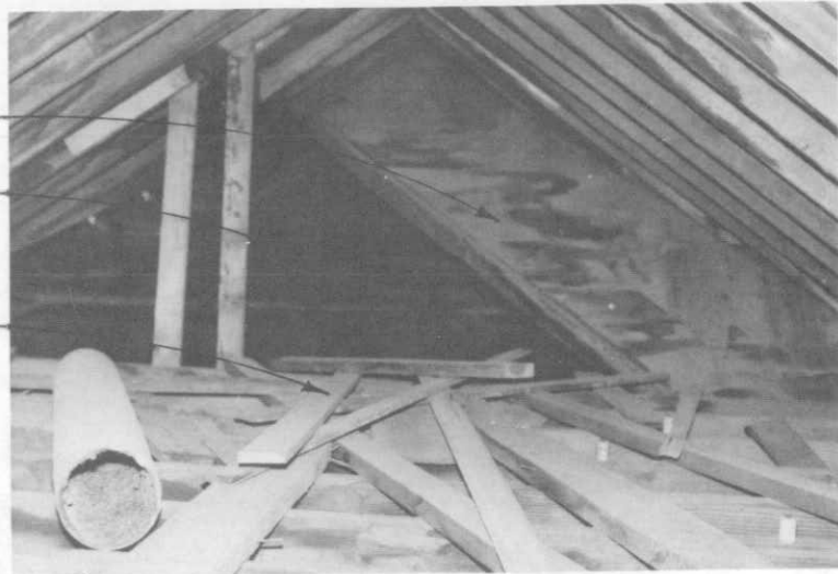
Photograph 24. West wing attic, east end.
