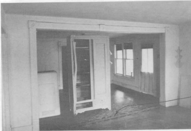
Photograph 33. East wall of parlor. N.P.S. photograph by R. Copeland, Oct. 1979.
