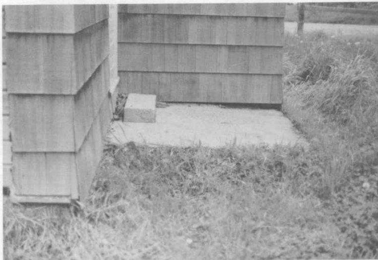
Photograph 12. Southeast porch detail.
