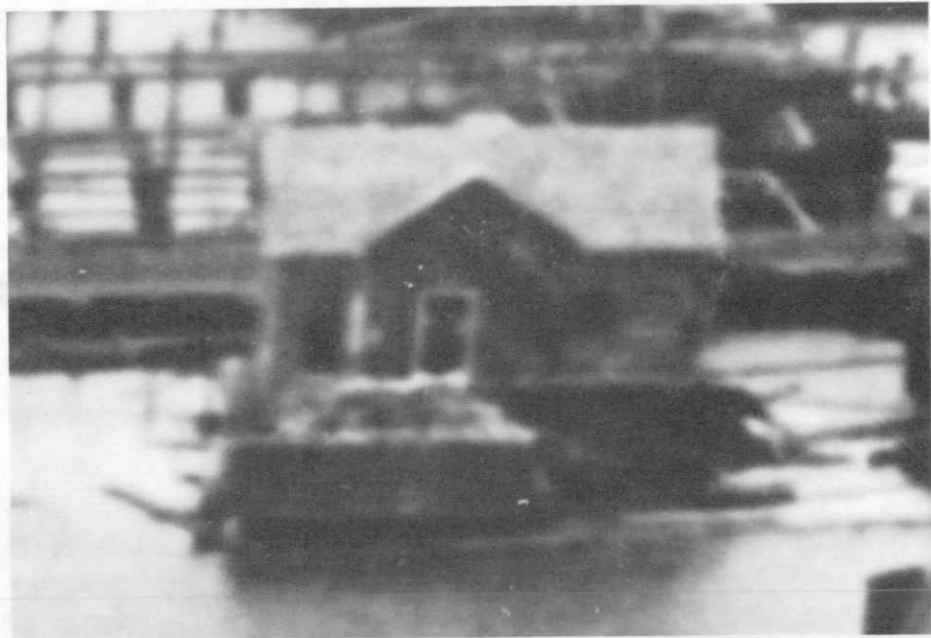
Photograph 2. Detail from ca. 1901 photograph. East elevation, now west.
