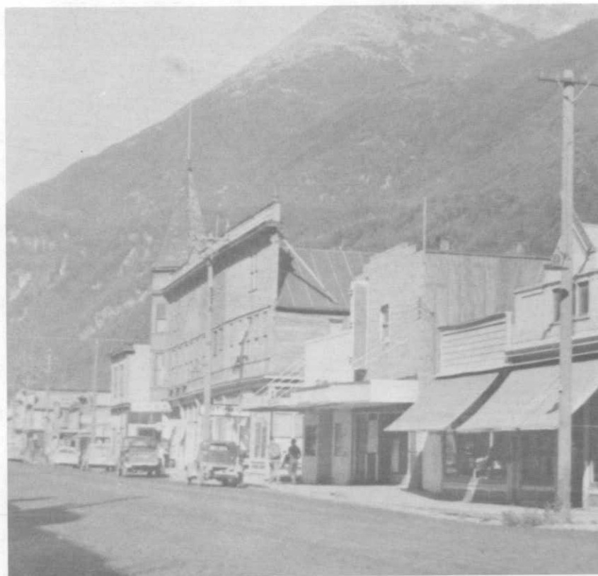
Photograph 11. From a ca. 1950 photograph. Note roll roofing. Dedman's Photo, Skagway.
