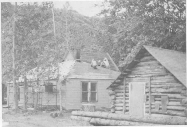
Photograph 27. View from northwest. July, 1981. New shingle roof installation in progress.
