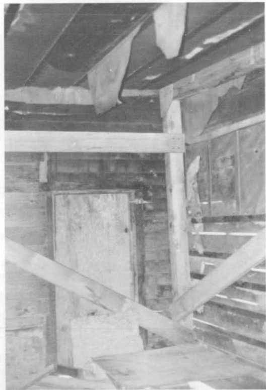
Photograph 15. Northwest corner, west room.
