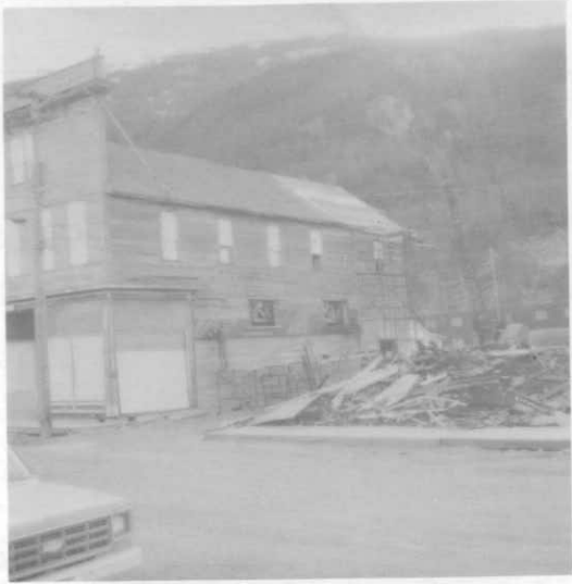
Photograph 20. April 1980. Exterior work in progress
