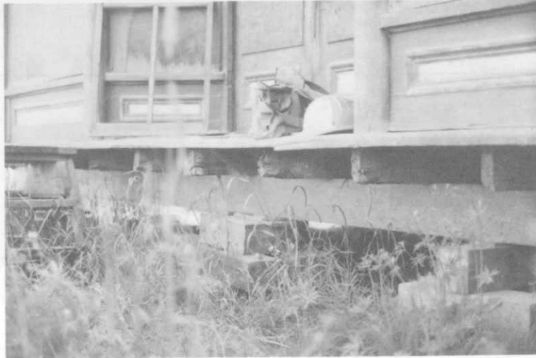
Photograph 24. Cribbing and floor framing detail.
