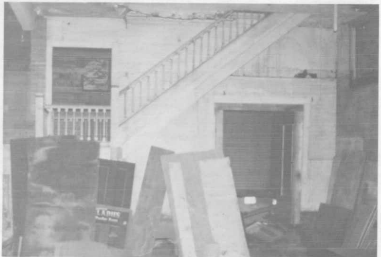
Photograph 37. 1981. East wall. Floor removed, foundation in place.
