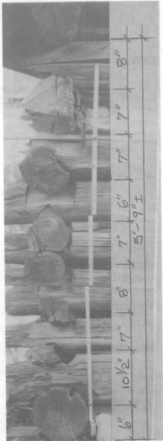
Photograph 69. Moore Cabin, southwest corner joint detail. April 1981.
