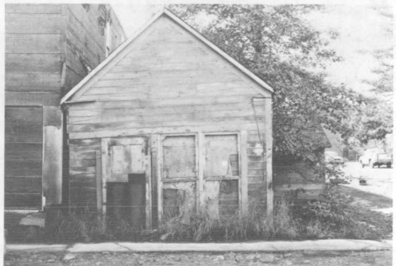
Photograph 4. Oct. 1977. North elevation on original site.
