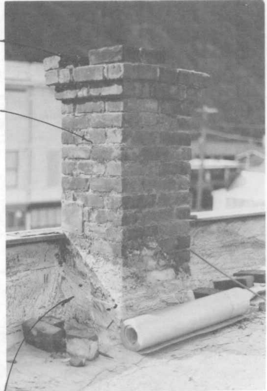
Photograph 37. Chimney detail, second story roof, ca. 1905 addition.
