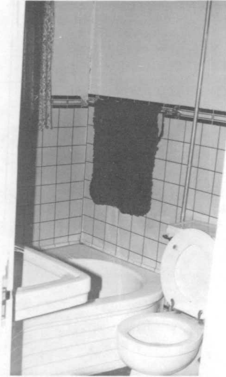
Photograph 28. West bathroom northeast corner.
