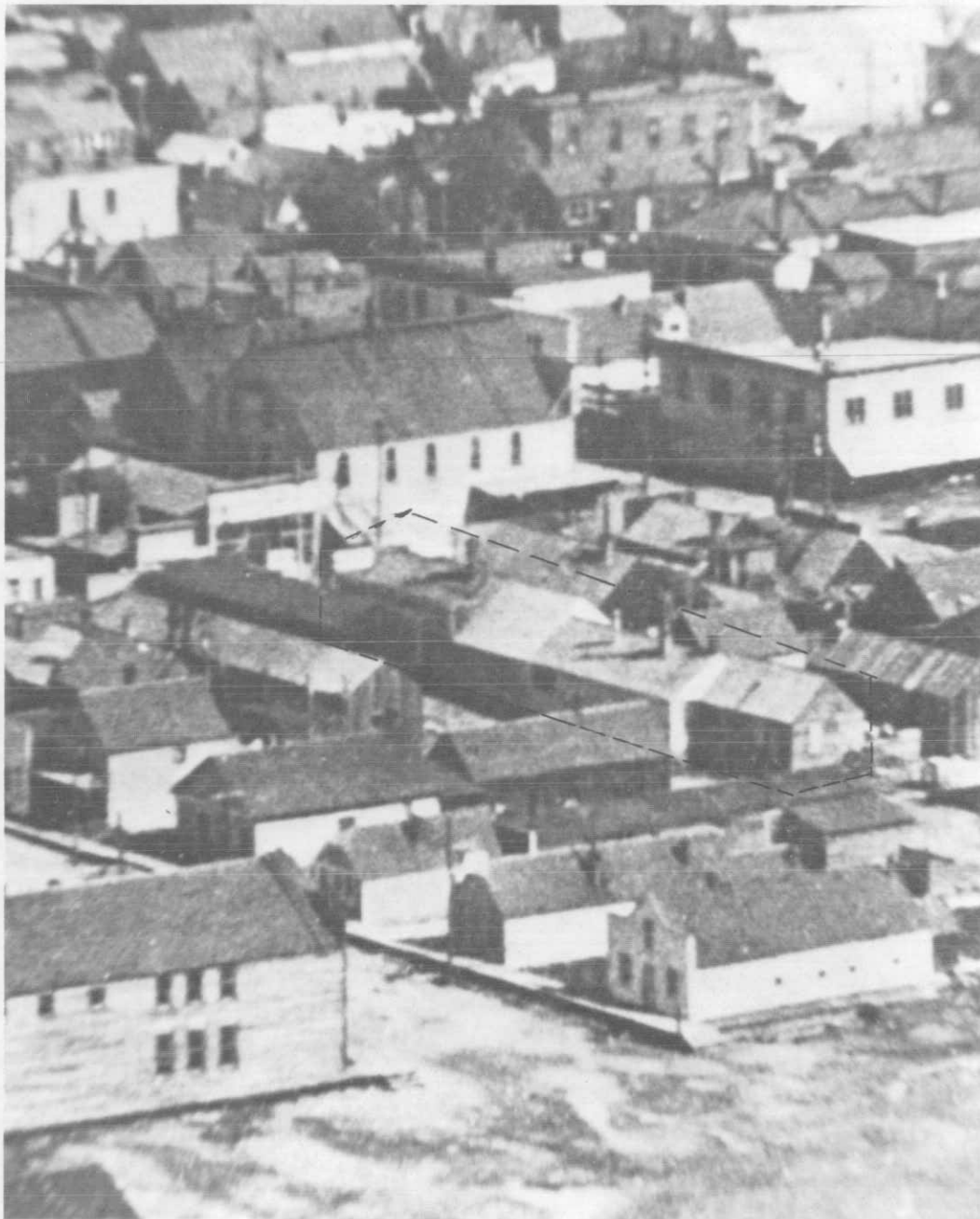
Photograph 11. Detail from a ca. 1943 photograph.
