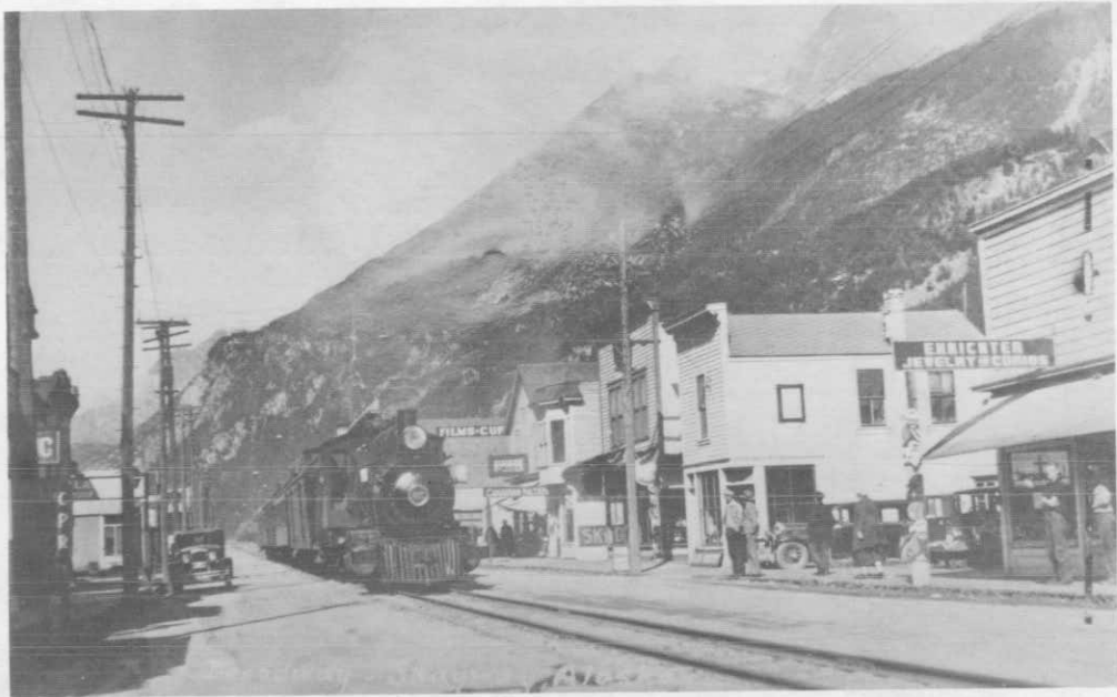
Photograph 8. From a ca. 1926-30 photograph; after 1926 relocation of building. Dedman's Photo, Skagway.
