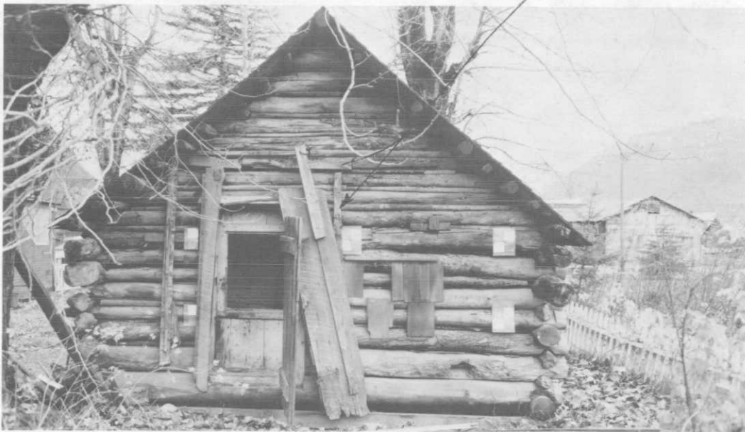
Photograph 67. Moore Cabin, north elevation.
