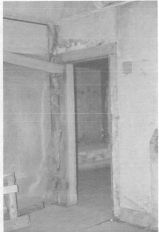
Photograph 17. Northeast corner, room 2.
