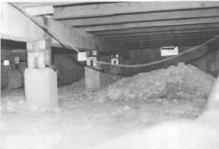
Photograph 18. Foundation and first floor framing.
