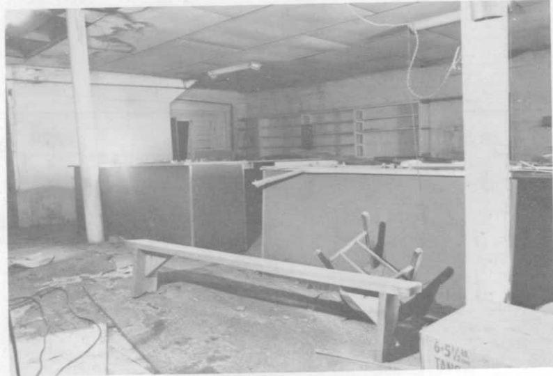
Photograph 32. 1978. As found conditions.
