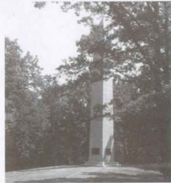
FIGURE 12. U. S. Monument, constructed in 1909.
