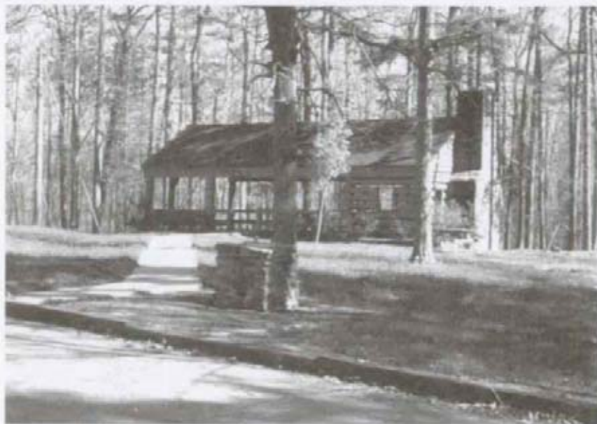
FIGURE 15. CCC Shelter in Kings Mountain State Park.
