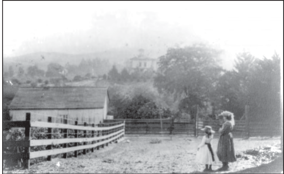
Figure 2.7: This photograph was taken next to the barn in the late 1880s and looks east toward the Muir House. (A1-16, Ref: 1890cP19. Same as Figure 2.7 in Volume 1 of the CLR).
