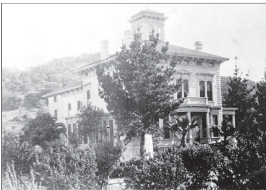
Figure 2.12: This photograph of the Muir House, looking southwest toward the wooded north slope of Mt. Wanda, dates from c.1890. (A1-34, Ref: 1890cP18a. Same as Figure 2.9 in Volume 1 of the CLR).
