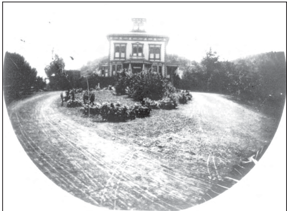
Figure 2.4: View from c.1886, looking south, of the carriage drive-loop and the front entrance of the Muir House. (A1-93, Ref: 1886cP1. Same as Figure 2.8 in Volume 1 of the CLR).
