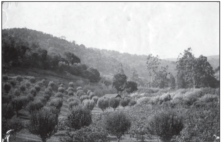
Figure 2.2: View looking southwest from the west side of the knoll toward Mt. Wanda in the late 1890s. (JOMU, no file #. Same as Figure 3.5 in Volume 1 of the CLR).
