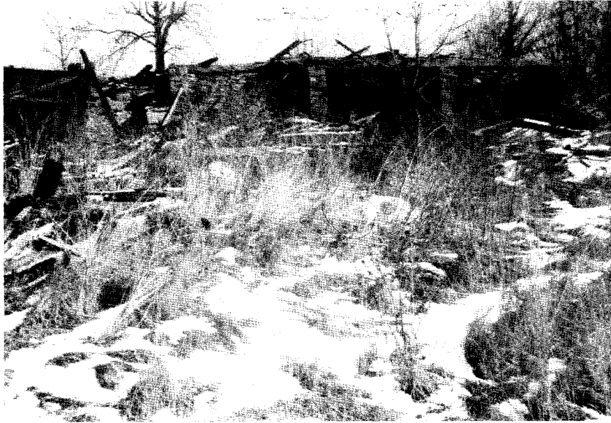
58. South foundation wall of carriage shed. February 1984. NPS photograph.
