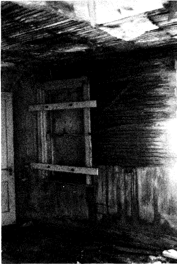
19. South wall of room 005, Unger House. October 1984. NPS photograph.
