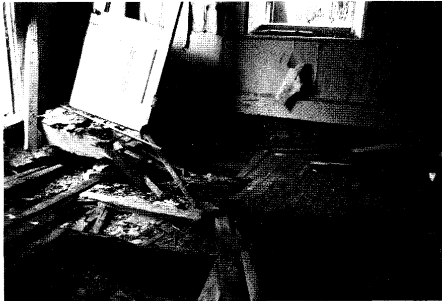
20. Floor of room 005, Unger House. October, 1984. NPS photograph.
