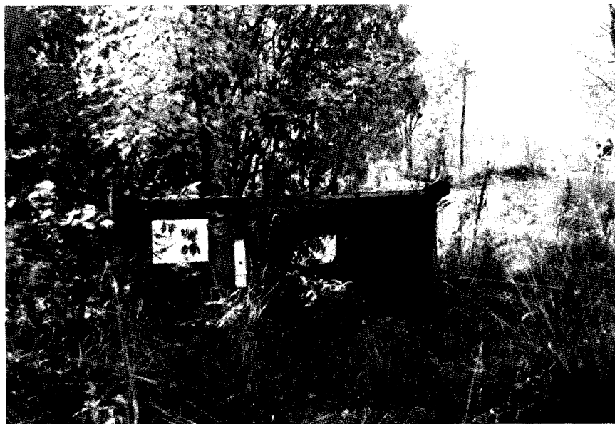
61. The well house, looking south. October 1984. NPS photograph.
