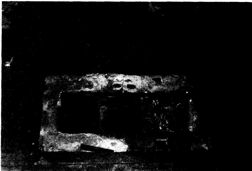
46. Floor opening at chimney, room 201, Unger House. October 1984. NPS photograph.
