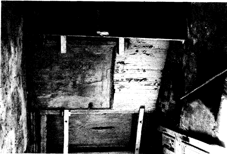
23. South wall of room 004, Unger House. October 1984. NPS photograph.
