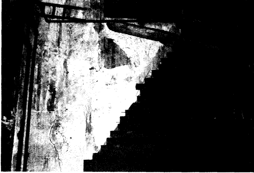
26. East wall of room 001, Unger House. October 1984. NPS photograph.
