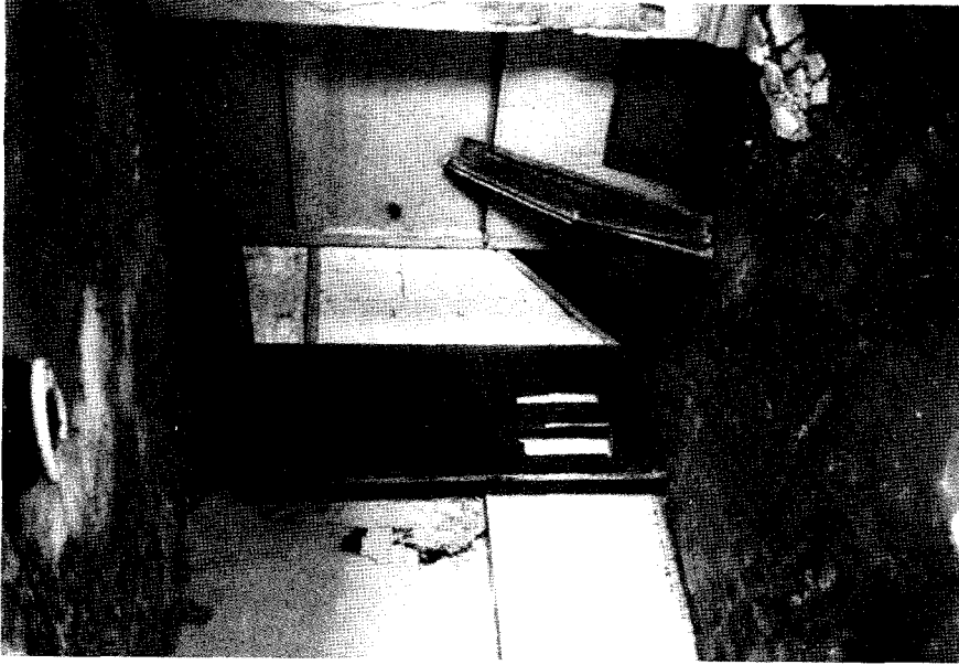
24. Northwest corner of room 004, Unger House. October 1984. NPS photograph.
