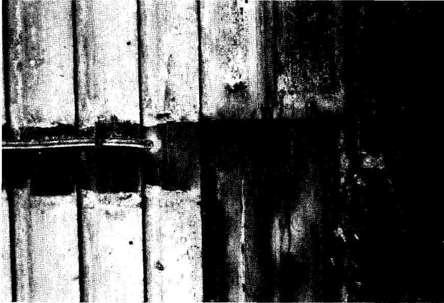
12. Mortise for porch beam, north facade, Unger House. October 1984. NPS photograph.
