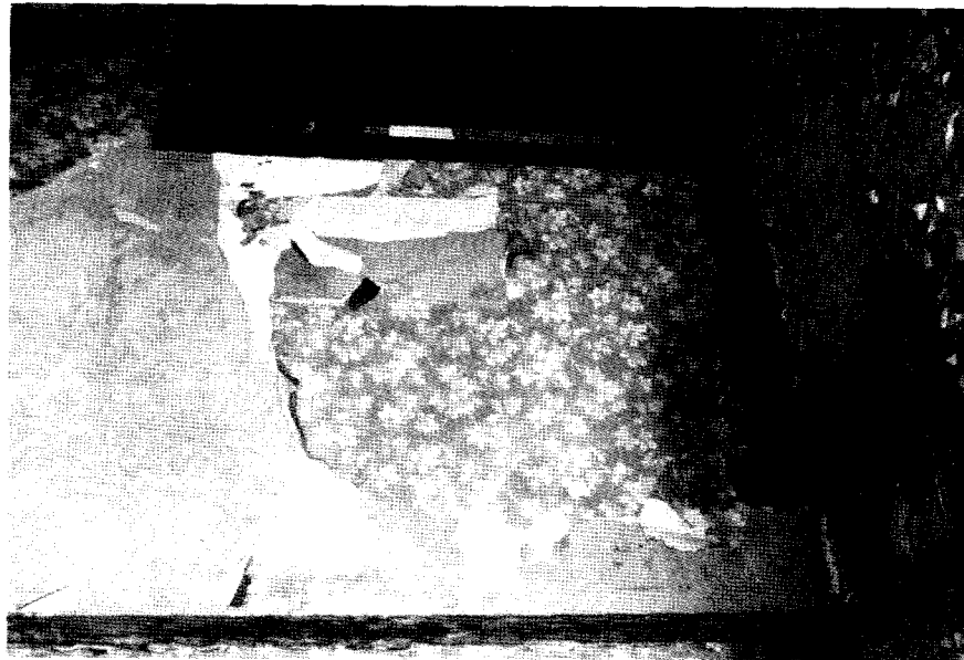
38. Fireplace at north wall of room 104, Unger House. November 1984. NPS photograph.
