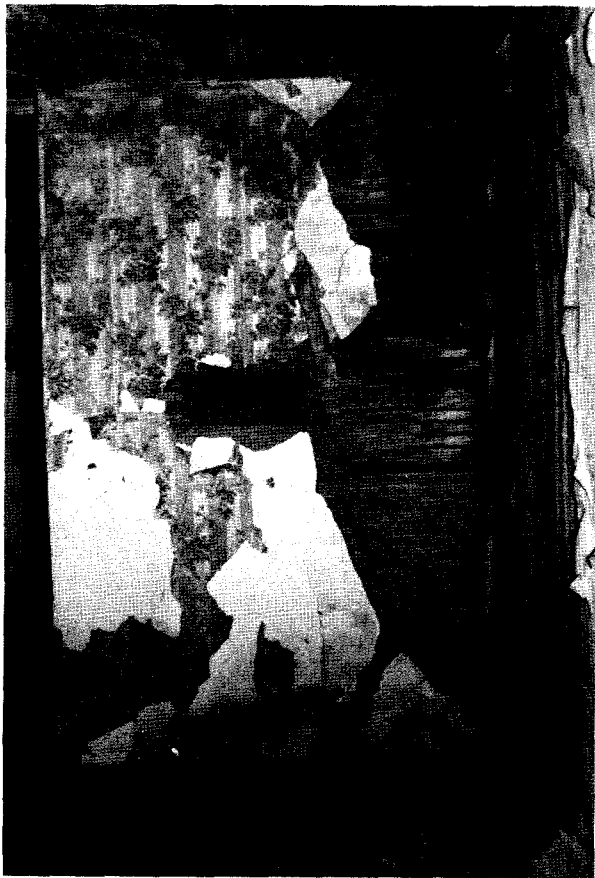
45. South corner of east wall of room 201, Unger House. October 1984.
