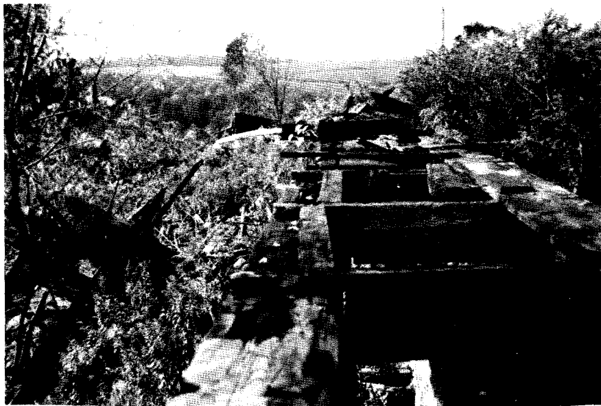
59. Floor framing of carriage shed at south foundation wall, looking west. October 1984. NPS photograph.
