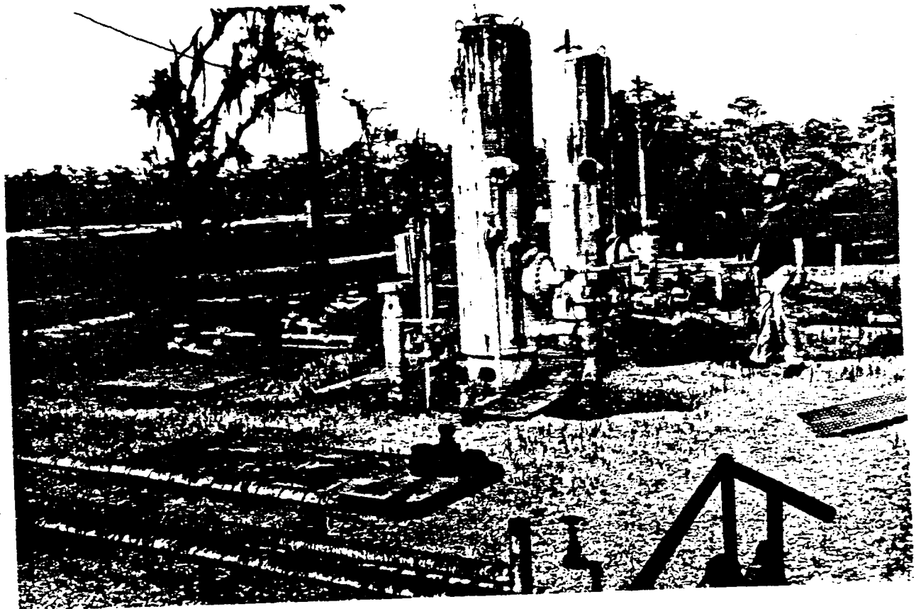
Barataria Oil Field, showing separator tanks on concrete pads and flow lines. 4/86.
