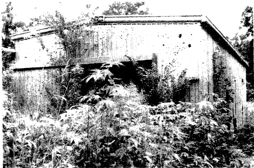
Photo 19. Illegal Pumphouse, Barataria District.
