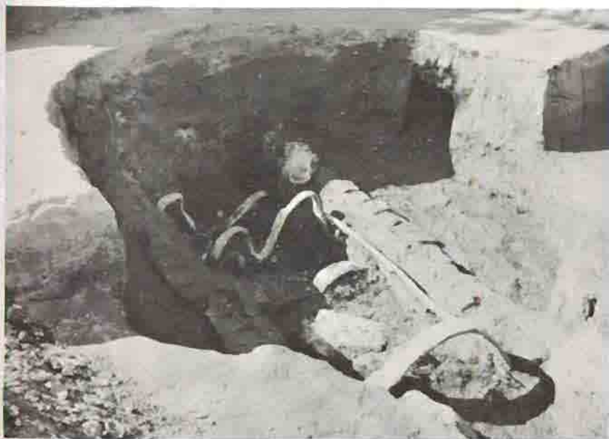
A 17TH-CENTURY LIME KILN EXCAVATED AT JAMESTOWN. IN IT OYSTER SHELLS FROM THE JAMES RIVER WERE BURNED FOR MAKING LIME. THE IRON HOOPS WHICH SUPPORTED THE ARCHED TOP OF THE KILN BUCKLED FROM THE INTENSE HEAT.
