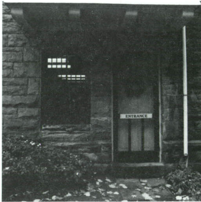
CP-55, Entrance to the gift shop and house tour. The high stoop is a barrier to wheelchairs.
