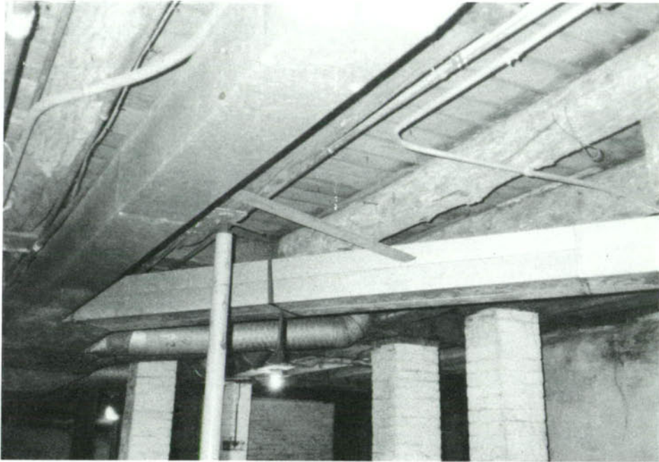
SP-23, First-floor framing, room 001.
