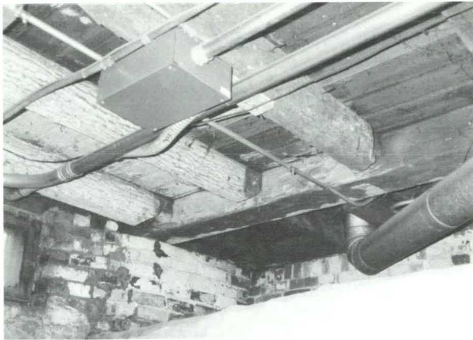
SP-2, Northeast foundation corner, room 103.
