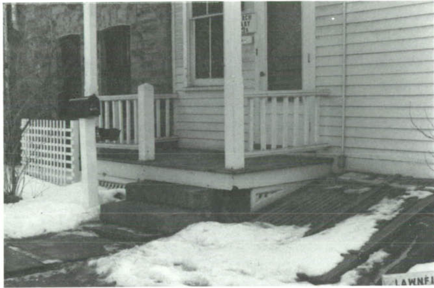
CP-29, North porch deck and cellar door.
