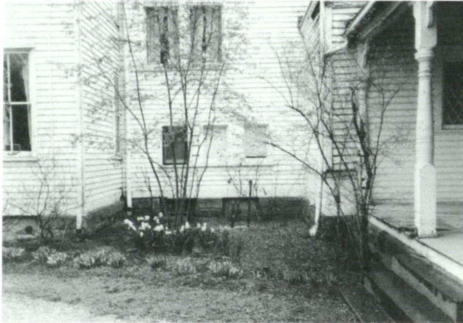
SP-7, Exterior view of main stair wall.
