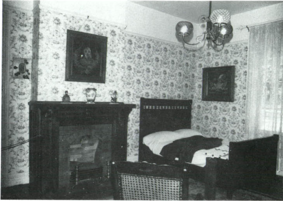
CP-67, James A. Garfield bedroom, room 103, looking northwest.
