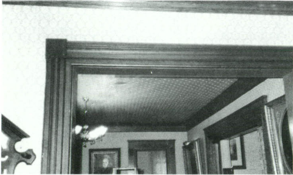
SP-27, Parlor ceiling at the beam.
