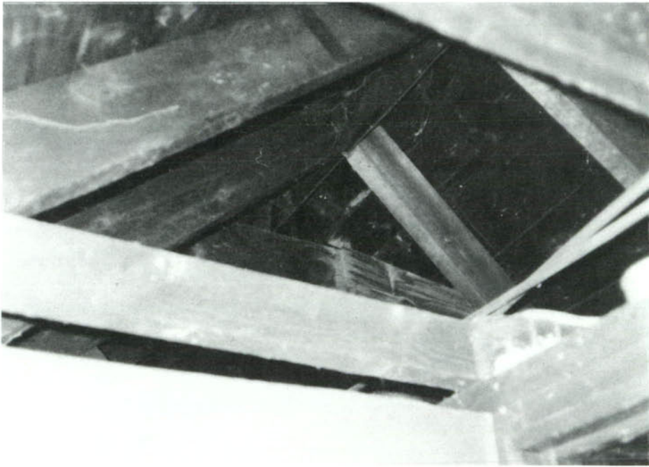
SP-40, Room 308, roof framing, southeast view.
