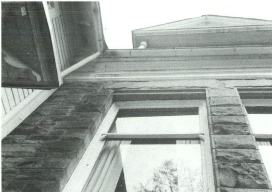
SP-10, Library window, exterior view.
