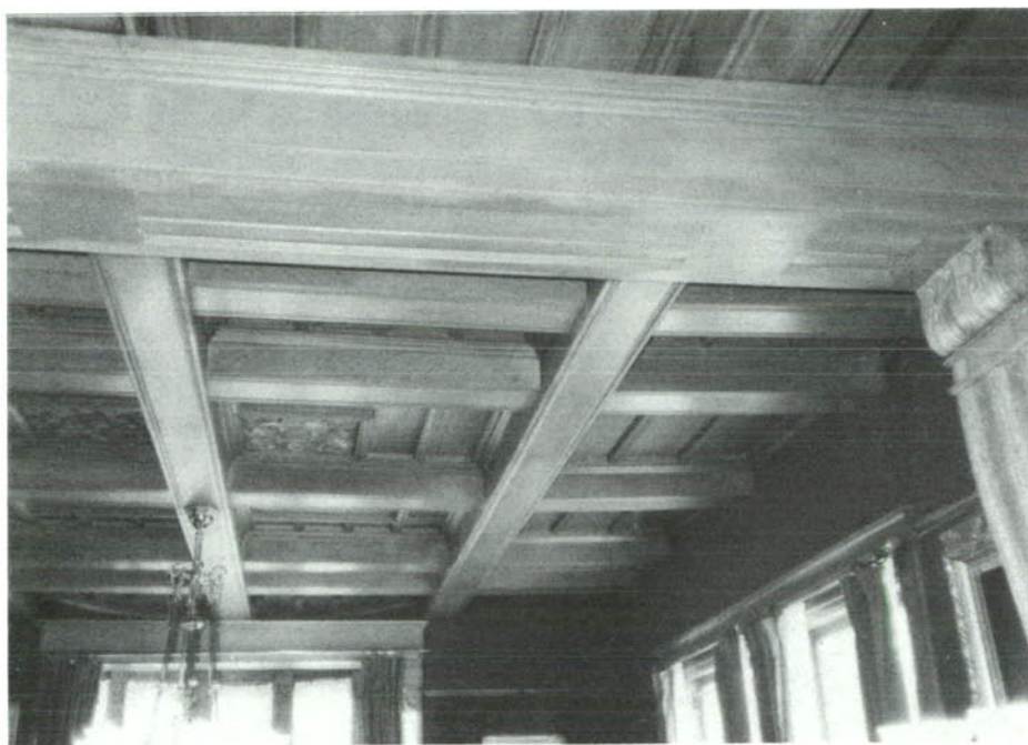
SP-30, Library ceiling, southeast view.
