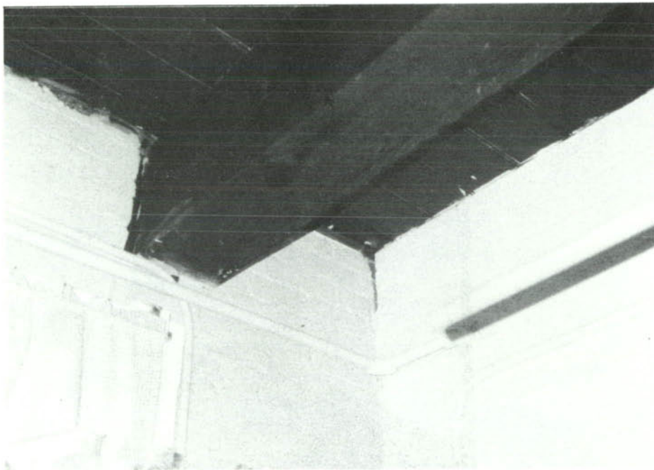
SP-26, Library floor framing.
