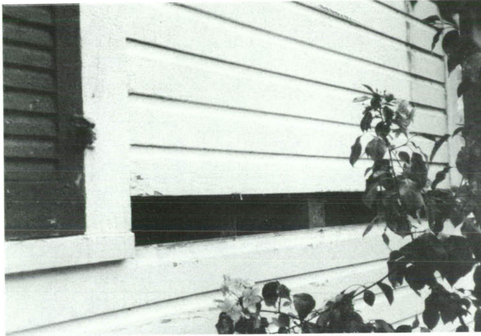
SP-5, Balloon framing, room 103.
