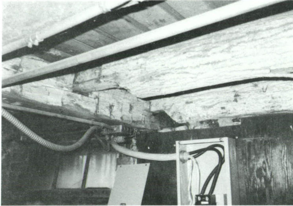
SP-19, First-floor framing beneath room 103.
