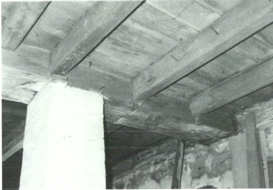
SP-21, First-floor framing, room 001.
