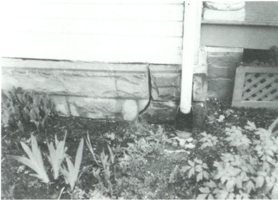
SP-4, Limestone veneer, west elevation, room 103.
