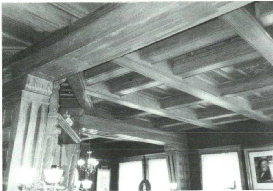
SP-29, Library ceiling, northeast view.
