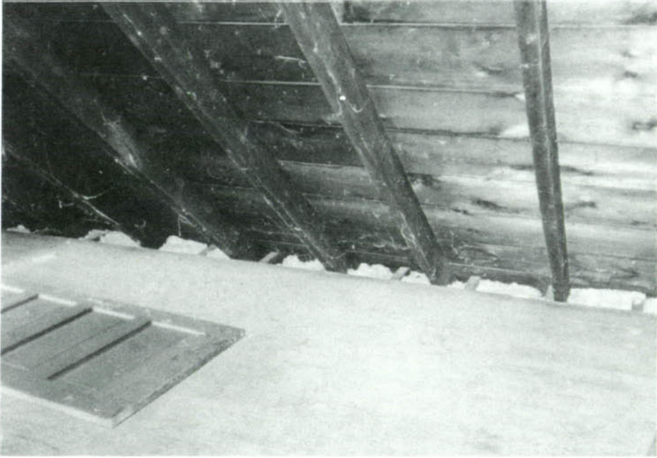
SP-39, Room 308, roof framing, north view.
