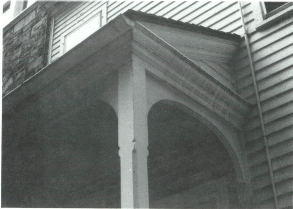
CP-28, Detail of the north porch roof.
