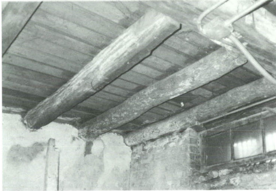
SP-1, Southeast foundation corner, room 103.
