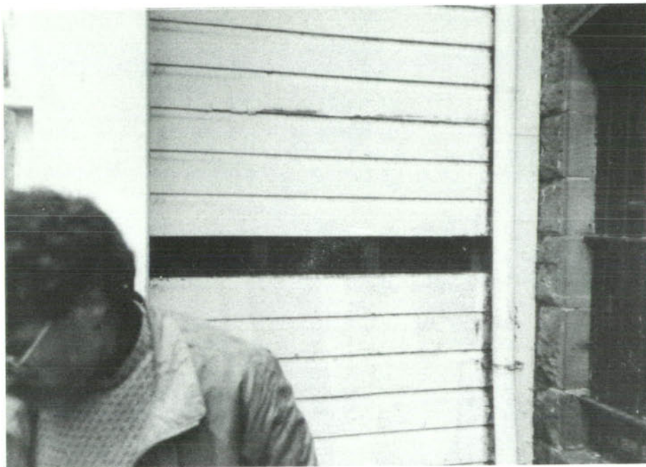
SP-6, Balloon framing, room 111.
