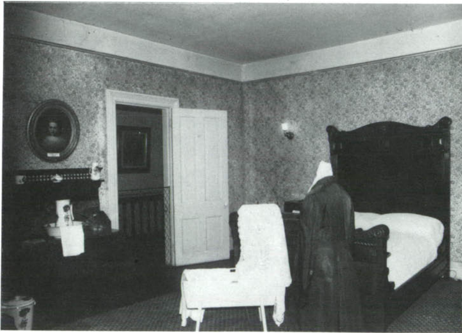
CP-96, Lucretia Garfield bedroom, room 208, looking northwest.
