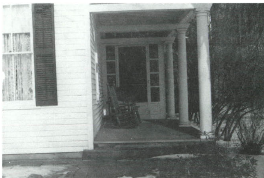
CP-24, 1904 east porch with enclosed entrance area to dining room.
