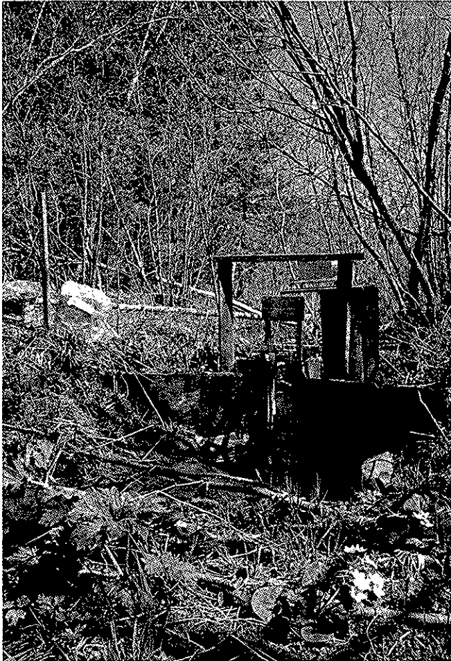
Figure 3. Stream gauging station (W1) at the mouth of the first-order sub-catchment Wallace 1 in the Wallace Lake watershed, Isle Royale National Park, Michigan.
