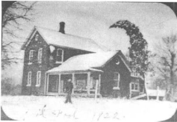
Figure II-29: The northeastern portion of the farmhouse. (H2-0010)
