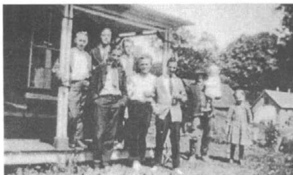
Figure II-19: Circa 1914-1915 photo of "Montreal Bank Employees" In the background there is a structure that looks like a corncrib near the chicken coop.
