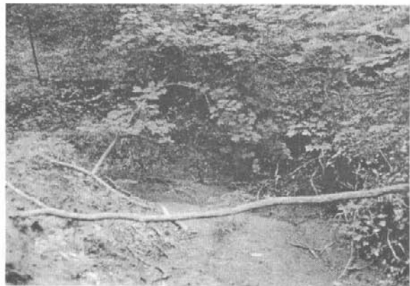
Figure III-31: Erosion west of Sugar camp, 8/11/98.
