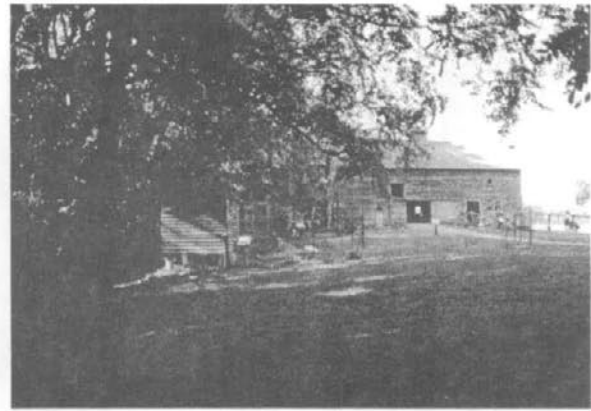
Figure III-14: Barn and chicken coop, south elevations, 8/11/98.
