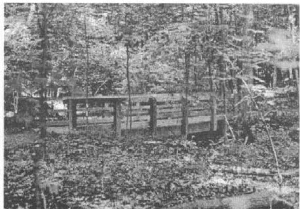
Figure III-32: Bridge over washout area west of Sugar camp, 8/11/98.
