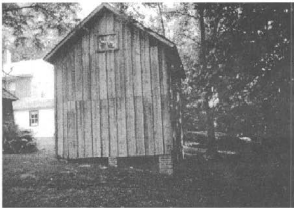
Figure III-16: Granary, north and west elevations, 8/11/98.
