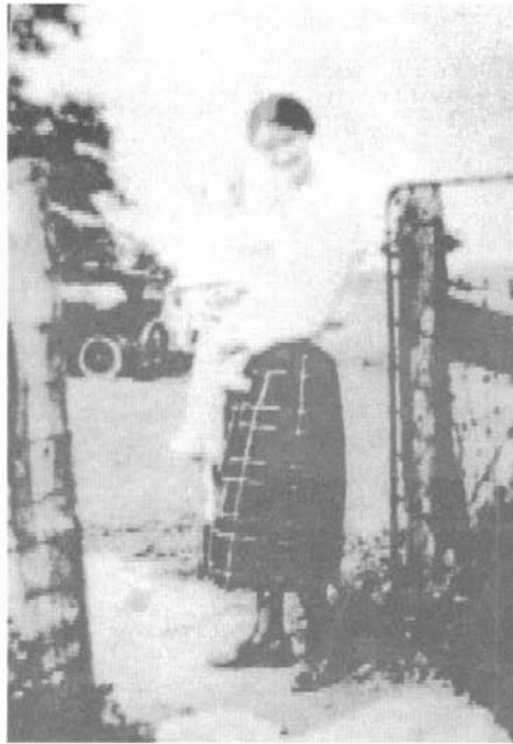
Figure II-36: Gate and sidewalk north of the farmhouse, circa 1920s.
