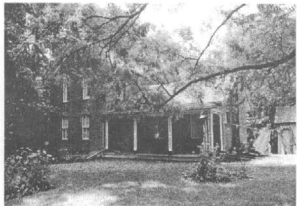
Figure III-9: Farmhouse, east elevation, 8/11/98.
