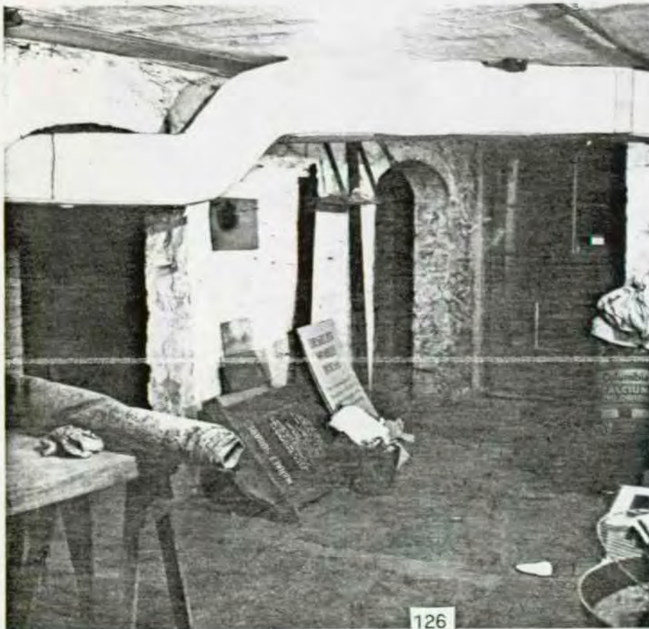
ILLUSTRATION 43 Photographed by NPS. 1772 Section Cellar-Room 02. Brick pier (1884) with wedges to support joists.
