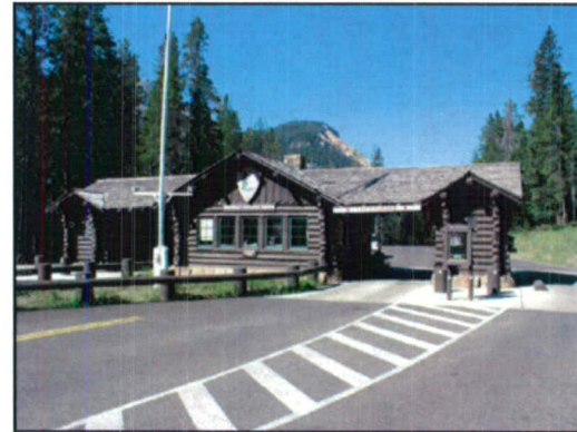
Northeast Entrance Station - Yellowstone NP
