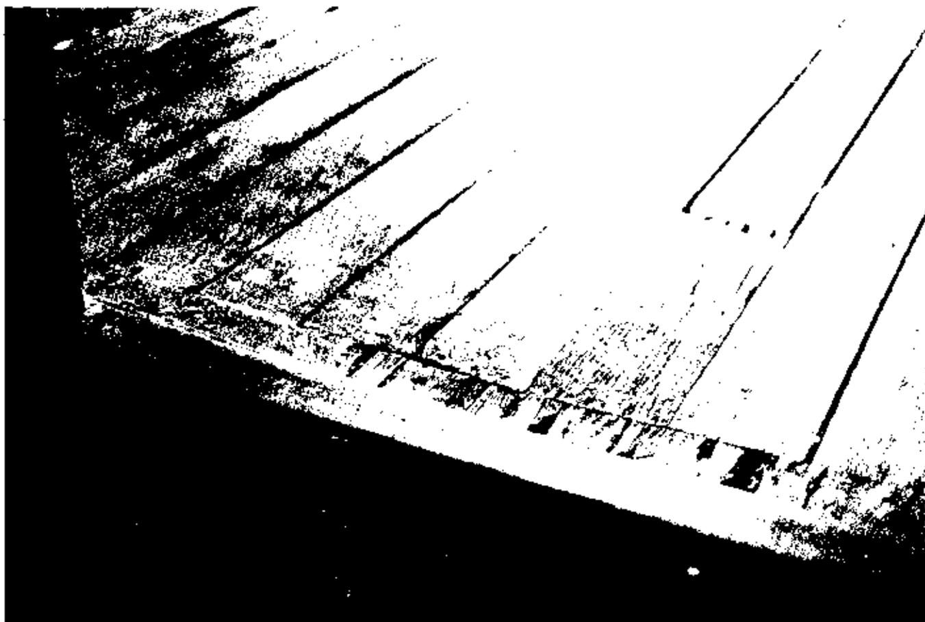
**Illustration 90.** The Grange: Second-Floor Southwest Room, Floorboard Evidence of Original Main Stairwell (1977).
