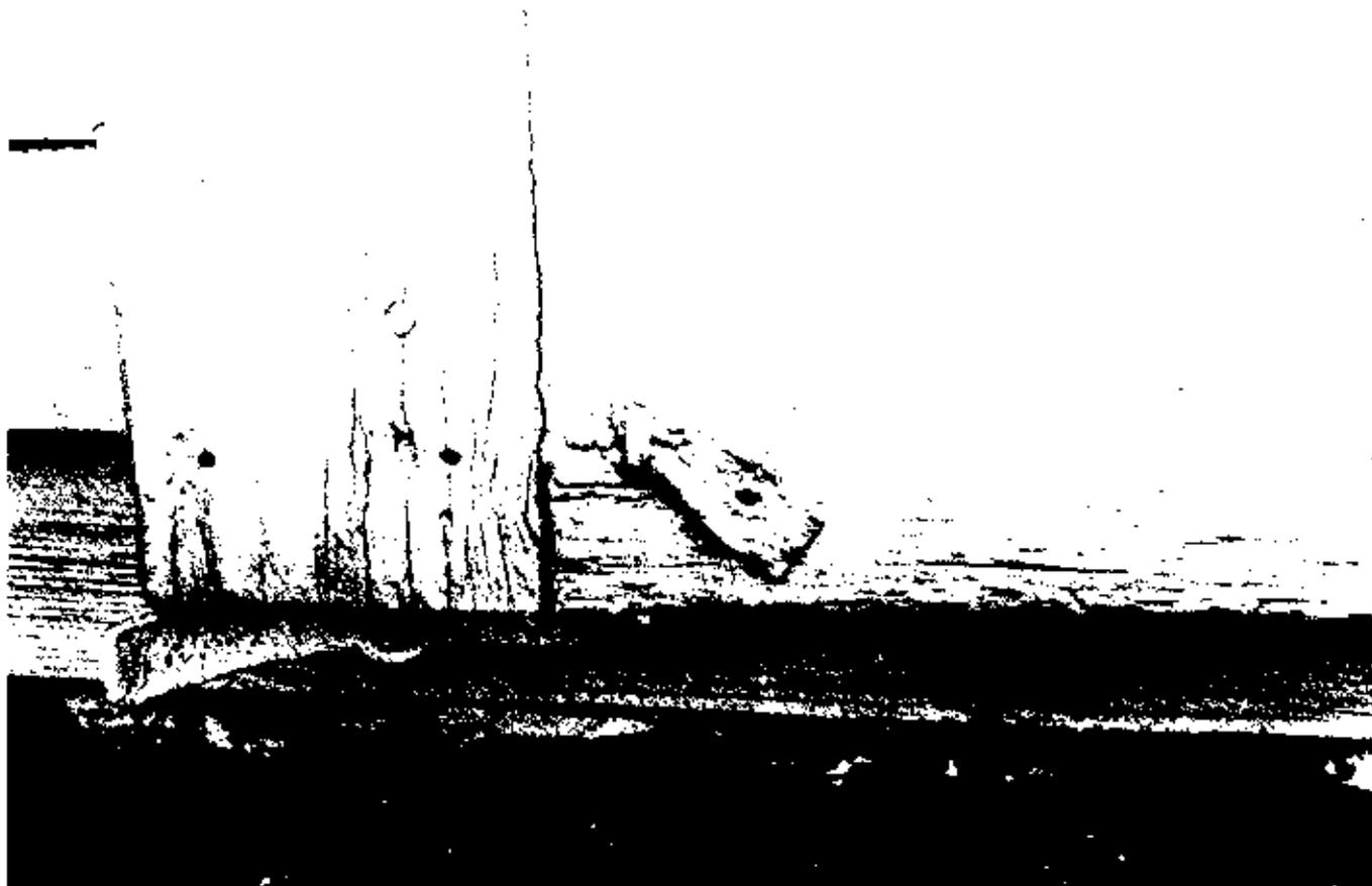
Illustration 128. The Grange: Exterior Shutters, Tab and Pin Fastener (1977).
