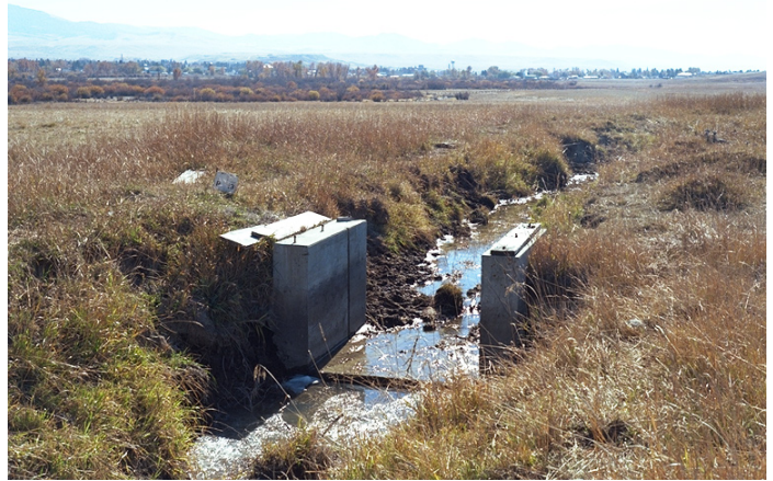
Concrete Headgate (JMA, Oct. 2002)
