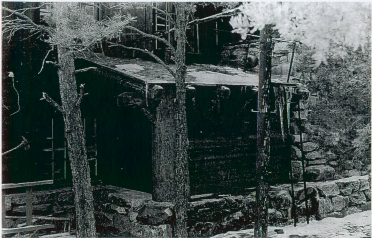
Figure 15: Completed vault at east elevation of Headquarters' Building, February 1936. Note stone foundation and emergency exit ladder.
