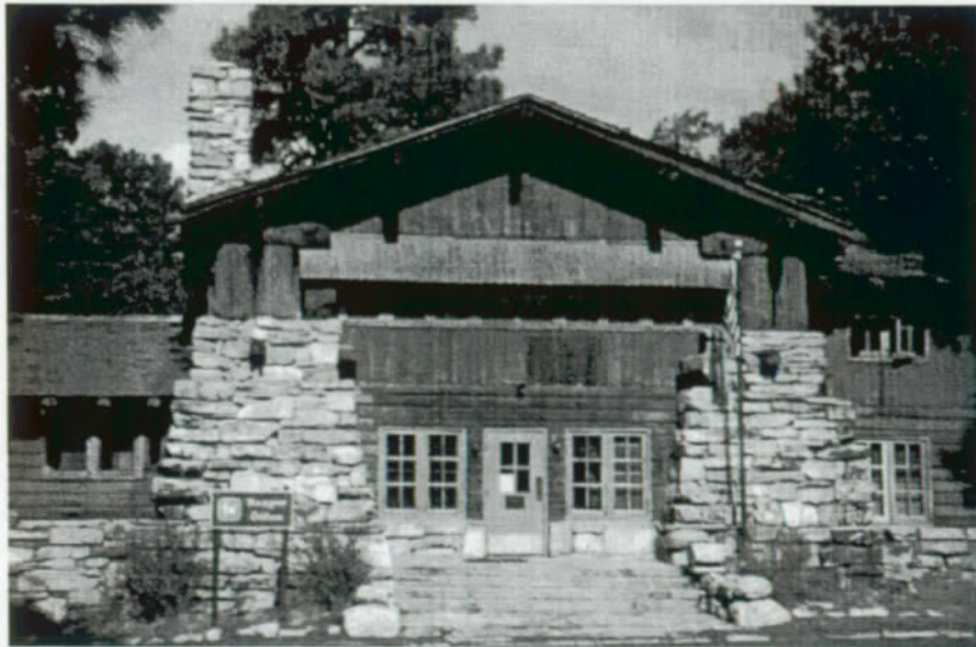
Figure 20: Principal facade, May, 2000. Dark patch above the main door and window on right indicates the previous position of non-historic building sign.
