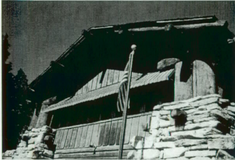
Figure 17: Metal awning at west elevation.
