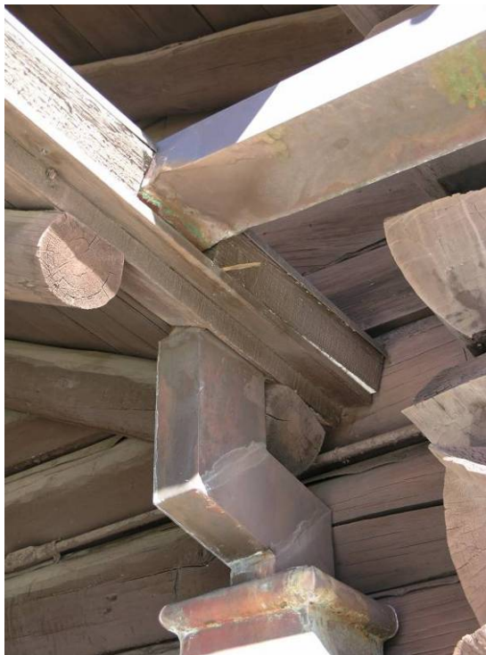
E-38 Same location as above, downspout/gutter detail. October 3, 2007. Photograph by Chamberlin Architects.
