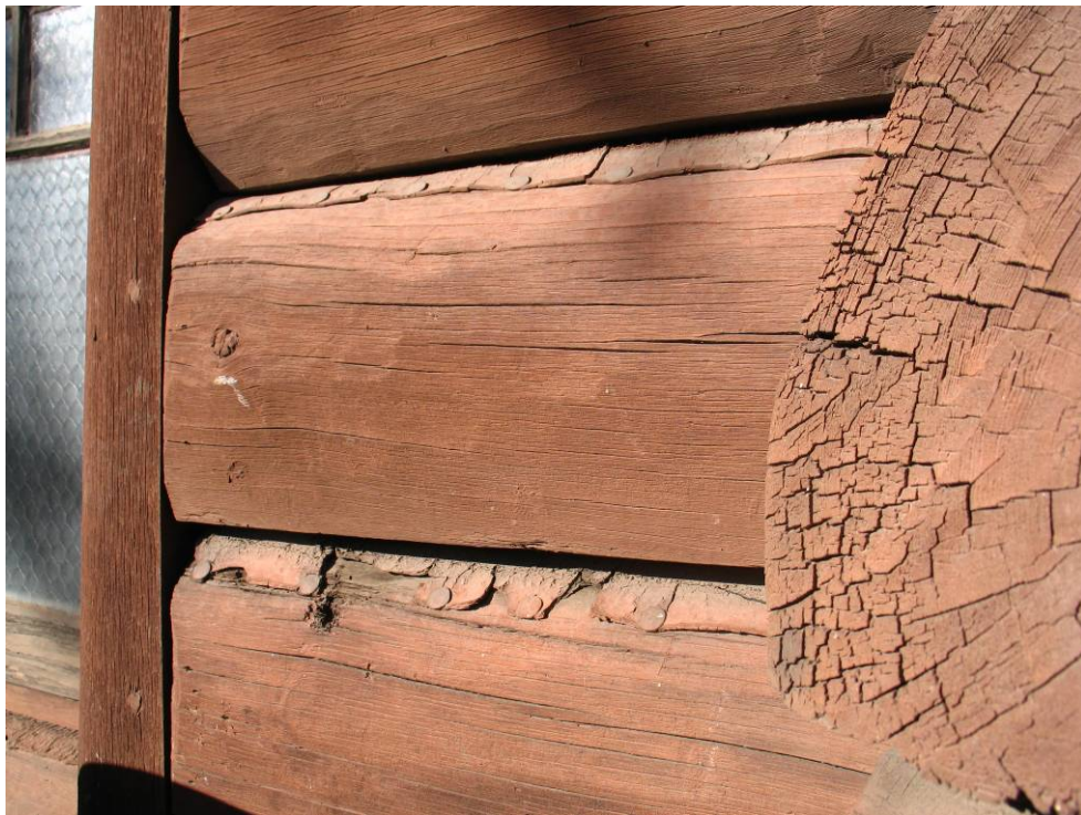
E-80 View of “Rubberoid” flashing. Note deterioration of exposed surface. October 3, 2007. Photograph by Chamberlin Architects.
