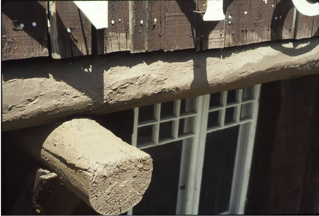
H-81 Grand Canyon Depot close up of log repair on south side brackets. Date 1984-1986. Scanned from building files.
