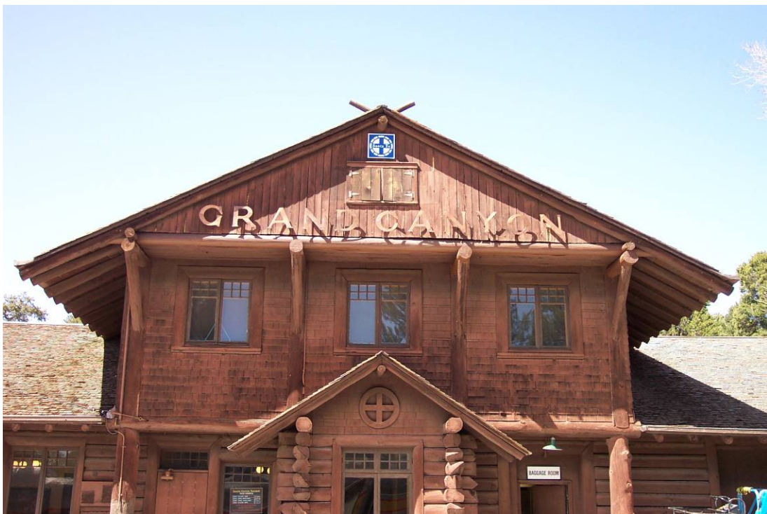
H-152 Grand Canyon Depot during rehabilitation. South elevation of completed gable beam and brackets. Date 2005. From building files. Photo by Craig Struble.
