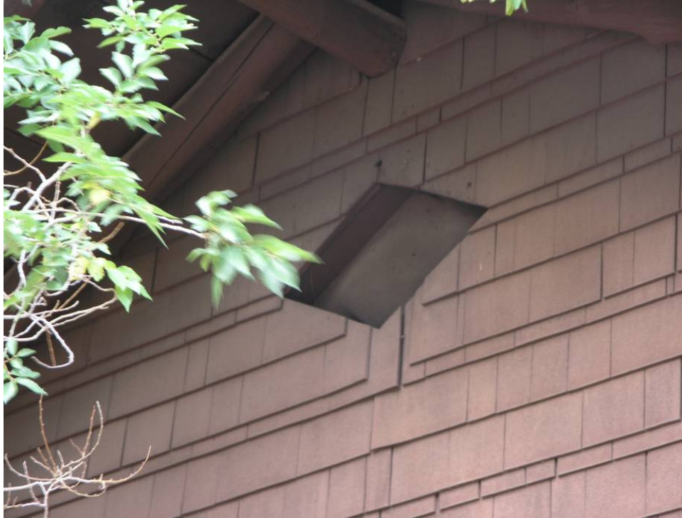
E-65 East façade, gable vent. Note that the vent has been closed off. A suitable screen and louver should be installed. October 3, 2007. Photograph by Chamberlin Architects.
