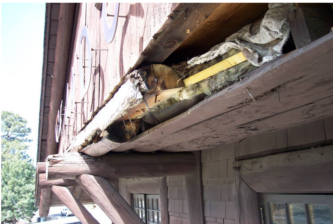
H-150 Grand Canyon Depot during rehabilitation. Deterioration of south gable beam and brackets. Date 2005. From building files. Photo by Craig Struble.
