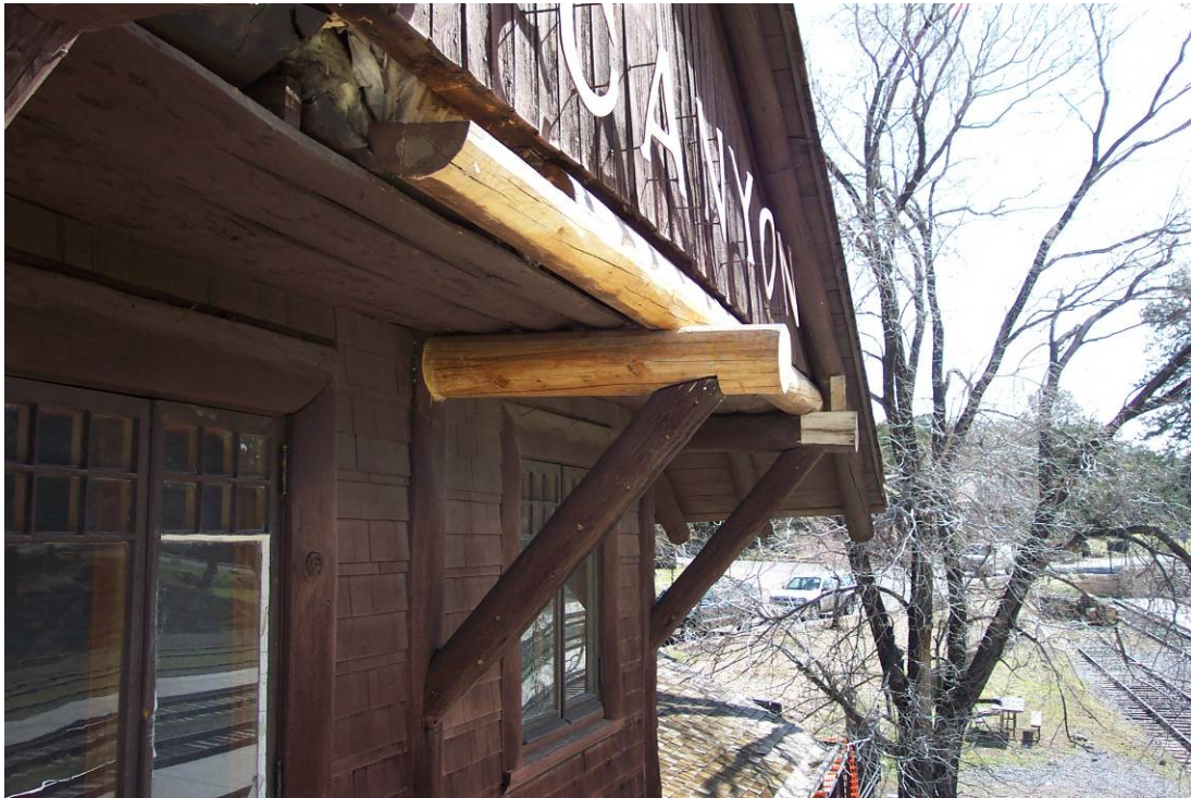
H-151 Grand Canyon Depot during rehabilitation. Replaced south gable beam and brackets. Date 2005. From building files. Photo by Craig Struble.
