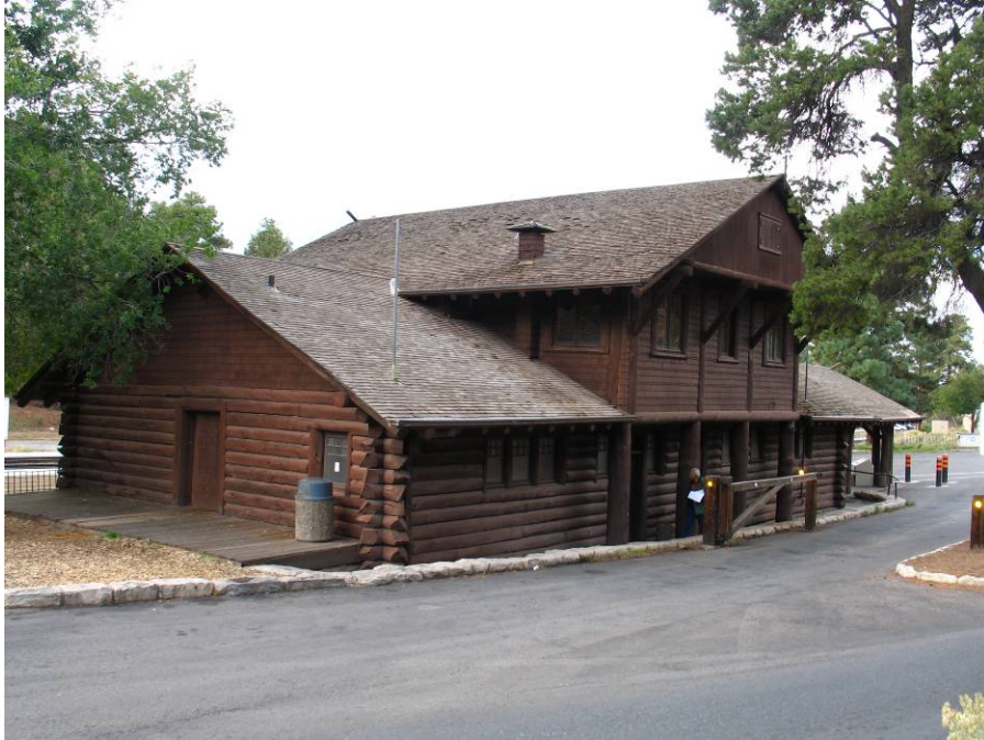
E-5 View from northeast. Note that the barge rafter extensions are missing from the east gable. October 3, 2007. Photograph by Martin/Martin.
