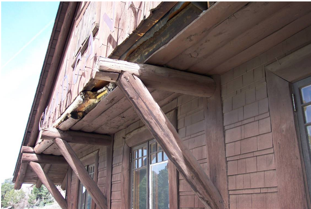
H-149 Grand Canyon Depot during rehabilitation. Deterioration of south gable beam and brackets. Date 2005. From building files. Photo by Craig Struble.
