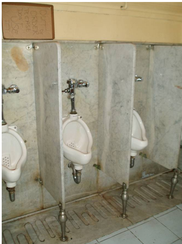
M-3: Men's Restroom 106 Urinals. Note marble floor, wainscot and partitions. Photograph by MKK.
