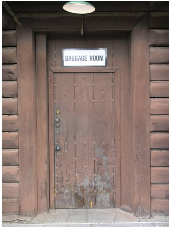
E-103 Door 103A. Note traffic wear on door. October 3, 2007. Photograph by Chamberlin Architects.
