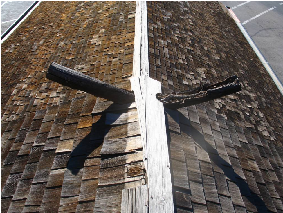
E-83 Close up of false barge rafter extensions at west roof. Note deterioration. October 3, 2007. Photograph by Martin/Martin.
