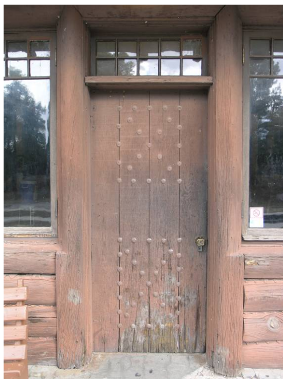
E-110 Door 101A. Note deterioration of door. October 3, 2007. Photograph by Chamberlin Architects.
