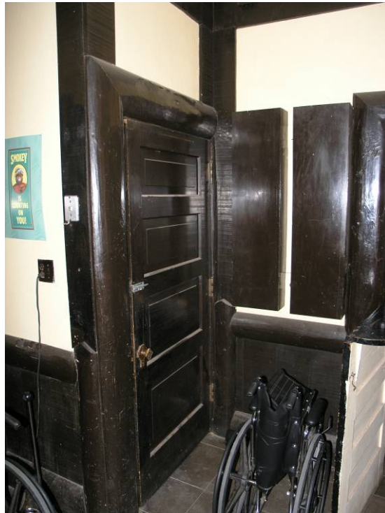
I-121 Door 107B (left) and partial door 102E. Note wood cabinets mounted on wall between the doors. Conflict with Door 107B. October 3, 2007. Photograph by Chamberlin Architects.
