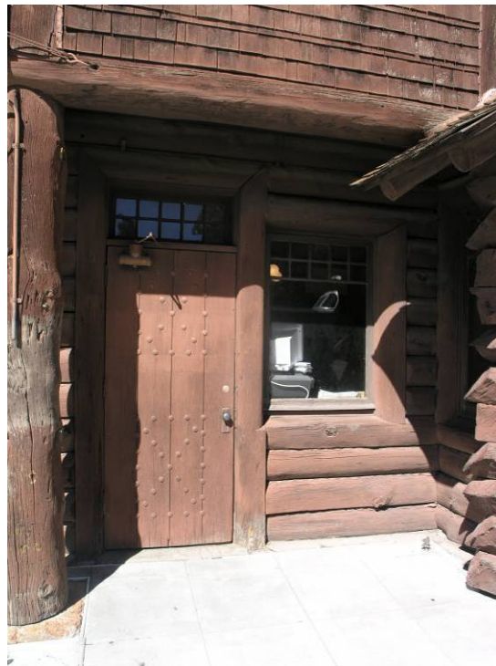
E-32 South façade, door and windows to office. Door 101A and Window 116. Note deterioration of lower door casing. October 3, 2007. Photograph by Chamberlin Architects.
