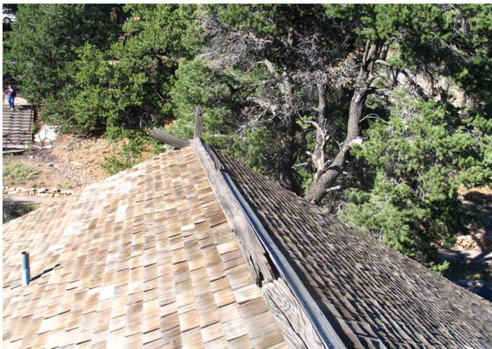
E-87 Main upper roof looking north. Note deterioration of ridge board and missing barge rafter extension. Note vertical board at gable end, possibly for radio antennae. October 3, 2007. Photograph by Martin/Martin.
