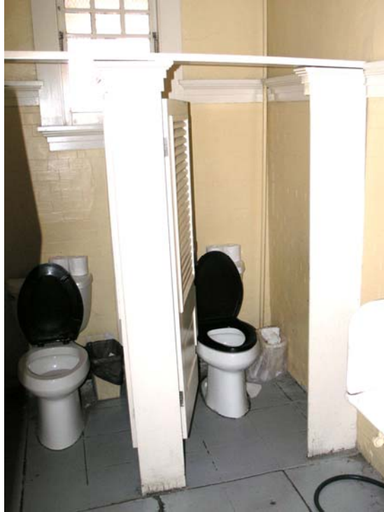
M-13: Womens's Restroom 110 Water Closet. Note that the women's fixtures appear to be more modern compared to men's [Photograph M-2. Photograph by Chamberlin Architects.
