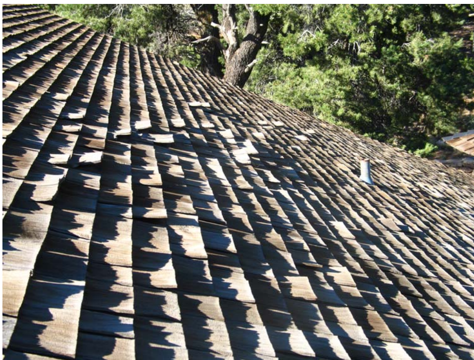
E-88 Main roof, east side, looking north. Note cupping of roof shingles. October 3, 2007. Photograph by Martin/Martin.
