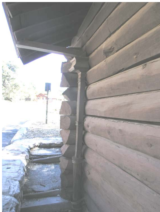
E-63 North façade, looking at northeast corner of building. Note the large gapes between some of the logs. October 3, 2007. Photograph by Chamberlin Architects.
