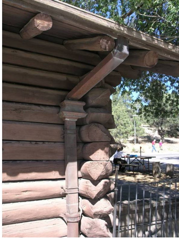
E-25 South façade, southeast corner. Note reconstructed copper downspouts. October 3, 2007. Photograph by Chamberlin Architects.
