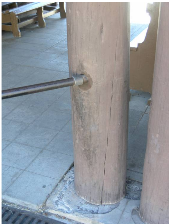
E-51 Base of column on east side of covered waiting area. Note handrail attached to column, installed sometime after 1935. October 3, 2007. Photograph by Chamberlin Architects.
