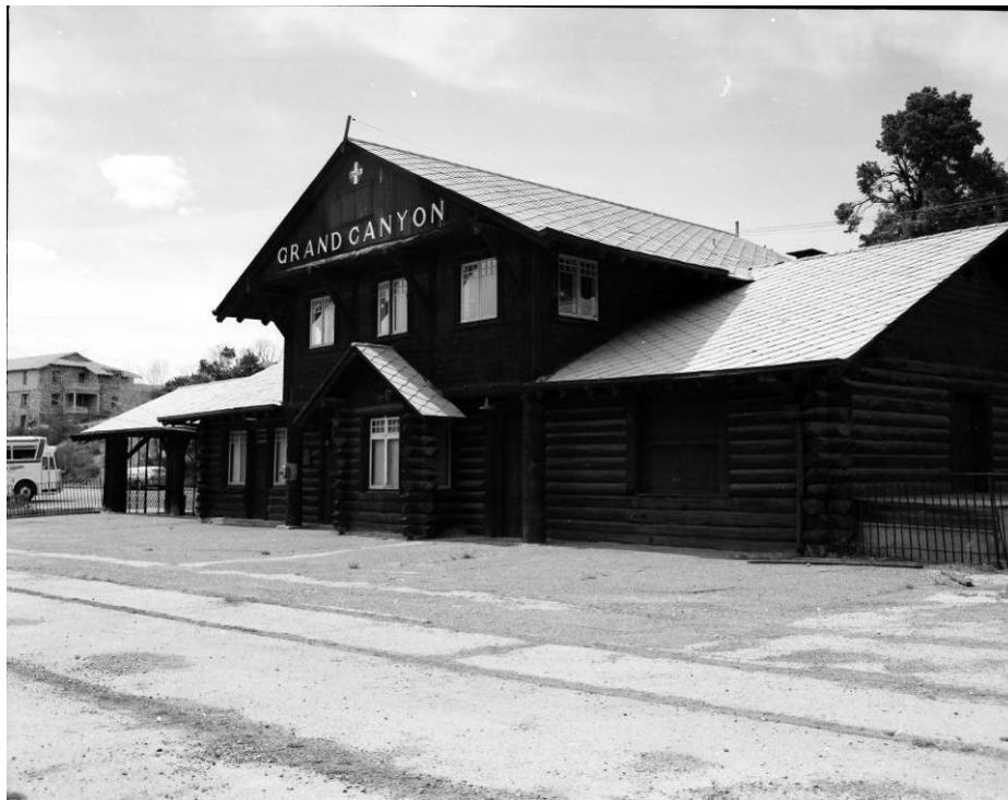
H-56 Santa Fe Railroad Depot, southeast exposure. Note that asbestos-cement shingles are still in place. Date 1976. NPS photo. NPS Catalog # GRCA 10737
