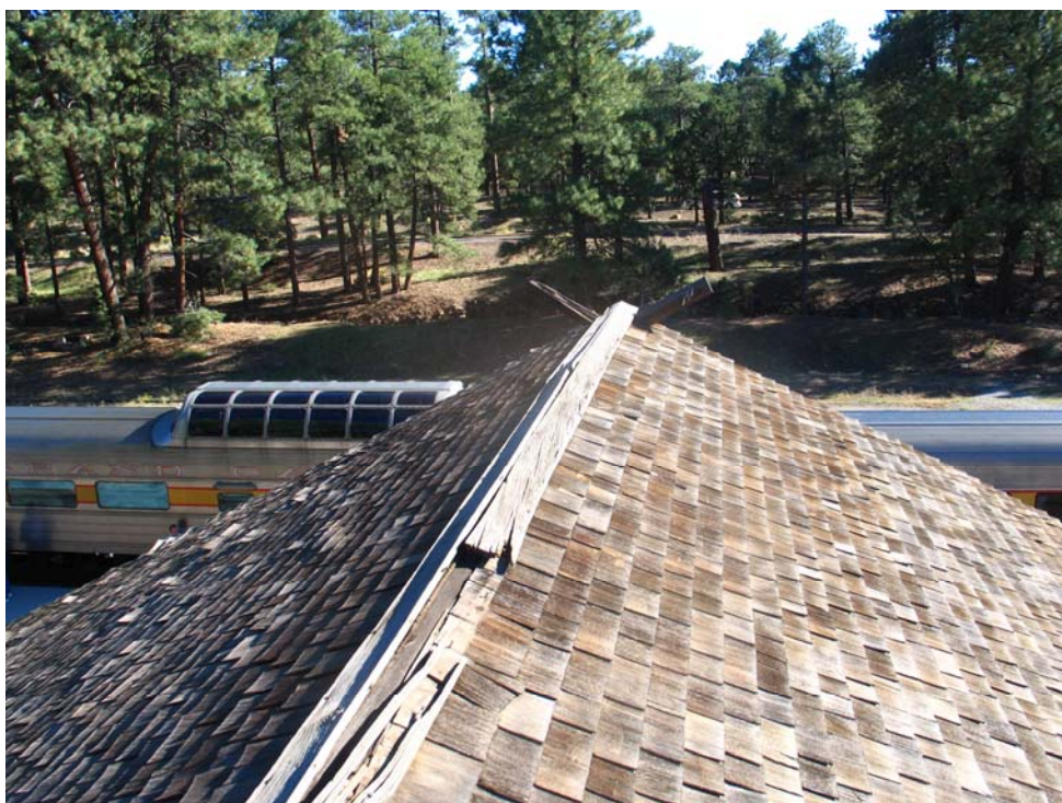
E-86 Main upper roof looking south. Note deterioration of ridge board and cupping of the shingles, particularly on the east side. October 3, 2007. Photograph by Martin/Martin.
