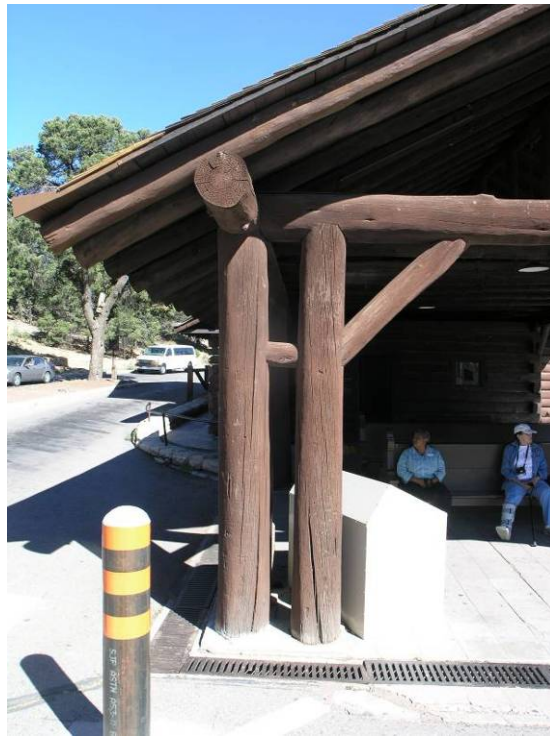
E-48 Northwest corner of covered waiting area, looking east. Note cracks in log columns. October 3, 2007. Photograph by Chamberlin Architects.
