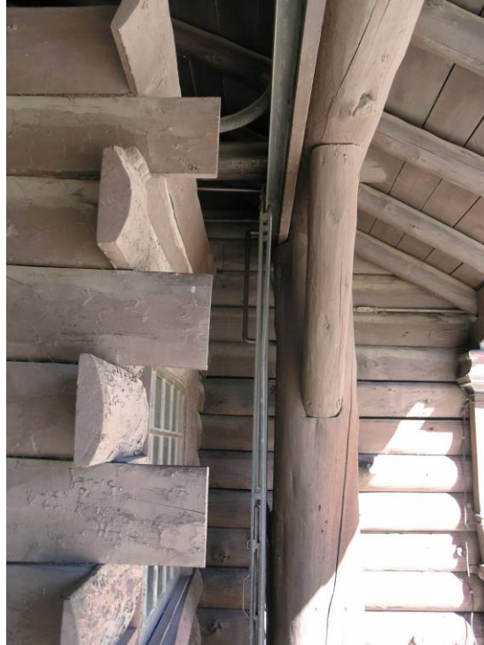
E-41 West façade, south side. Note collapsible gate and track. October 3, 2007. Photograph by Chamberlin Architects.
