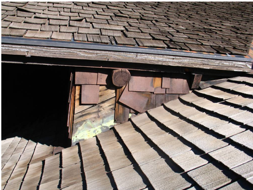
E-84 West side of dormer at Pantry. Note loss of shingles. Also note cupping of roof shingles. October 3, 2007. Photograph by Martin/Martin.
