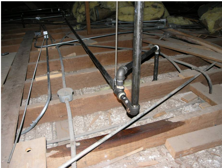
I-108 Attic space looking southwest. Note leak in fire sprinkler line. October 3, 2007. Photograph by Chamberlin Architects.
