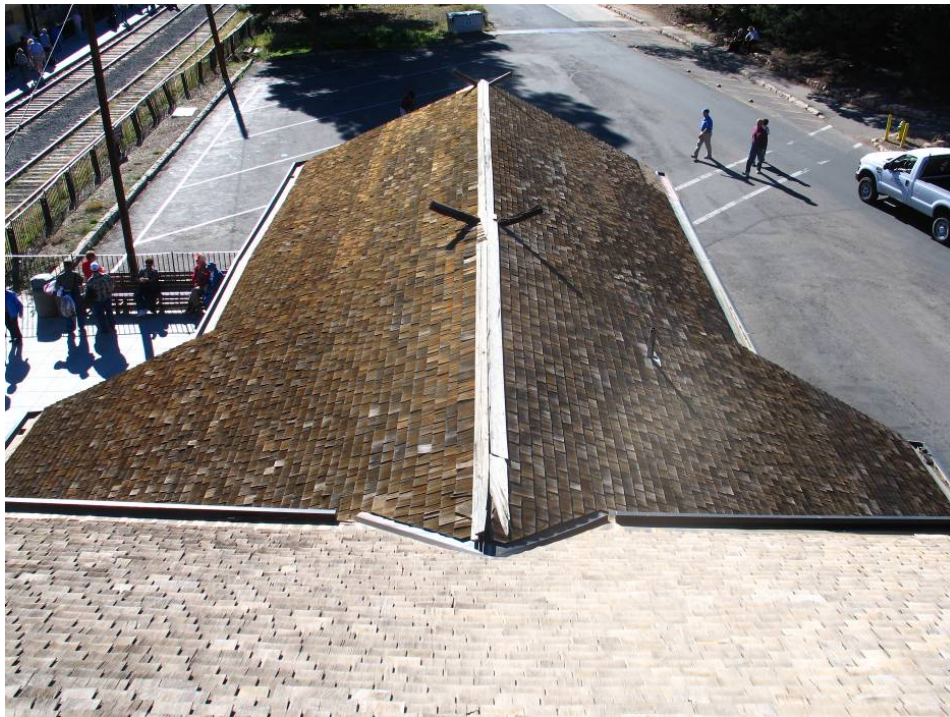
E-78 View of main roof looking west with west bedroom roof and covered waiting area roof beyond. Note damage to ridge boards. October 3, 2007. Photograph by Martin/Martin.
