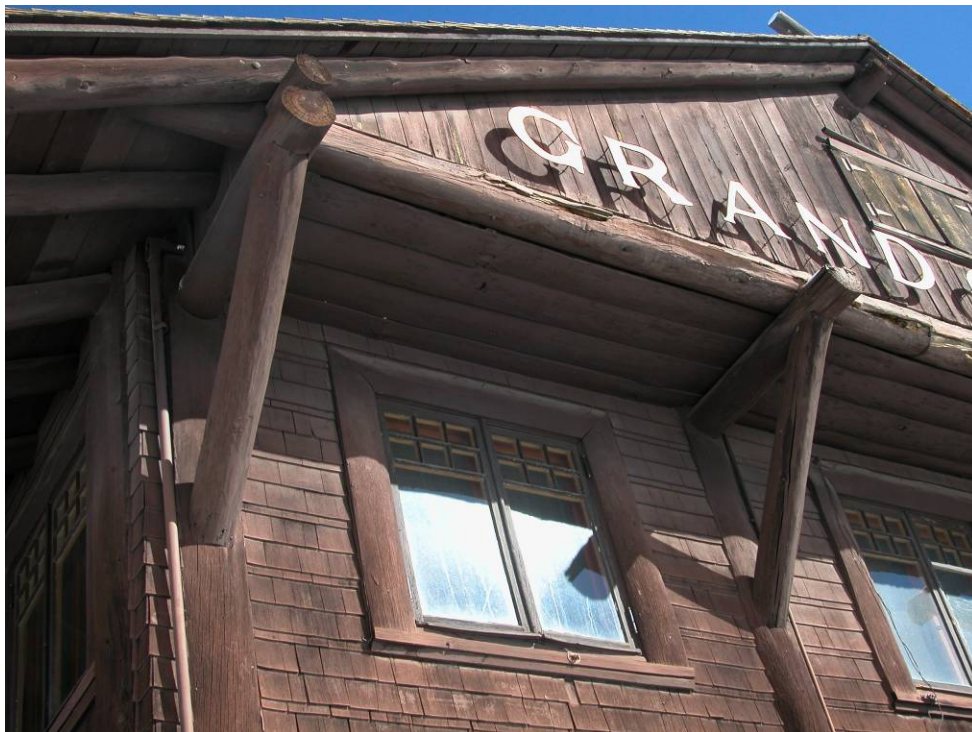
H-139 Grand Canyon Depot prior to rehabilitation. South elevation. Note deterioration of log beam. Date March 3, 2005. Scanned from building files.
