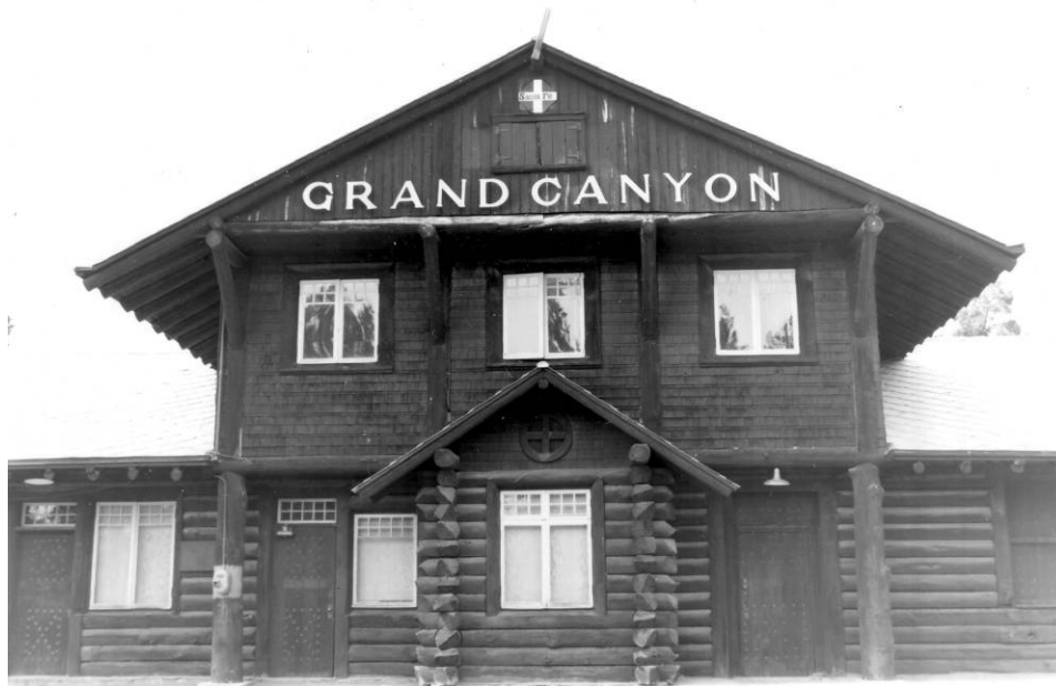
H-55 Santa Fe Railroad Depot, southern exposure. Note apparent deterioration of wood members of upper gable. Date 1976. NPS photo. NPS Catalog # GRCA 10736
