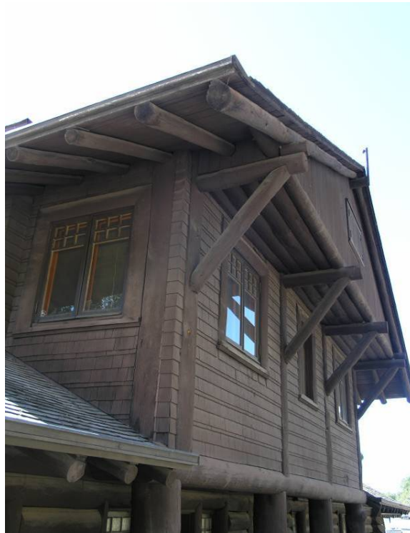
E-61 North façade, looking southwest. Window 205 is to the upper left. Note the wood piece nailed to the gable peak. This should be removed. October 3, 2007. Photograph by Chamberlin Architects.
