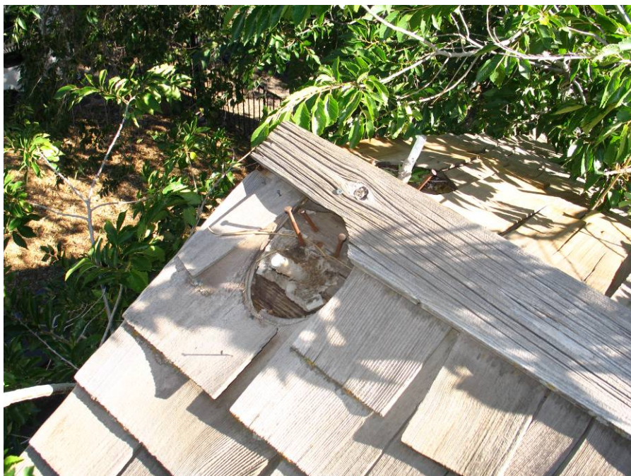
E-85 Evidence of missing barge rafter extensions at east roof. October 3, 2007. Photograph by Martin/Martin.
