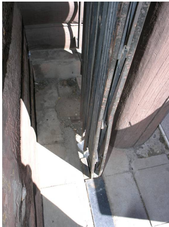
E-42 West façade, south side. East end of collapsible gate. Note base track is covered. October 3, 2007. Photograph by Chamberlin Architects.
