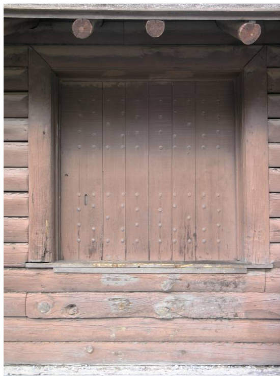
E-102 Door 104B. Note wear of logs below the door. Protection should be provided. October 3, 2007. Photograph by Chamberlin Architects.
