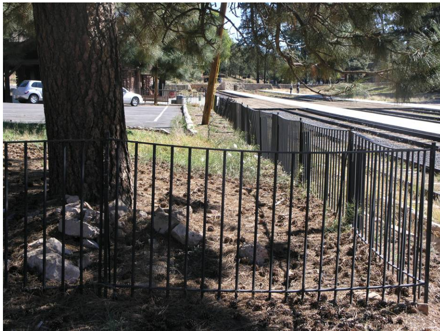
E-10 Metal fence, southwest corner of parking area. Note sag in rails. October 3, 2007. Photograph by Chamberlin Architects.
