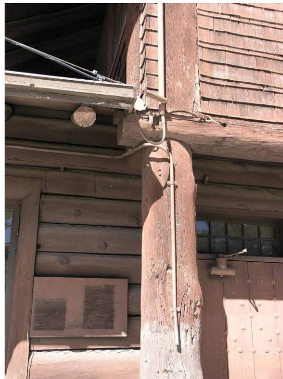
E-34 South façade. Door 102A to right. Note telephone cable and conduit attached to log column. These should be removed if possible. Also note discoloration of column. October 3, 2007. Photograph by Chamberlin Architects.
