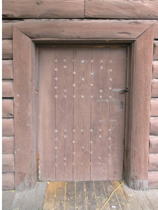
E-101 Door 104A. Note deterioration at base of casing. October 3, 2007. Photograph by Chamberlin Architects.
