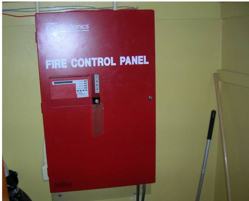
EL-8: Existing fire alarm control panel. Photograph by MKK.
