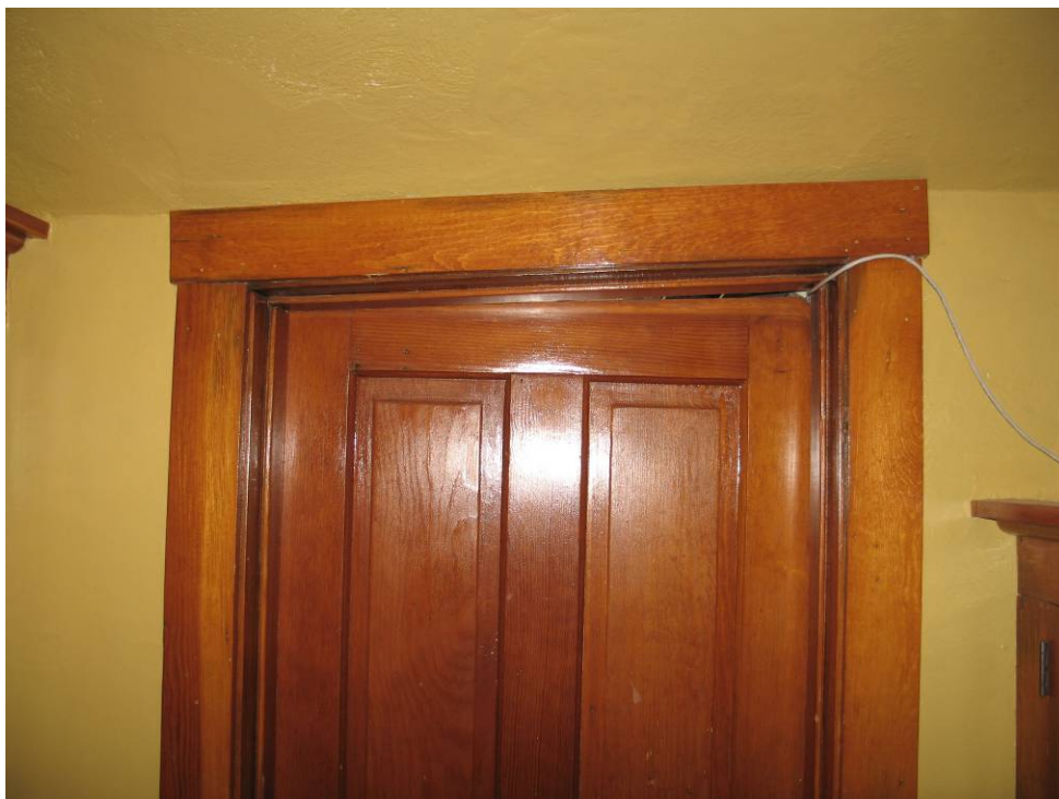
I-135 Head of Door 208A. Note door head and casing are cut to match slope of ceiling. Also note vertical orientation of door panels. October 3, 2007. Photograph by Chamberlin Architects.
