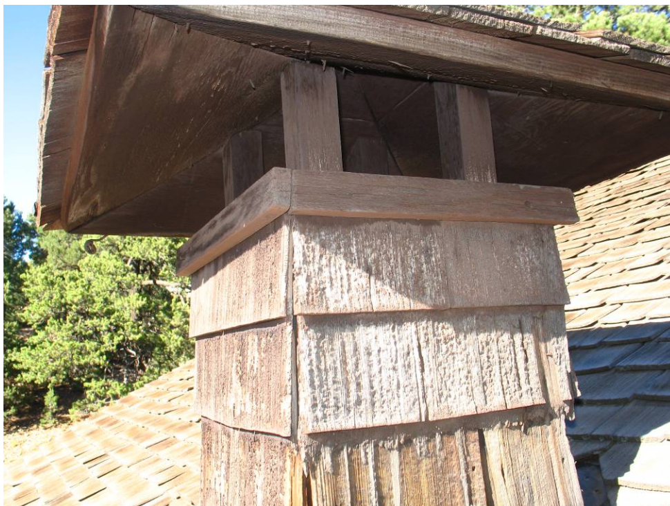
E-81 Close up of restroom vent. Note deterioration of wood shingles October 3, 2007. Photograph by Martin/Martin.
