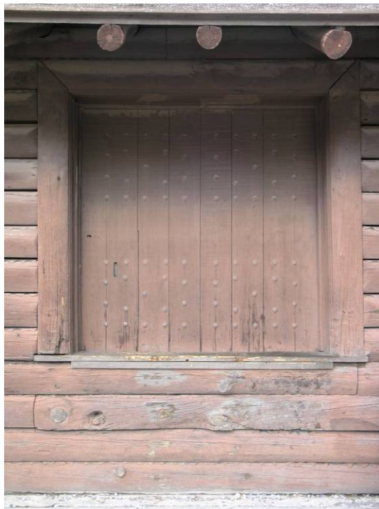
E-29 South façade, door to freight room. Door 104B. Note wear on logs below the door. October 3, 2007. Photograph by Chamberlin Architects.
