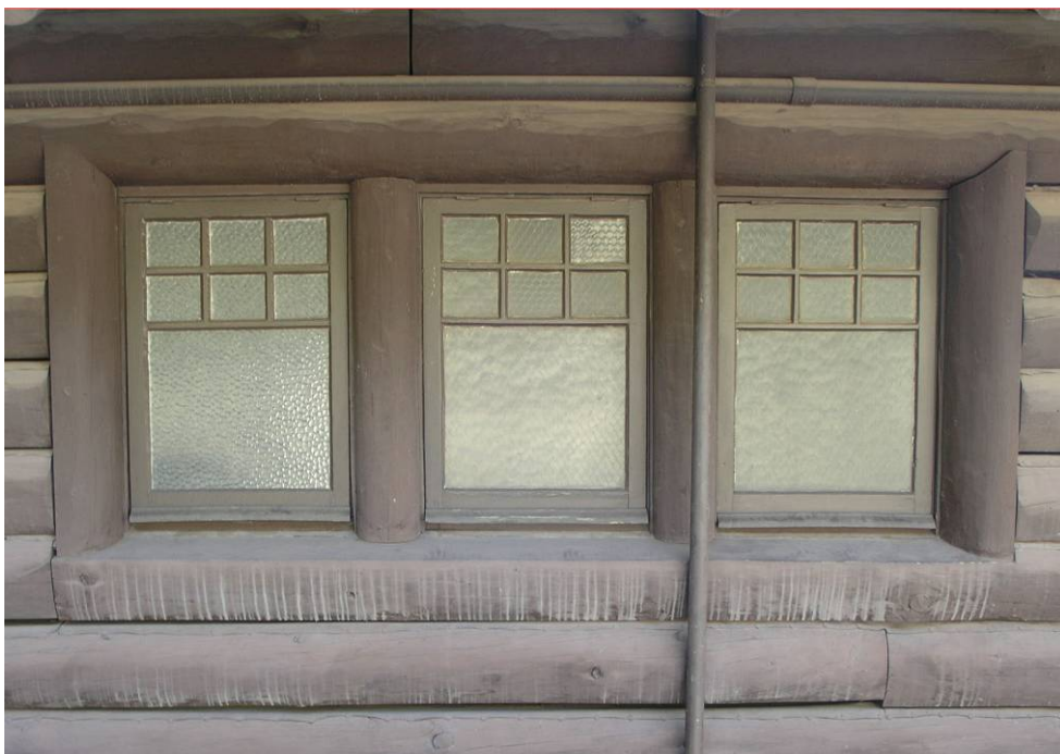
E-90 Windows 104, 103 & 102. Note the different type of glass in 104. October 3, 2007. Photograph by Chamberlin Architects.
