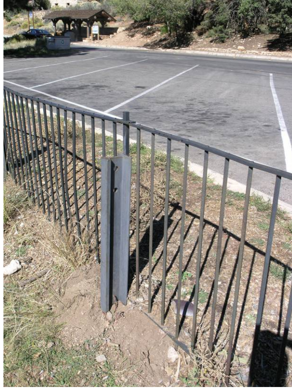
E-7 Metal fence along south side of parking area. Note steel rail for support and buried bottom rail. October 3, 2007. Photograph by Chamberlin Architects.
