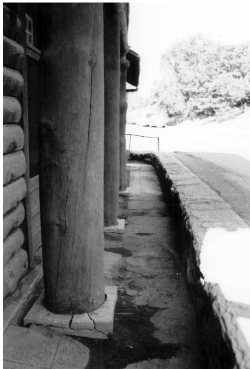
H-92 Grand Canyon Depot north side. Note cracked concrete column bases. Date assumed to be July 31, 1986. NPS photos. Scanned from building files.
