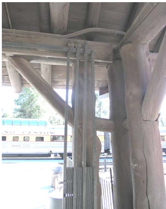
E-45 Southwest corner of covered waiting area. Note differential settlement of columns evident by the slope of the log spacer. October 3, 2007. Photograph by Chamberlin Architects.
