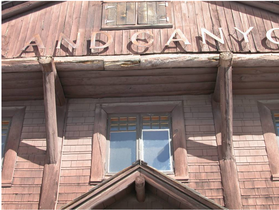
H-141 Grand Canyon Depot prior to rehabilitation. South elevation. Note deterioration of log beam. Date March 3, 2005. Scanned from building files.
