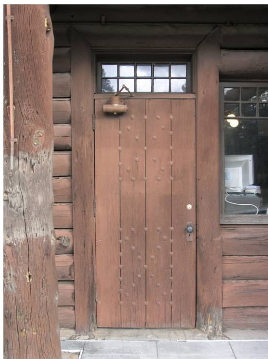
E-108 Door 102A. Note deterioration at base of casing. October 3, 2007. Photograph by Chamberlin Architects.
