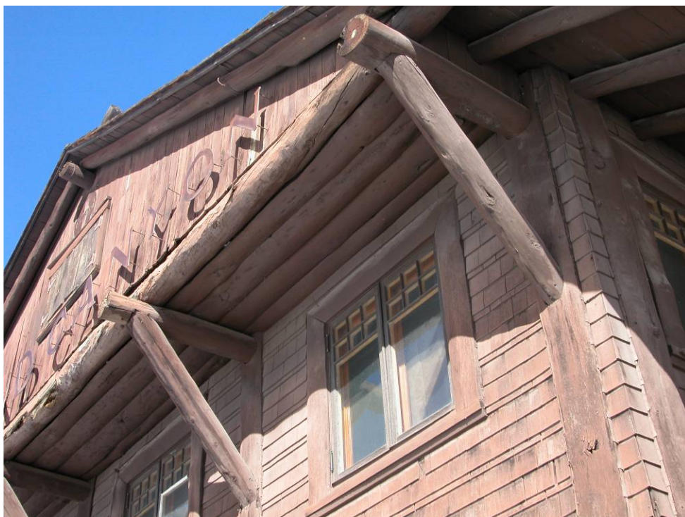
H-140 Grand Canyon Depot prior to rehabilitation. South elevation. Note deterioration of log beam. Date March 3, 2005. Scanned from building files.
