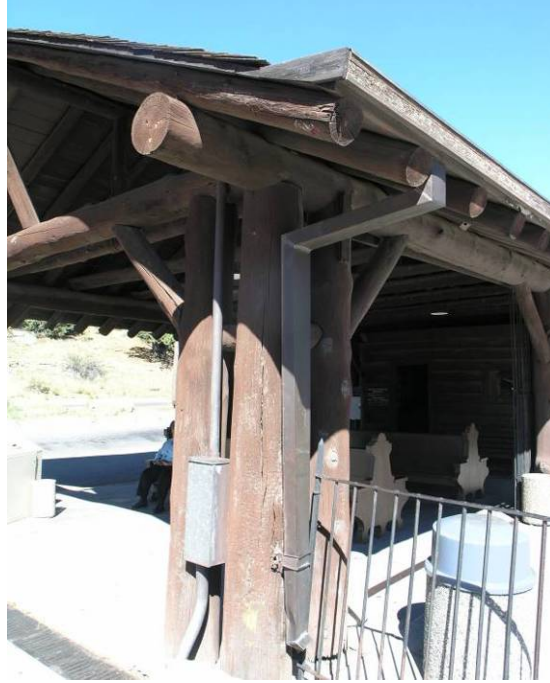
E-47 Southwest corner of covered waiting area looking northeast. Roof drain leader, added in 1986, is not historic. Note wrought iron fence to the right. October 3, 2007. Photograph by Chamberlin Architects.
