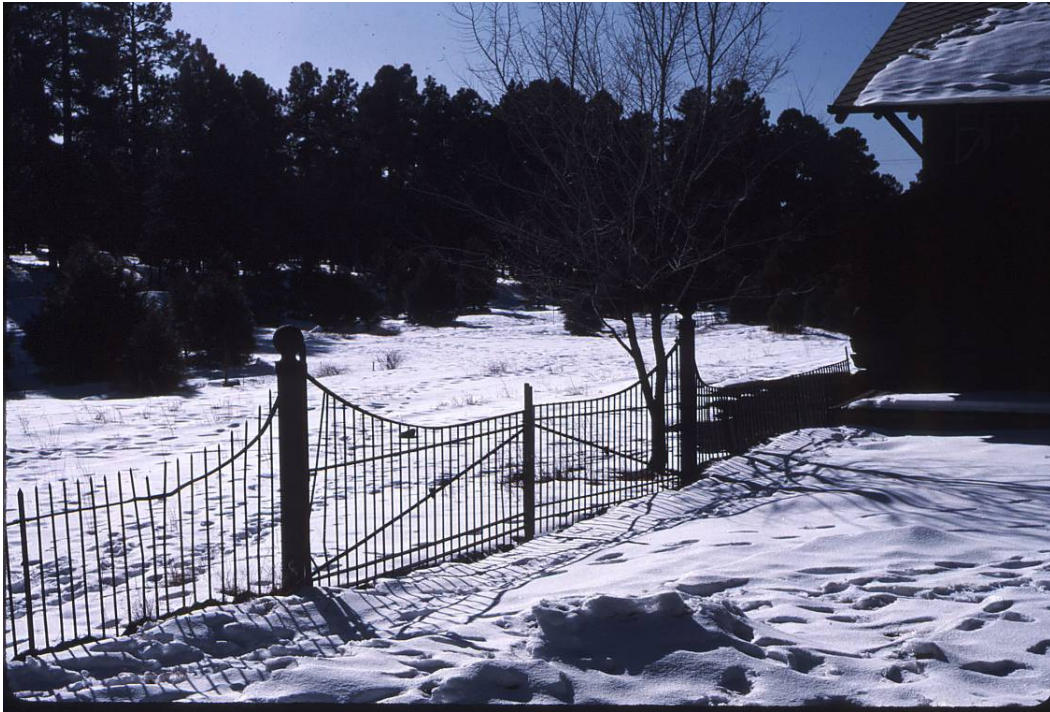
H-82 Grand Canyon Depot wrought iron gate at east end. Note that the fence finials are still in place on the east side of the gate. Compare to photos E-12 and E-13. Date 1984-1986. Scanned from building files.
