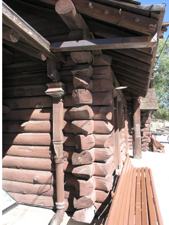
E-37 South west corner. Note that leader is disconnected from gutter on the right. October 3, 2007. Photograph by Chamberlin Architects.
