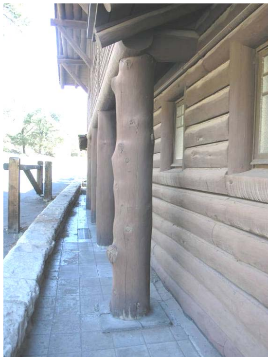
E-57 North façade, looking east. Note deterioration at column bases. Also note the gaps between some of the wall logs. October 3, 2007. Photograph by Chamberlin Architects.
