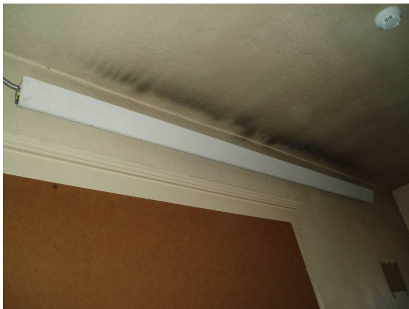
M-11: Cove Heater Discoloration. Photograph by MKK.
