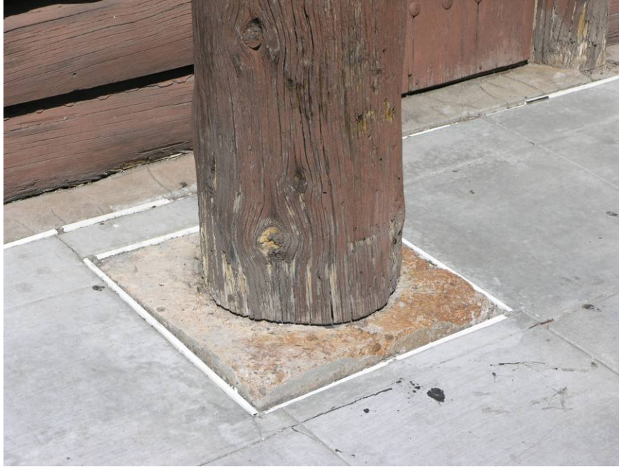
E-35 South façade, base of previous column. Note some deterioration around the base. October 3, 2007. Photograph by Chamberlin Architects.
