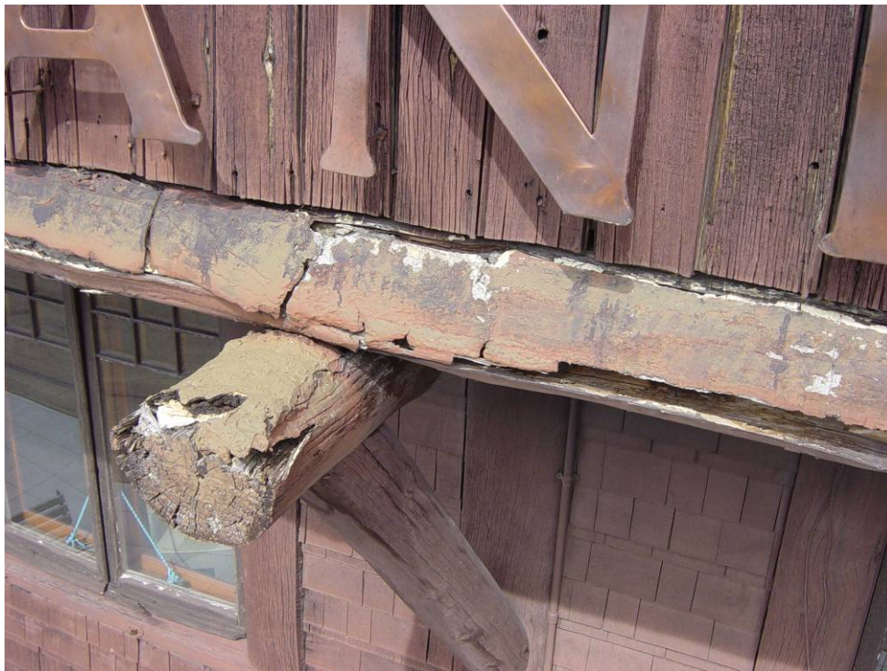
H-145 Grand Canyon Depot prior to rehabilitation. South elevation. Close up of east central bracket logs. Date March 3, 2005. Scanned from building files.
