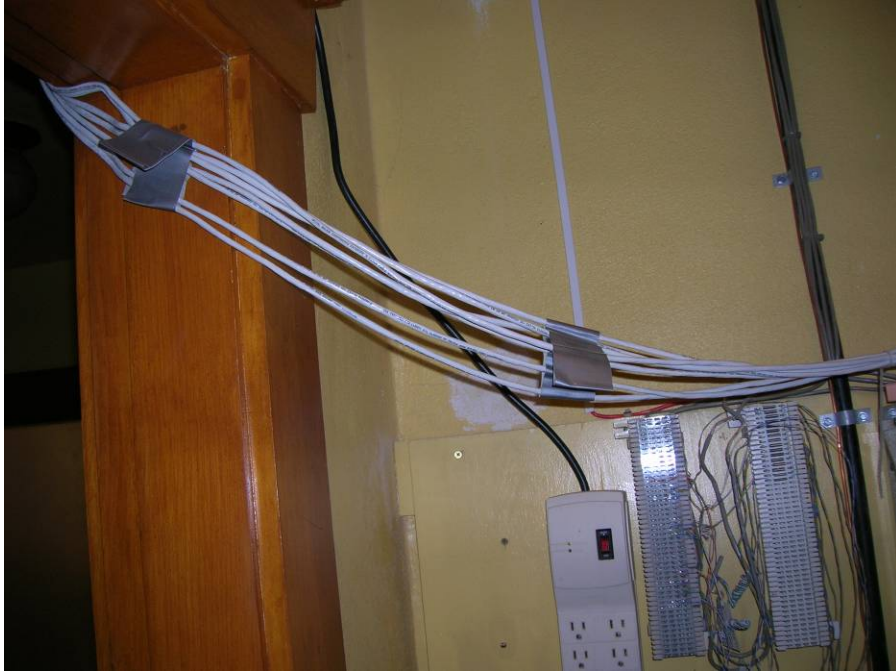
EL-7: Telecommunication cabling leaving closet. Photograph by MKK.
