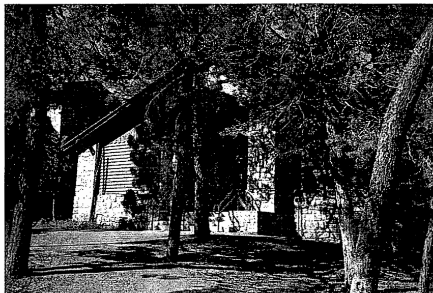
Photograph 225. Grand Canyon Middle School. Note pipe handrail on stair. (JMA, 2001)
