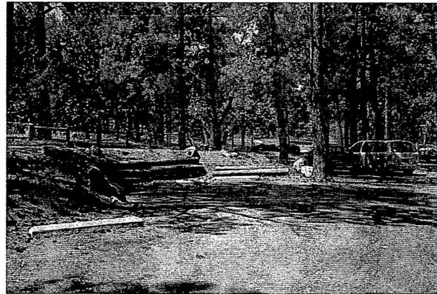
Photograph 150. Log retaining wall and wheelstops near General Office and Public Garage. (JMA, 2001)
