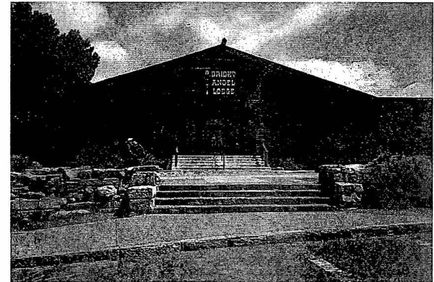
Photograph 30. Bright Angel Lodge south entrance. (JMA, 2001)
