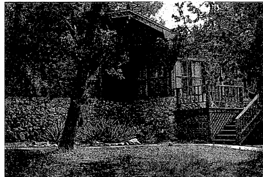
Photograph 205. Residence #5 Apache Street (Bldg. #0822), with ornamental vegetation in yard. (JMA, 2001)
