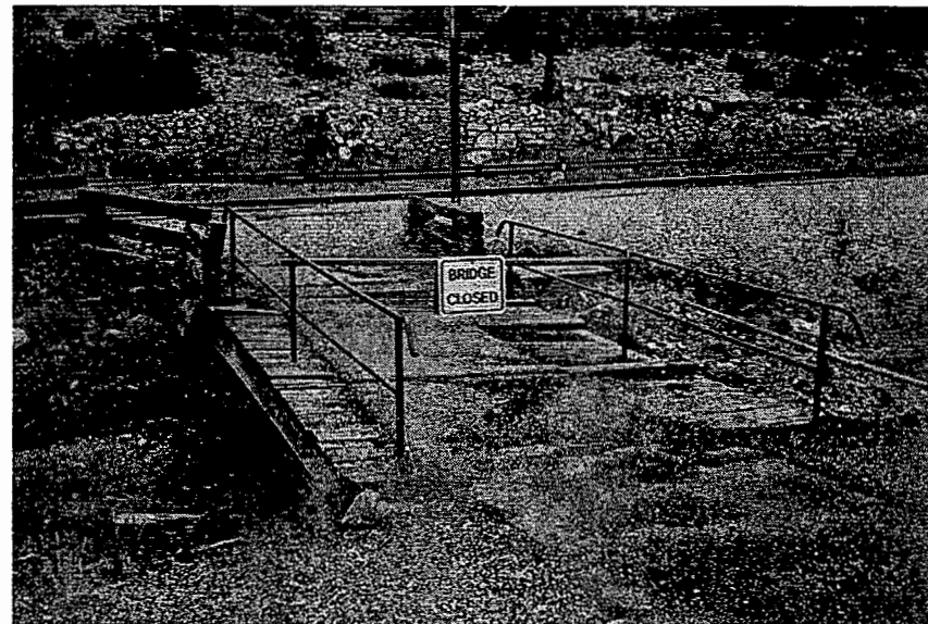
Photograph 117. Wood and asphalt bridge. (JMA, 2001)
