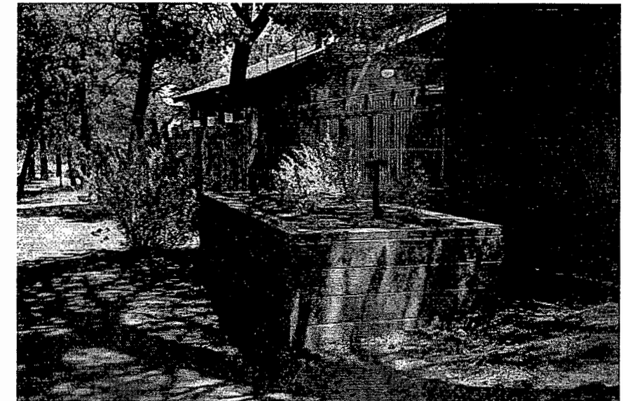
Photograph 143. Concrete masonry unit planting bed. (JMA, 2001)
