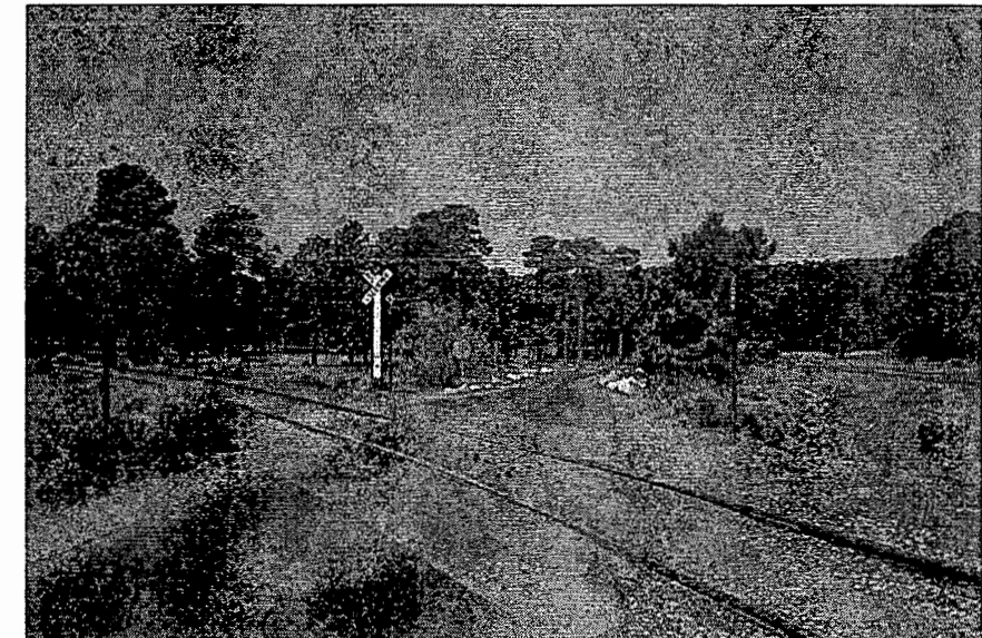
Photograph 110. Old Village Bypass Road at crossing of tracks. (JMA, 2001)
