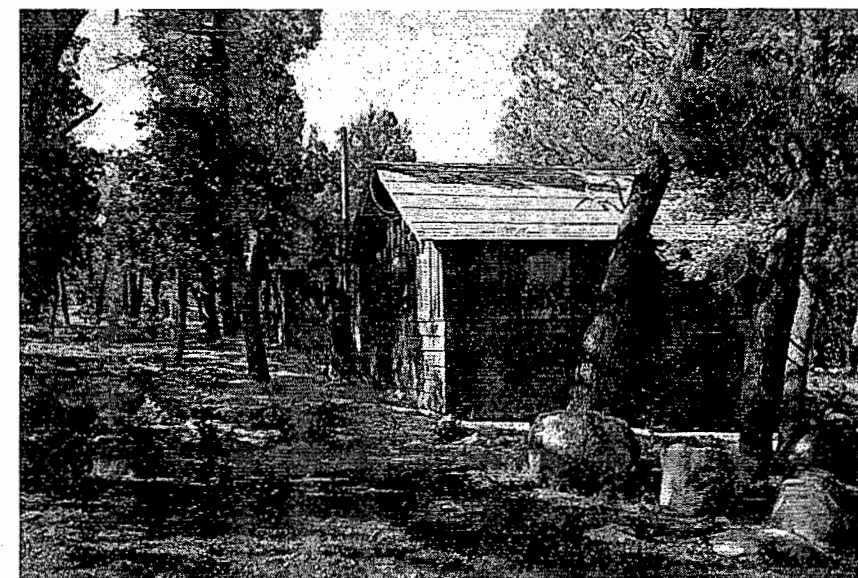
Photograph 180. Labor Cabins and Ponderosa pines. (JMA, 2001)
