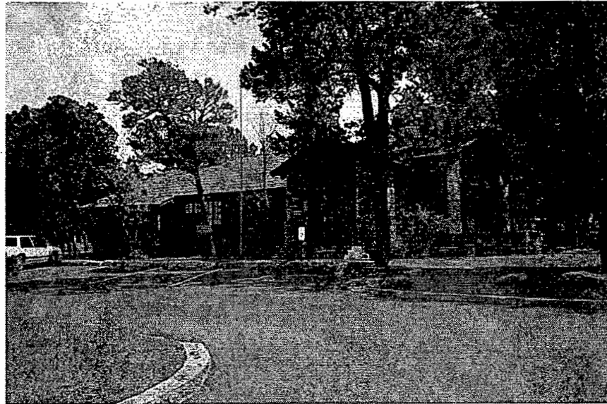
Photograph 138. Magistrate's Office with parking lot. (JMA, 2001)
