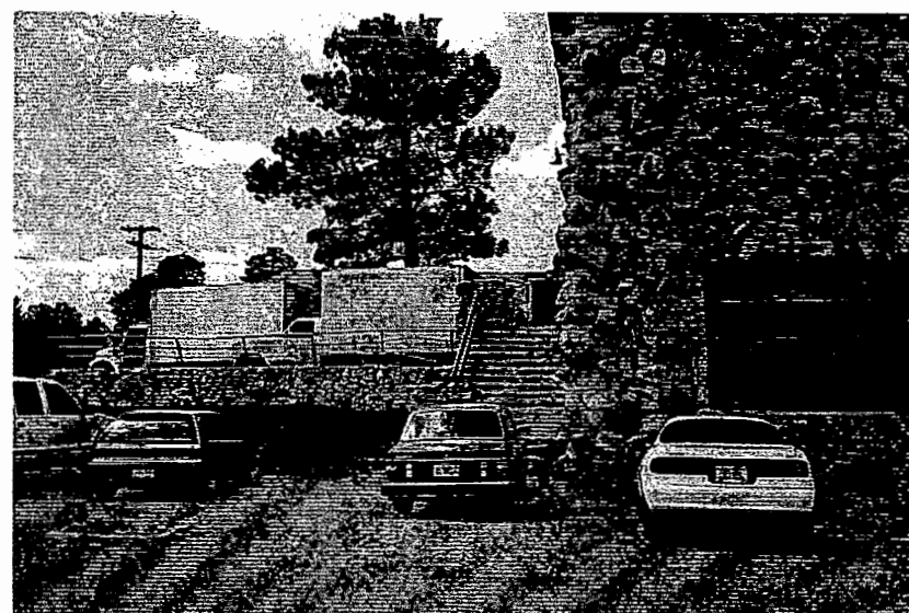
Photograph 86. Concrete steps, rubble stone retaining wall at Power House. (JMA, 2002)
