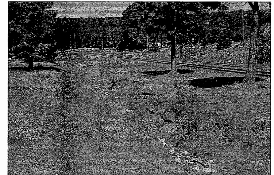
Photograph 106. Drainage ditch along tracks. (JMA, 2001)
