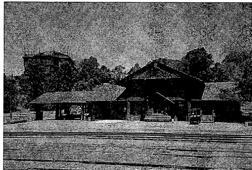
Photograph 114. Railroad Depot from south. (JMA, 2001)
