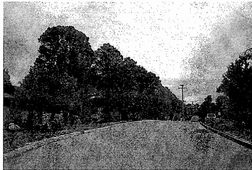
Photograph 197. Coconino Street section with curb. (JMA, 2001)
