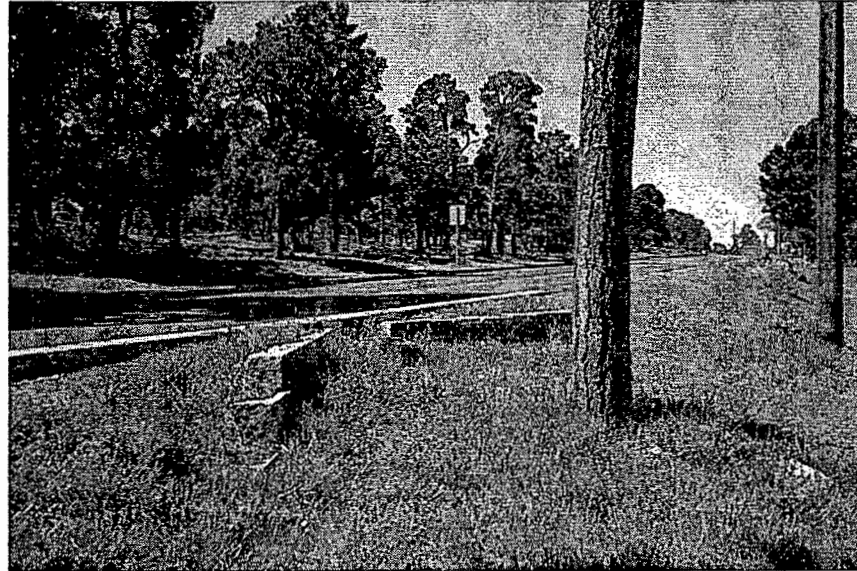
Photograph 97. Cut stone curb blocks used as tree guards along Village Loop Drive bank. (JMA, 2001)
