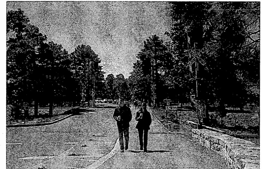
Photograph 126. Railroad crossing gate and sign, cut stone curbing along Village Loop Drive. (JMA, 2001)
