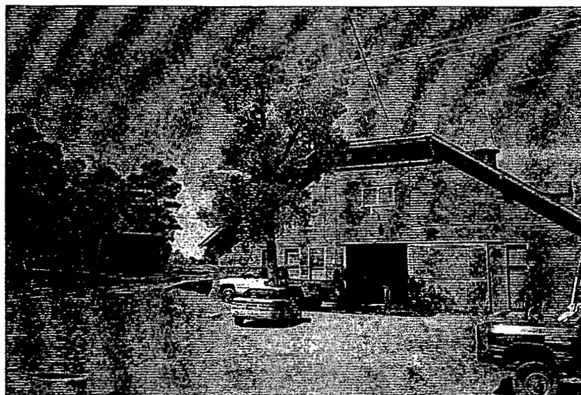
Photograph 87. Livery Stable. (JMA, 2001)
