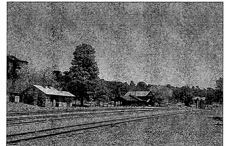
Photograph 108. Railroad Depot node and tracks. (JMA, 2001)
