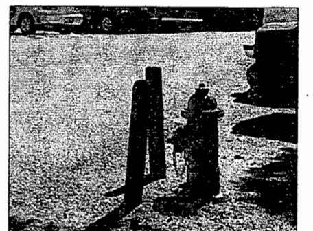
Damaged and inadequate bollards
