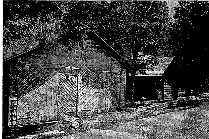
Photograph 166. Garage and shed at Bldg. #SRQ0004. (JMA, 2001)
