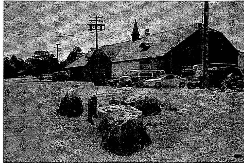
Photograph 98. Fire hydrant and protective boulders. (JMA, 2001)
