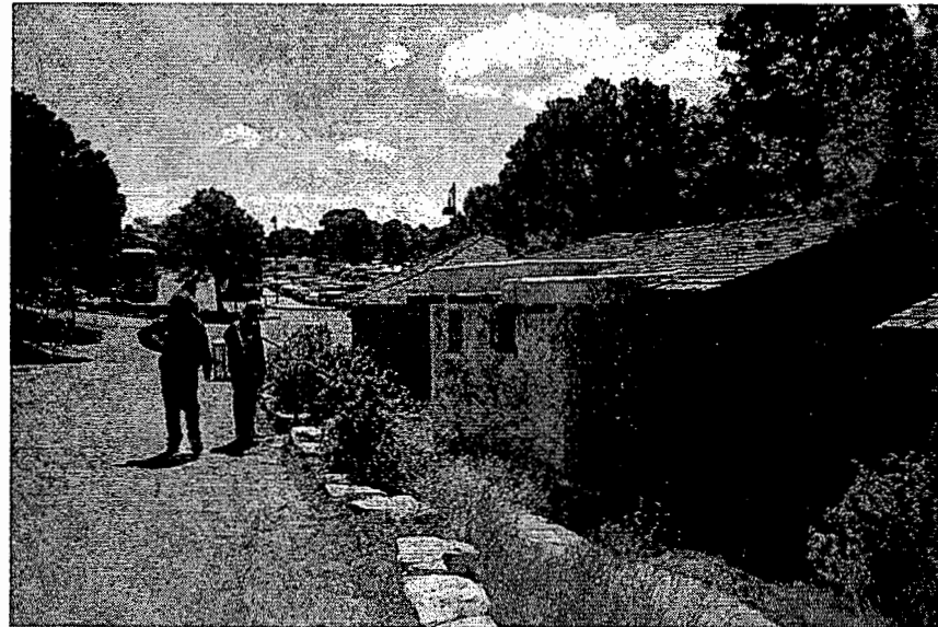
Photograph 25. Bright Angel Cabins. Note stone edging along road. (JMA, 2001)
