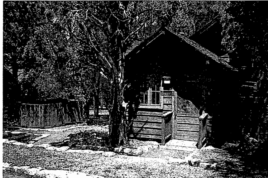
Photograph 165. Single family residence #8 Tonto St. (Bldg. #SRQ0003). (JMA, 2001)
