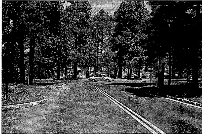
Photograph 132. Intersection of Center Road and Village Loop Drive. (JMA, 2001)
