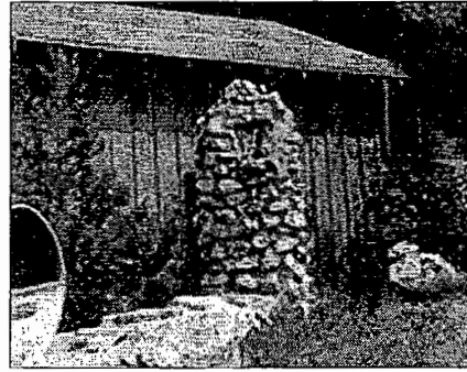
Remnant stone pier
