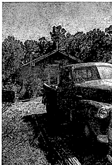
Photograph 171. Single family residence #53 Juniper Hill (Bldg. #SRQ0053), with gravel parking and wood edging. (JMA, 2001)
