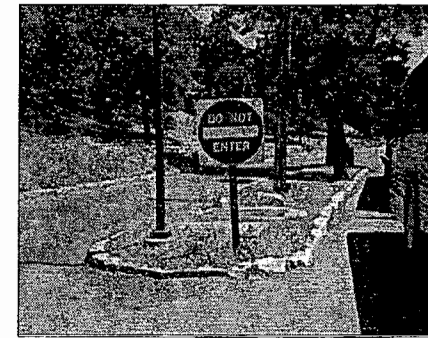
Excessive signage in historic median
