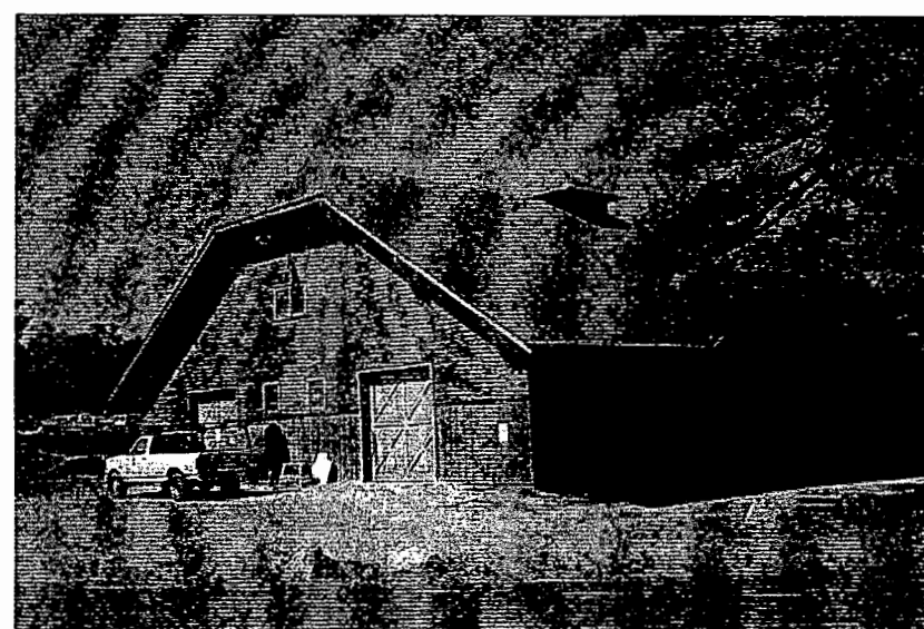
Photograph 88. Eastern facade of the Mule Barn. (JMA, 2001)
