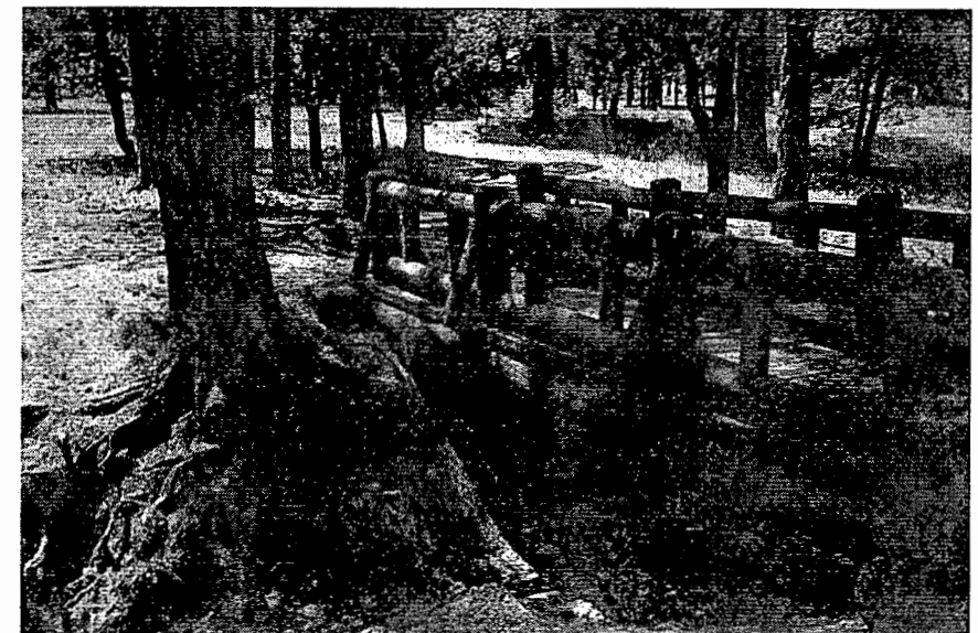
Photograph 118. Peeled-log bridge. (JMA, 2001)
