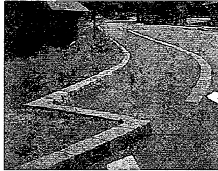
Cut stone curbing
