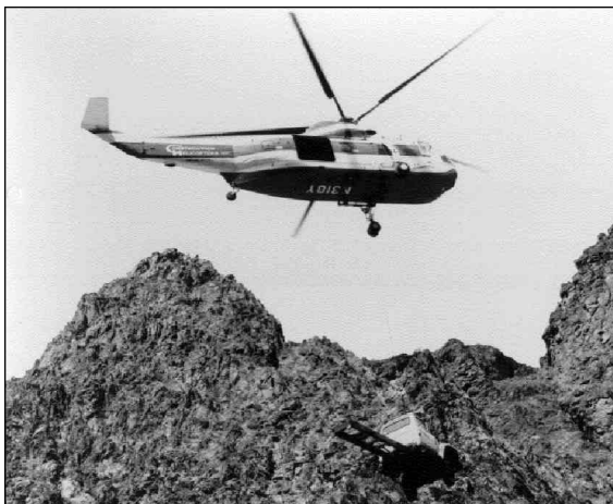
Figure 43.A Sikorsky S-61 carrying a truck down to Phantom Ranch to facilitate construction of the trans-canyon pipeline May 1968. GRCA 5208.
