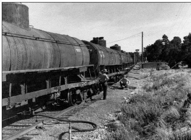
Figure 17. Twenty 10,000-gallon tankers deliver water from the Chinle Valley to South Rim storage tanks, 1961. The Santa Fe supplied water in this manner from 1901 until the late 1960s—daily until 1932 and as needed thereafter. GRCA 3605.
