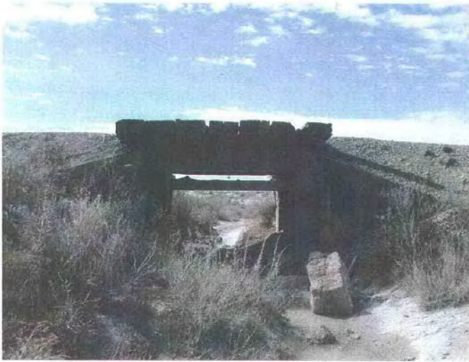
Wooden Culvert, Transcontinental Railroad National Backcountry Byway
