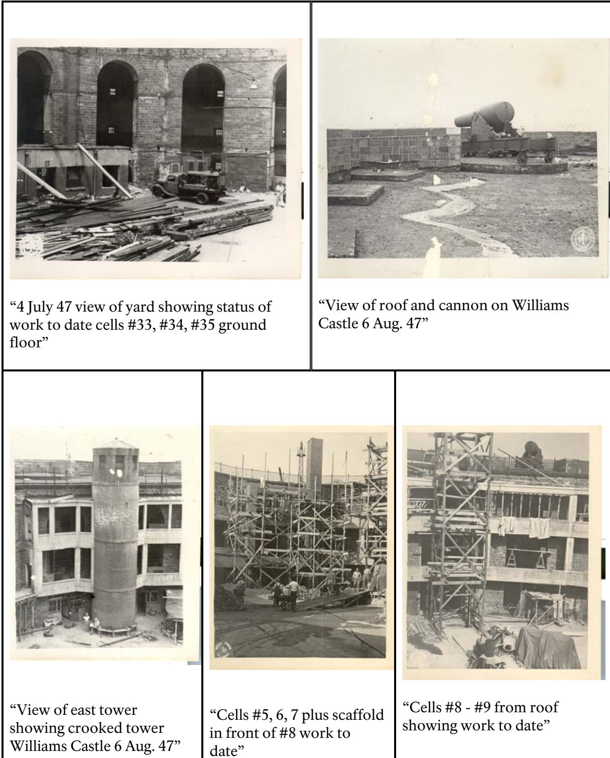
Figure 43. Construction photographs of Castle Williams with original captions, 1947.
