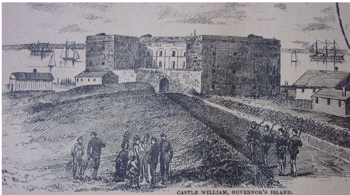
Figure 24. East elevation of Castle Williams, 1886.
