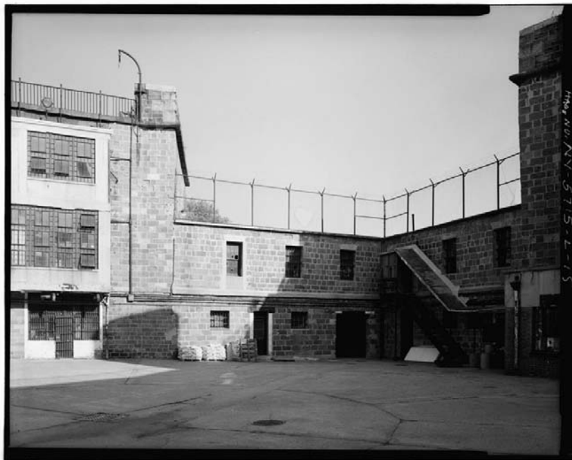
Figure 55. Interior southeast elevation of Castle Williams, 1982- 83.
