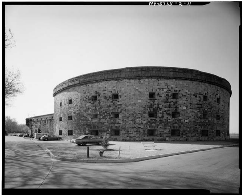
Figure 54. Exterior east elevation of Castle Williams, 1982- 83.
