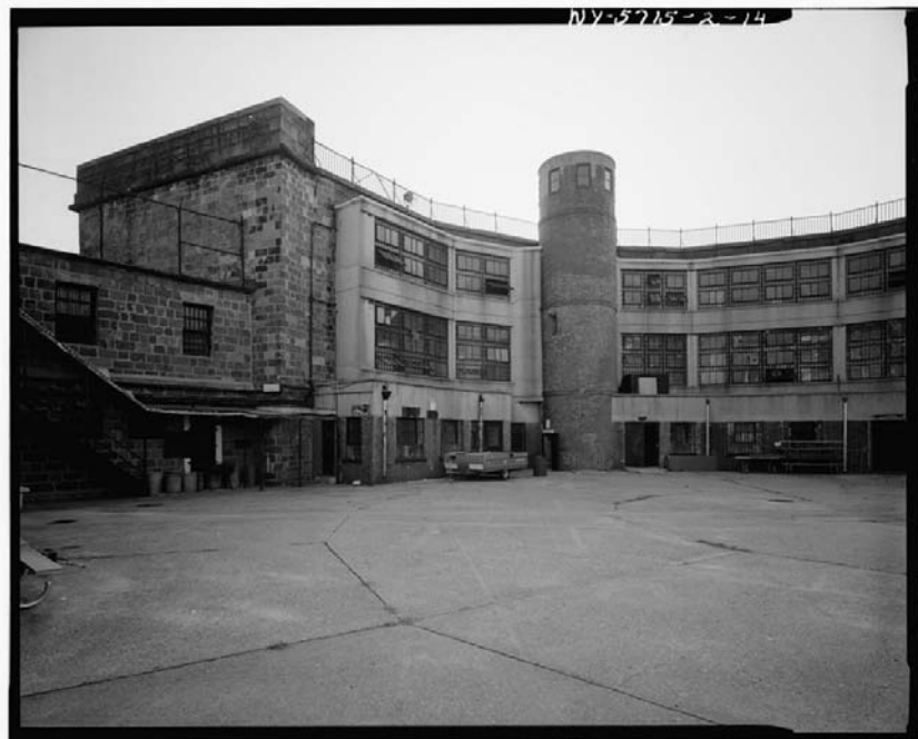
Figure 56. Interior south elevation of Castle Williams, 1982- 83.
