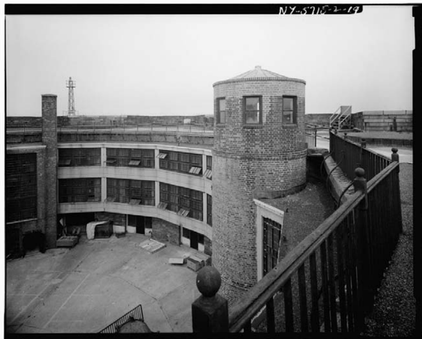
Figure 60. View looking west from the northeast barbette tier of Castle Williams, 1982- 83.
