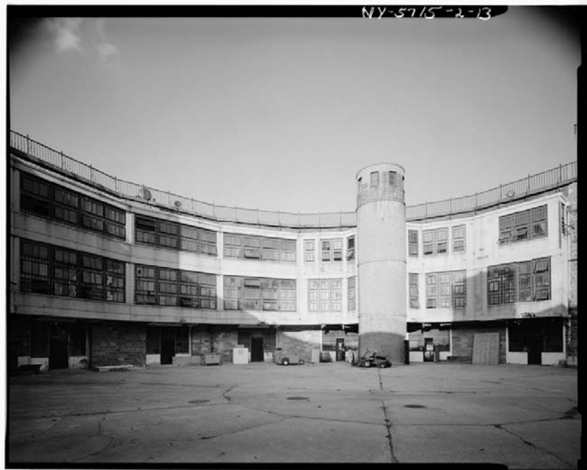
Figure 58. Interior northeast elevation of Castle Williams, 1982- 83.
