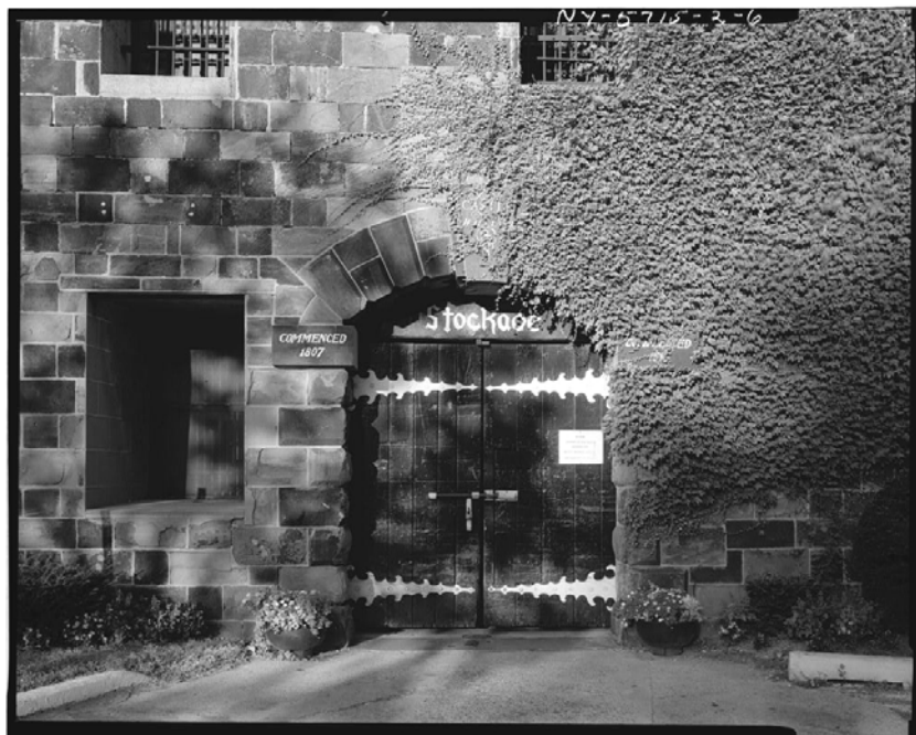
Figure 47. Exterior sally port [entrance] of Castle Williams, 1982- 83.
