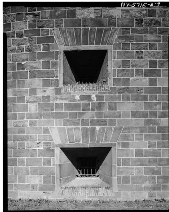
Figure 52. Detail of exterior embrasures in the first and second tiers of Castle Williams, 1982- 83.
