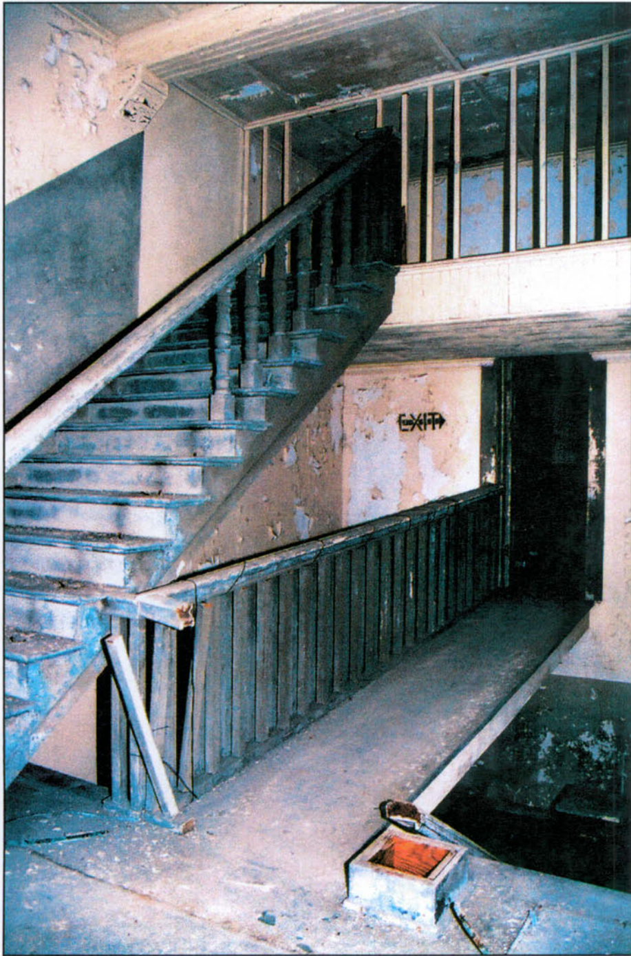
Stair 01 at third floor landing, 2003. Photo Credit: John Martini.
