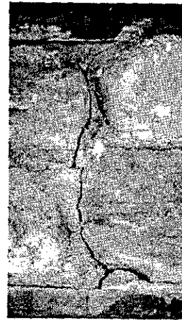
Photograph 96: Typical cracking above door and window openings.
