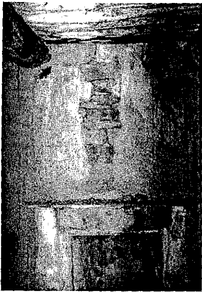
Photograph 193: Wall erosion above fireplace
