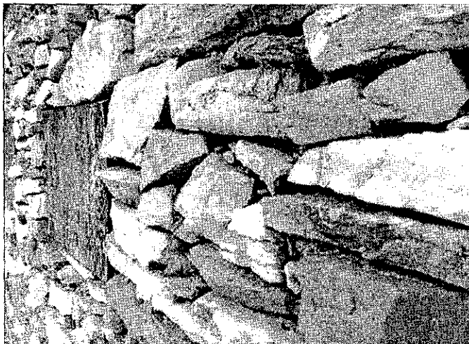
Photograph 237: Detail of wall jointing.
