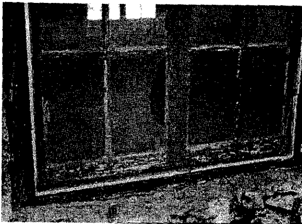
Photograph 95: Weathering of wood windows.
