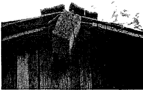
Photograph 50: Detail of twisted ridge beam
