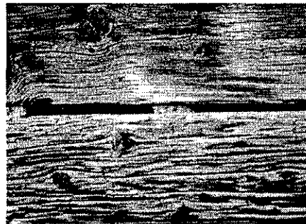
Photograph 51: Detail of log weathering and eroded chinking
