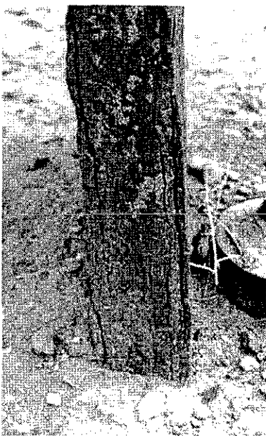
Photograph 148: Sandstone delamination
