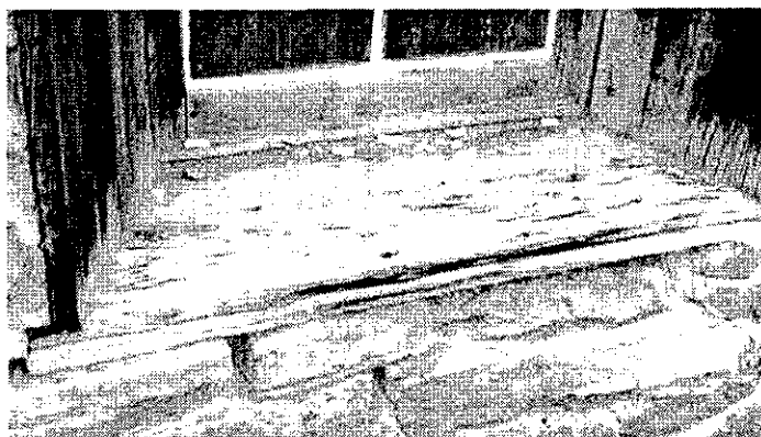
Photograph 213: Deteriorated sill at south window.
