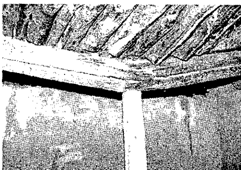
Photograph 191: Collapsing roof structure supported on shoring.
