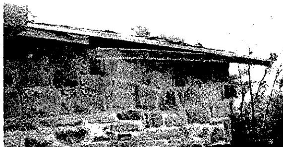
Photograph 254: Deteriorating fascia at west eave.
