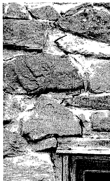
Photograph 209: Crack above south window.
