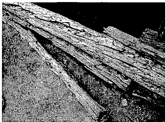
Photograph 119: Detail of sill damage below window.
