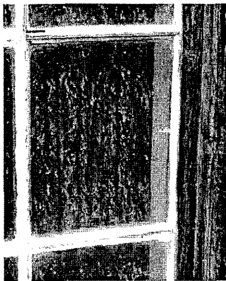
Photograph 211: Failure of glazing putty at window.
