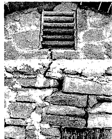
Photograph 238: Crack through west vent.
