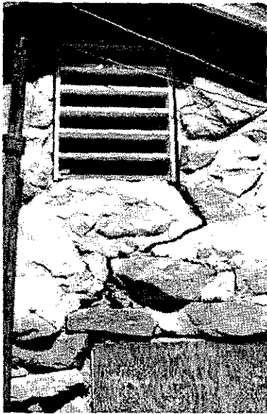
Photograph 234: Crack at east vent.
