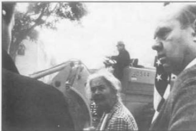
Preservationists in Lexington, Kentucky, attempt to stop the destruction by a redevelopment bulldozer of one of the oldest buildings in the city, November, 1969. Courtesy, National Register Branch, National Park Service (WASO).
