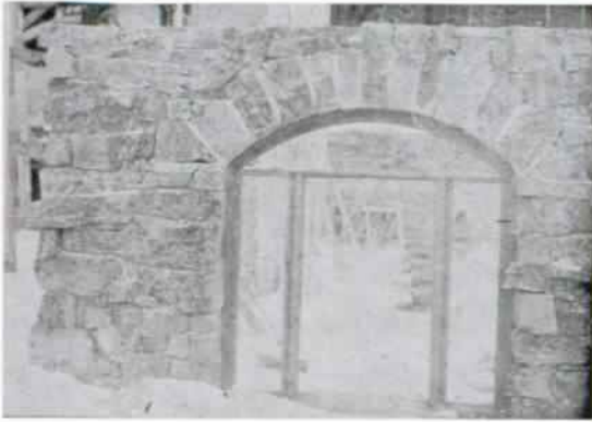
The stone segments creating the arched windows were constructed from locally quarried stone. Courtesy of Minnesota Historical Society
