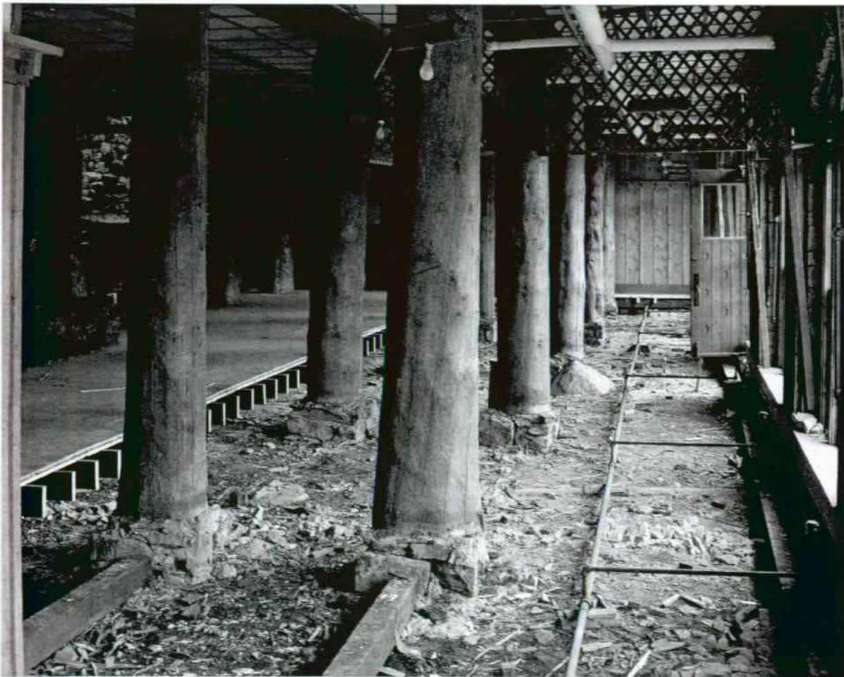
Base of original log columns set in main building. The typical peeled log column measured approximately 36 inches at its base and reduced to approximately 30 inches at its peak. This photo shows the floor of the Grill Room opened for repair work to bad concrete bases under log columns in 1952. Courtesy Glacier National Park Archives
