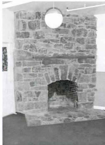
Corner fireplace in Deluxe Guestrooms. Note obtrusive contemporary light fixture. 2001 Courtesy Glacier National Park
