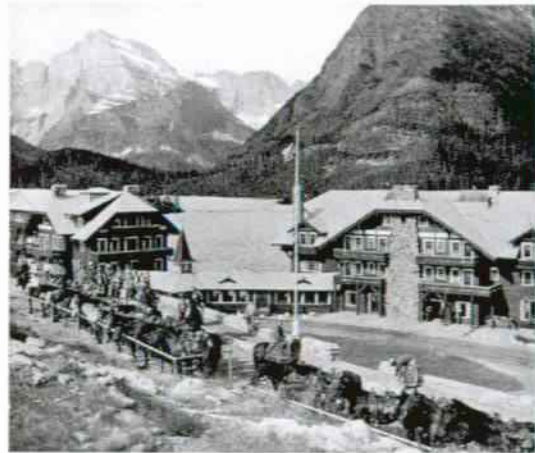
Note flagpoles and weather vane atop south bridge cupola, 1932. Courtesy Glacier National Park Archives
