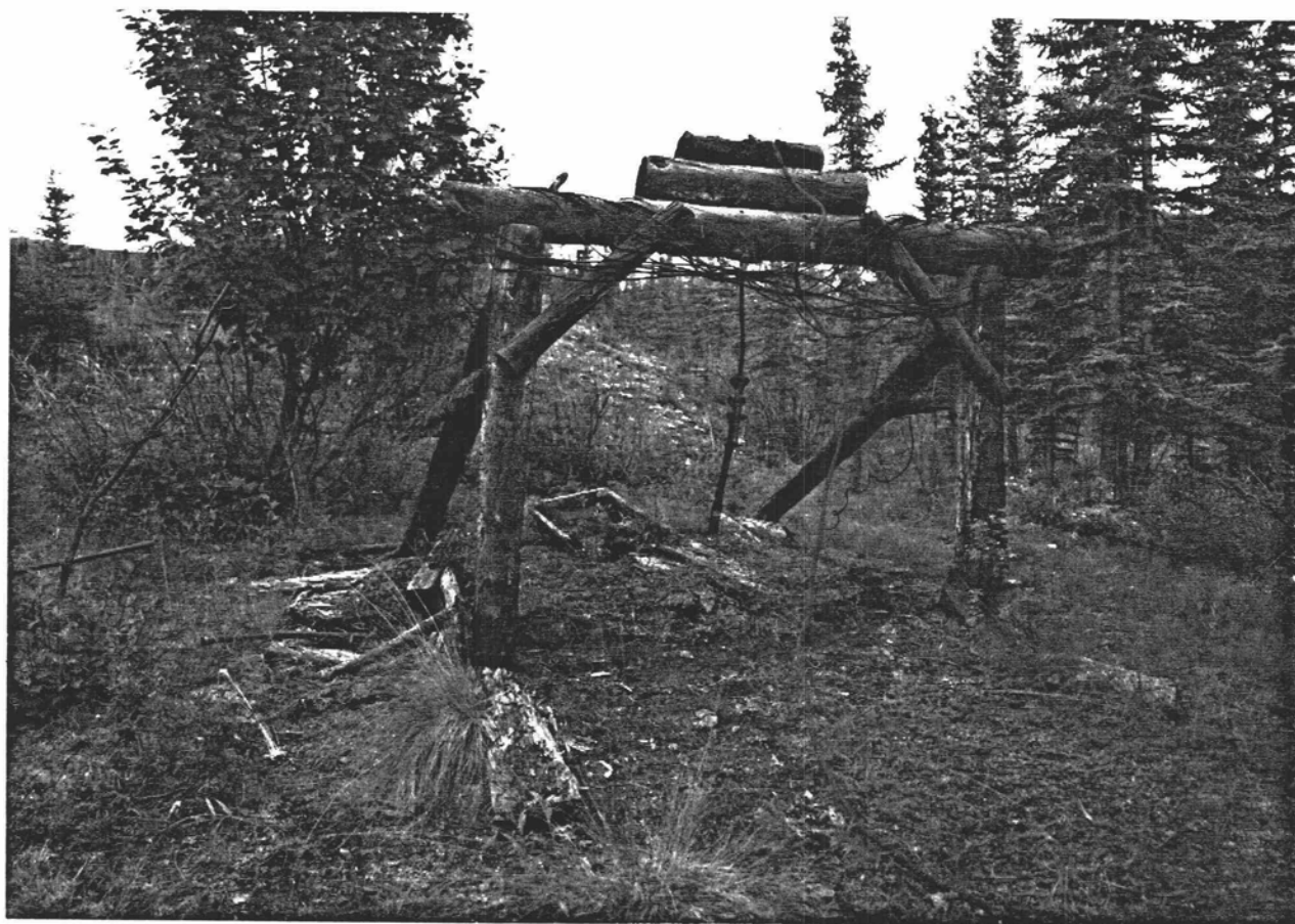
Linda Creek Complex: headframe over drift mine shaft. Jet Lowe, HAER photo.
