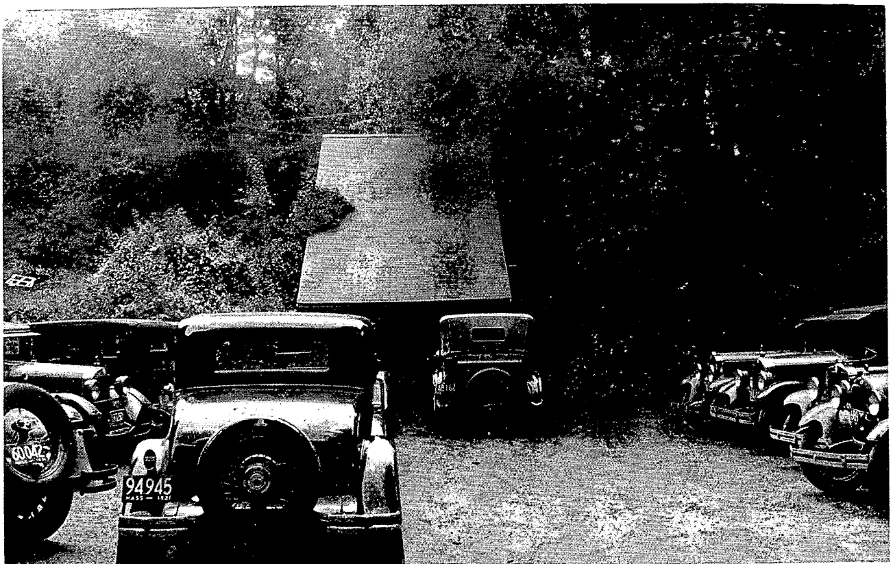
May 1931. Parking Lot and Shed. View West.
