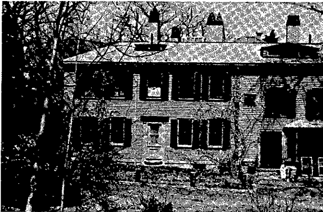
NORTHWESTERLY ELEVATION OF OLMSTED HOME
