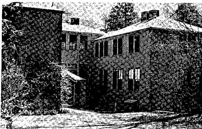
REAR VIEW OF OFFICE SECTION
