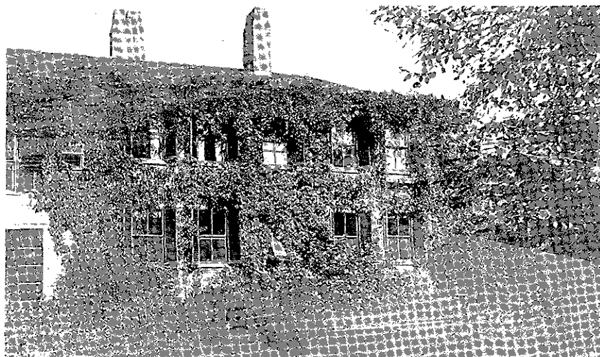
(4.30) South facade of house. Undated. Photograph #673-[not numbered] (album #2).
