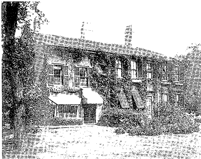
(2.48) South facade of house. Undated. Photograph #673-44.
