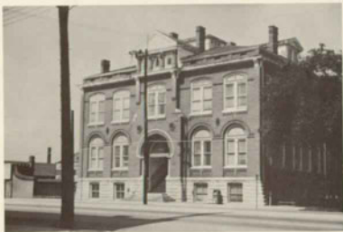
11. Central of Georgia offices at 233 West Broad St. (NPS 8/20/65)
