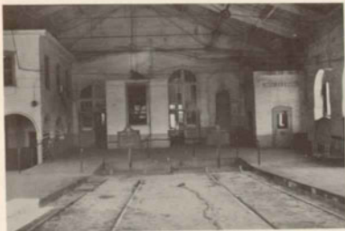
8. Interior of terminal train shed showing historical markers (NPS Photo 8/20/65)
