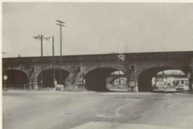
12. Southernmost of two Central of Georgia brick viaducts spanning Highway 17A (NPS Photo 8/20/65)
