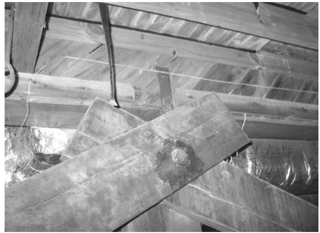
FIGURE 25. View of typical pile-beam-crossbrace
