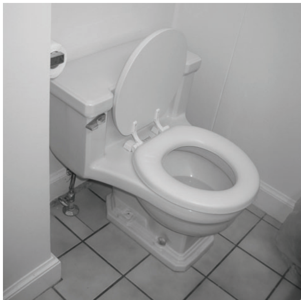
FIGURE 56. View of historic toilet in bathroom 104. (NPS-SERO-CR, 2003)
