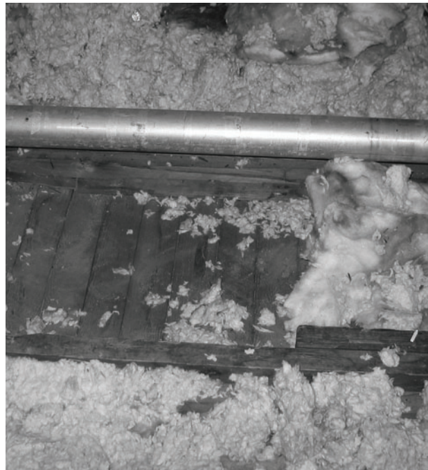
FIGURE 33. View of typical ceiling joists, with original tongue-and-groove ceiling paneling visible beneath modern insulation. (NPS-SERO-CR, 2003)
