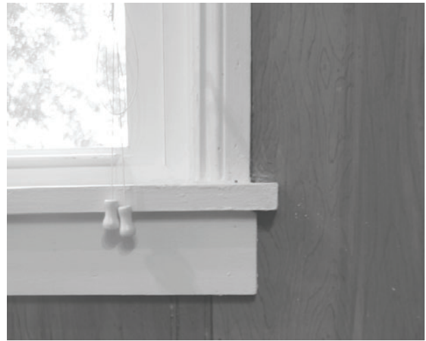
FIGURE 46. View of typical historic window stool and apron. (NPS-SERO-CR, 2003)
