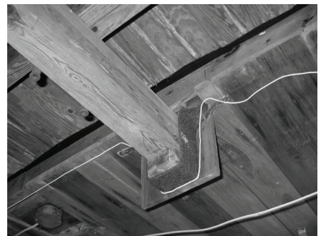
FIGURE 27. View of typical cast-iron U-shaped bracket used to hang beams for porch floor joists. (NPS-SERO0CR, 2003)
