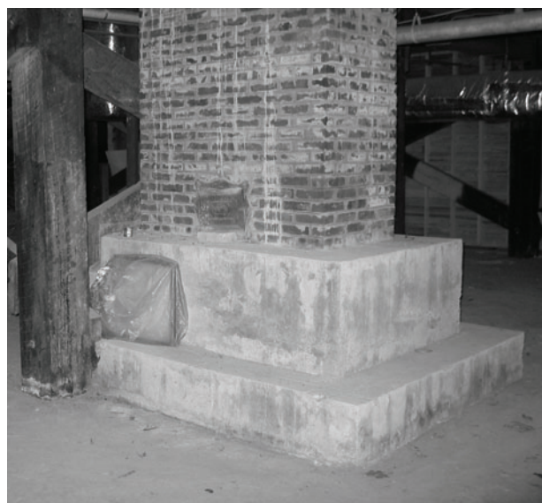
FIGURE 29. View southwest of chimney breast. (NPS-SERO-CR, 2003)
