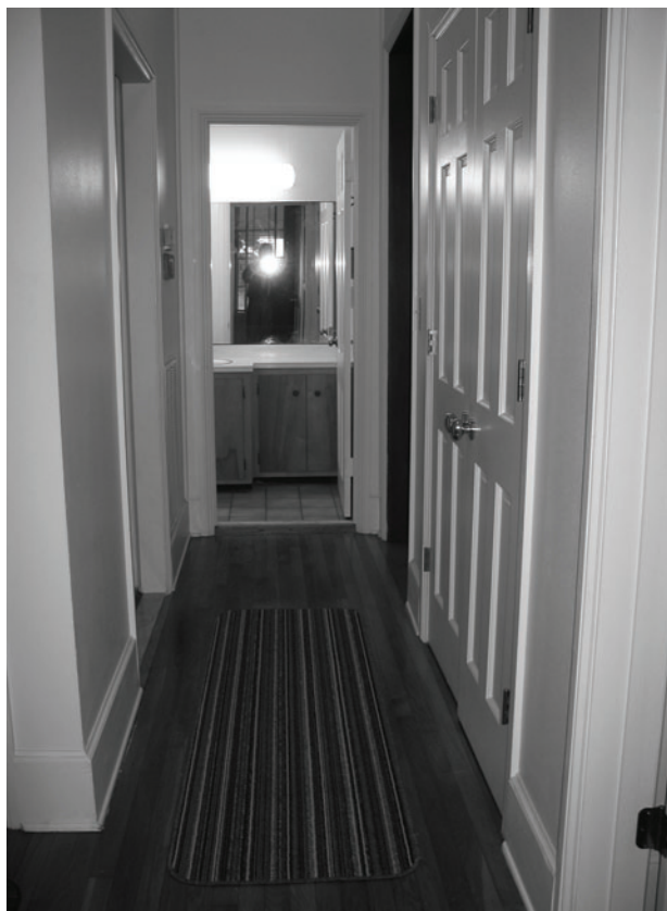
FIGURE 55. View north in hall toward bathroom 104. (NPS-SERO-CR, 2003)
