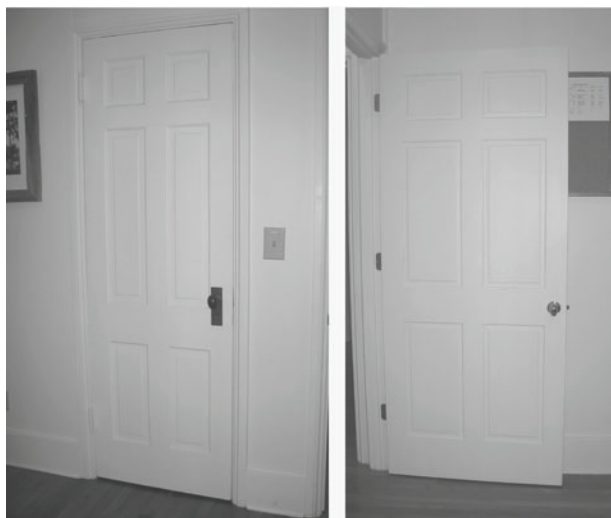
FIGURE 43. View of typical historic six-panel doors installed in 1942, left, and typical modern six-panel door installed in 2002. (NPS-SERO-CR, 2003). (NPS-SERO-CR, 2003)
