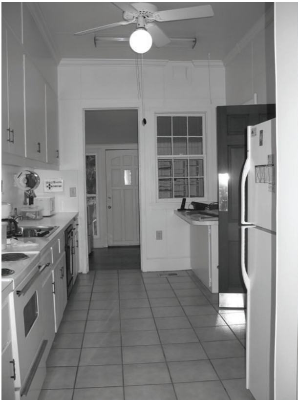
FIGURE 66. View west in kitchen, Room 108. (NPS-SERO-CR, 2003)
