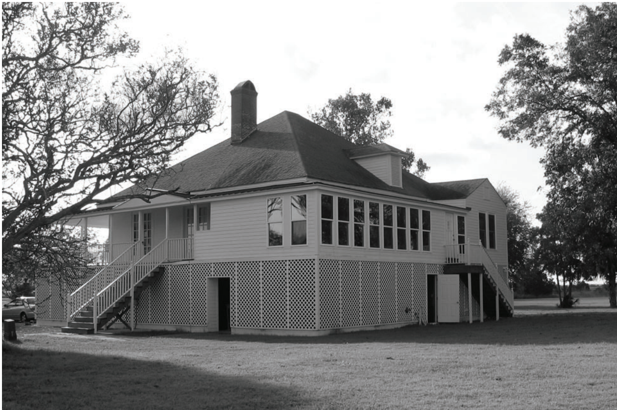
FIGURE 21. View of building from northwest, 2003. (NPS-SERO-CR, 2003)
