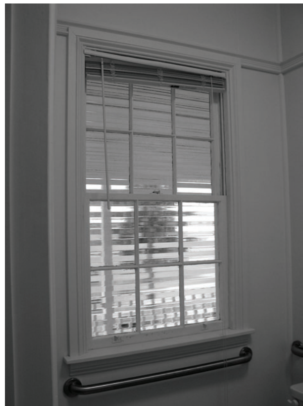
FIGURE 40. View of translucent, prismatic glass in bathroom. (NPS-SERO-CR, 2003)
