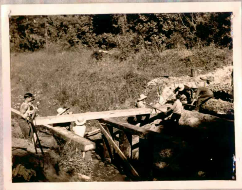
CCC enrollees of Georgia EM-1, building a wooden bridge on bridge path at Robert Jechner Park.
