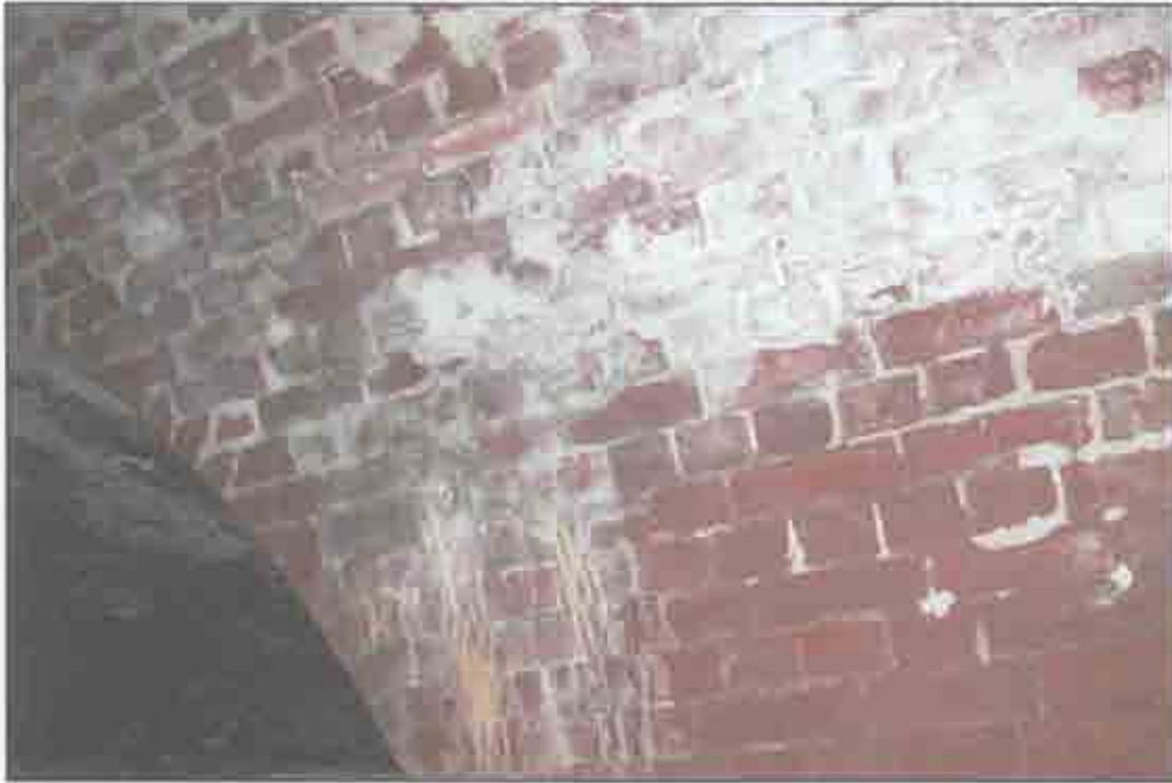
Condition Photo 3: Casemate 101; Calcium deposits are draining from open joints and coating is no longer extant. (Courtesy of ARG, 2003)
