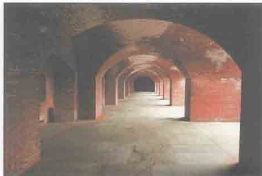
Typical brick casemate with arched ceilings and granite floors. (John Martini, 2005)
