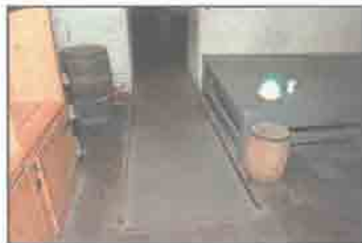
The reconstructed banquette on the right would have doubled as a platform to fire into the sallyport and a sleeping area for the guards. (John Martini, 2005)
