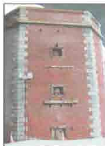
The west face of the west bastion has the remains of a fog bell and other structures that were attached to the sides of the fort. (Jane Lehman, 2005)
