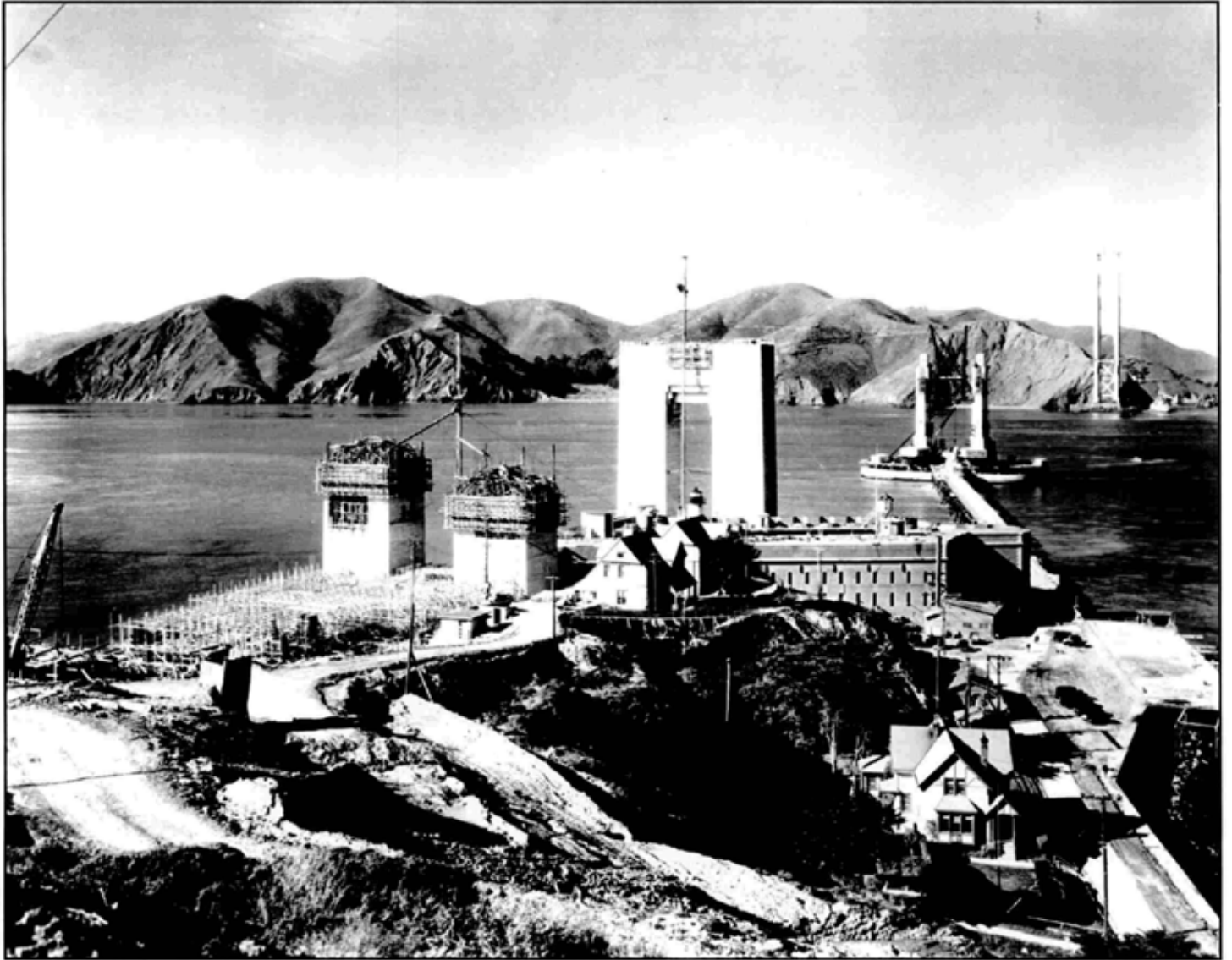
Figure 16. Photograph: Golden Gate Bridge construction, Lighthouse Keeper's Houses, viewed from bluff above Fort, circa 1933. Credit: Fort Point NHS Collection, Golden Gate National Recreation Area.
