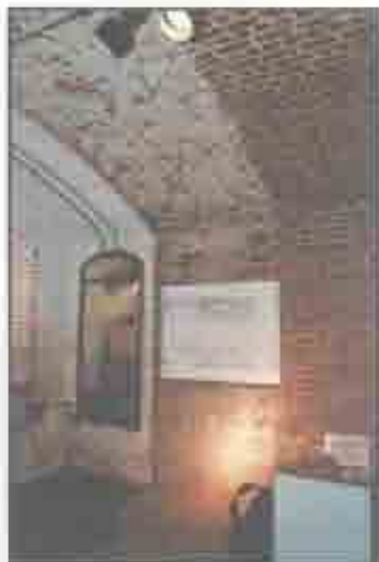
Walls were removed in the magazines during the conversion of the fort to a disciplinary barracks in 1914. Half of the 4-foot thick brick and rubble wall remains at right, while only the outline of a wall remains above. (John Martini, 2005)
