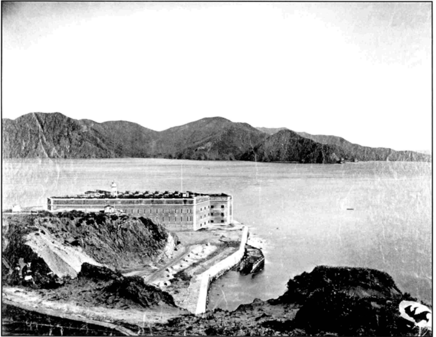
Figure 7. Photograph: Southeast view of Fort, circa 1868-1876. Credit: Fort Point NHS Collection, Golden Gate National Recreation Area.
