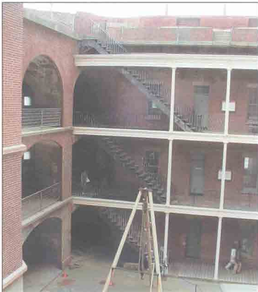
The cast iron staircase at the east end of the gallery is the only straight-run staircase in the fort. (Jane Lehman, 2005)
