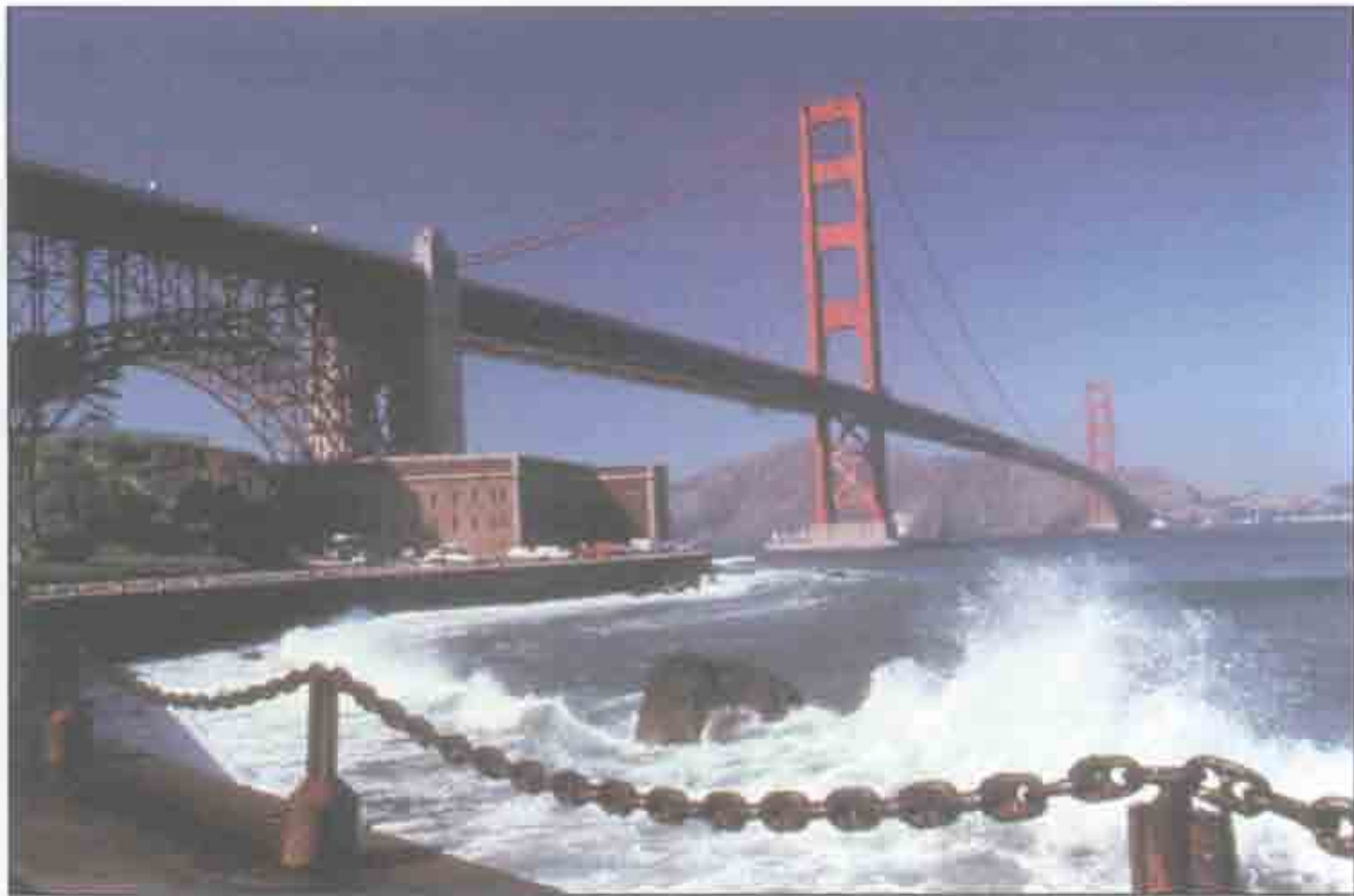
Above: Contemporary view of Fort Point, circa 2000. Credit: Golden Gate National Parks Conservancy.
