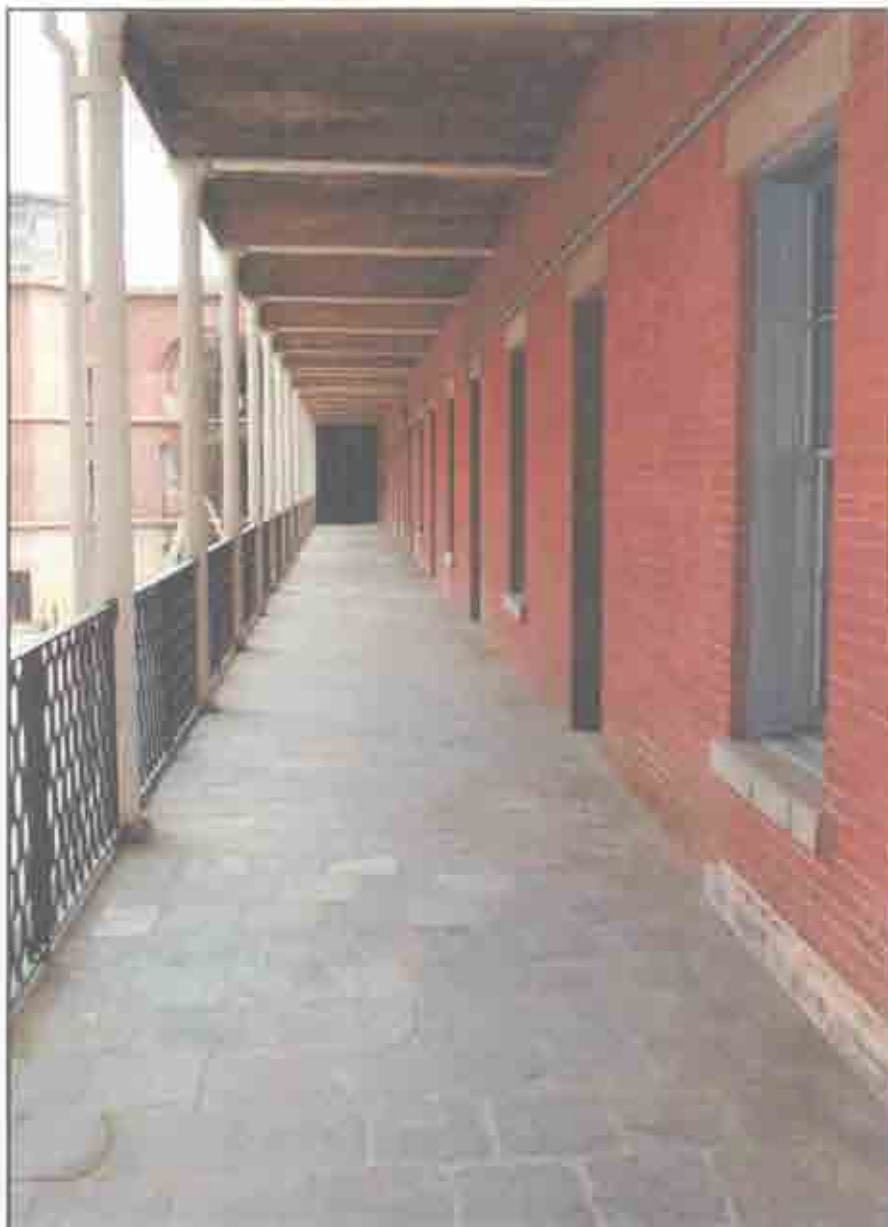
View of the 2nd tier gallery with its cast iron columns, brick ceiling, and slate floor. (John Martini, 2005)
