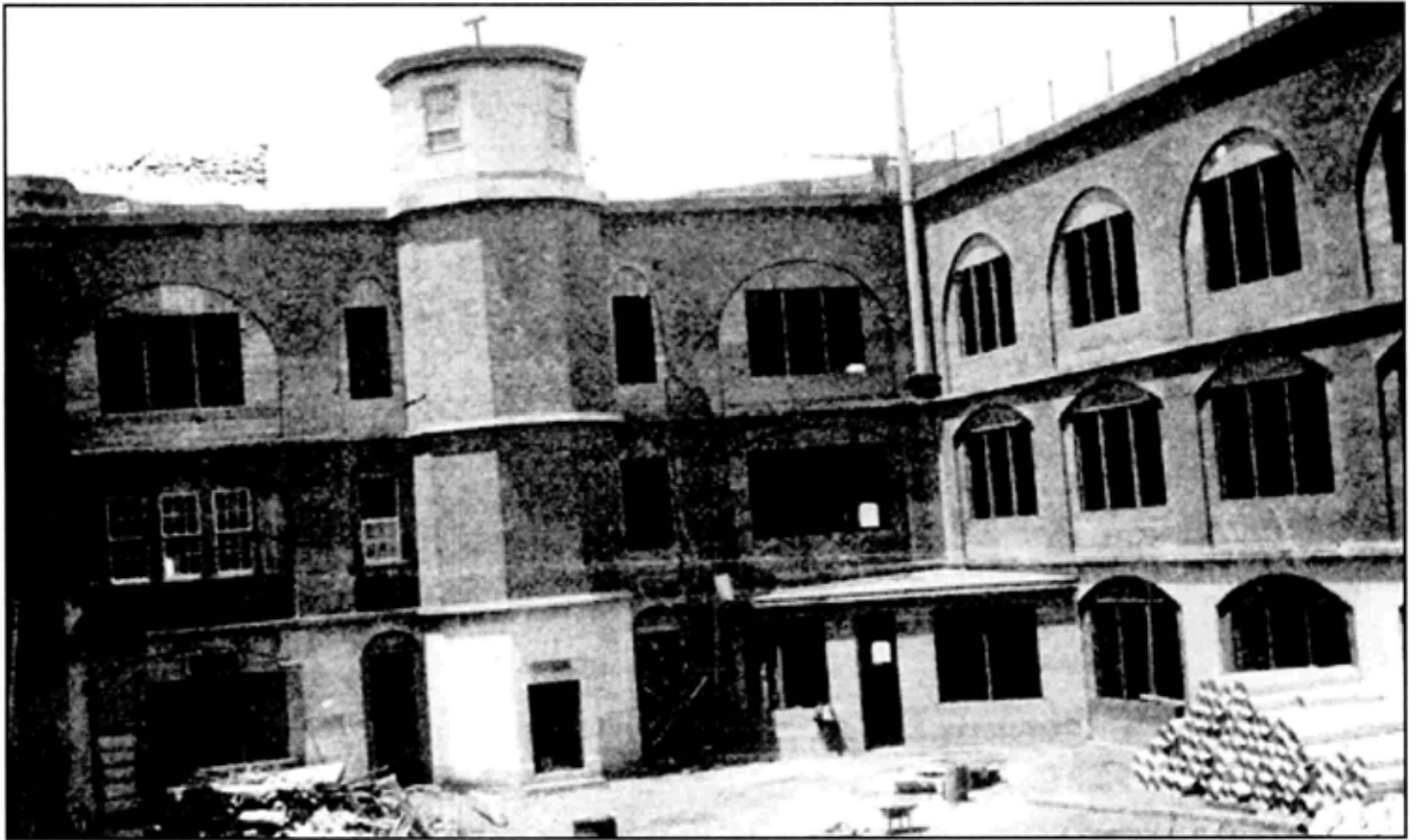
Figure 11. Photograph: Detention Barracks conversion in progress, viewed from the parade, circa 1914. Credit: Fort Point NHS Collection, Golden Gate National Recreation Area.
