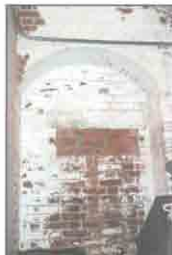
The rifle slit in the corridor of the jail area has been infilled with brick. (John Martini, 2005)
