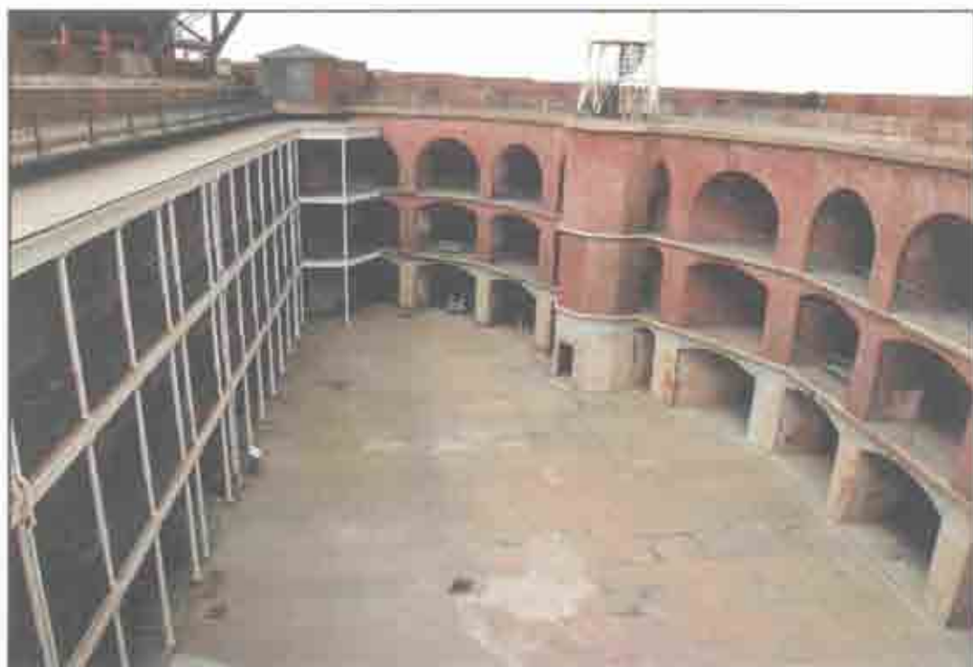
Interior courtyard elevation looking west. The southeast courtyard face is on the left and the lighthouse is partially visible on top of stair #2. (John Martini, 2005)
