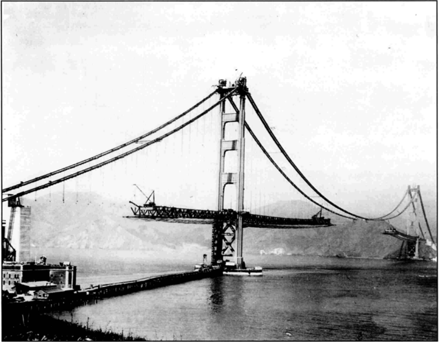
Figure 17. Photograph: Golden Gate Bridge construction, viewed from East, circa 1936. Credit: Fort Point NHS Collection, Golden Gate National Recreation Area.
