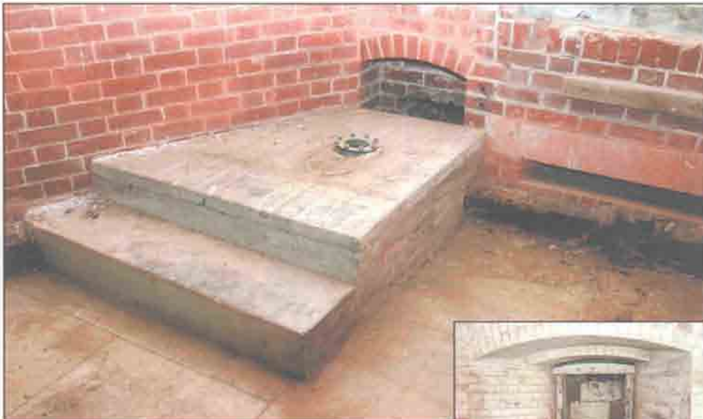
These concrete platforms for plumbing fixtures remain from the 1914 attempted remodel of the fort into a disciplinary barracks. (John Martini, 2005)
