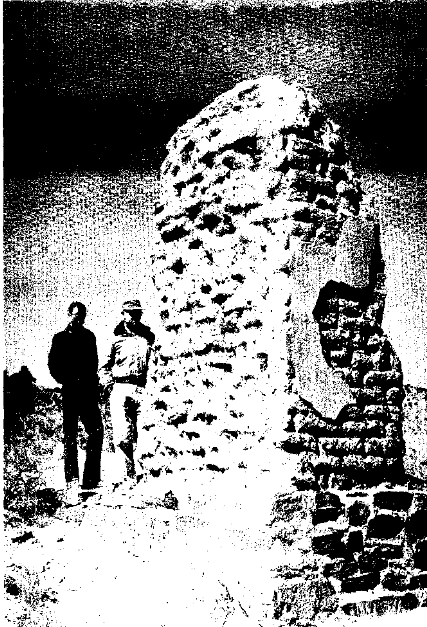
Photo No. 7 - Standing wall of the Hospital Stewards Quarters showing typical construction. Stone foundation, adobe walls and exterior plaster. McCole and Benson in photo. Arnberger, 1957.
