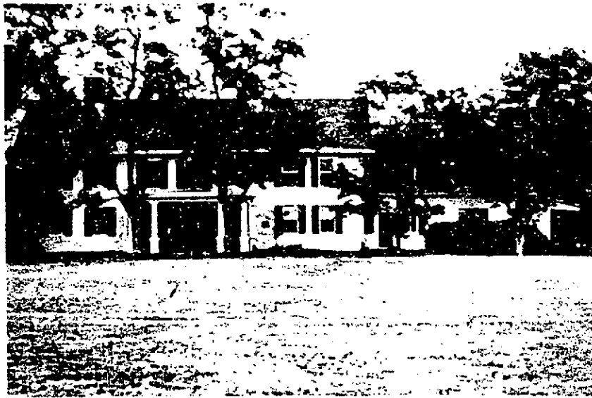
FRONT (SOUTH) VIEW, FLOYD HOUSE
