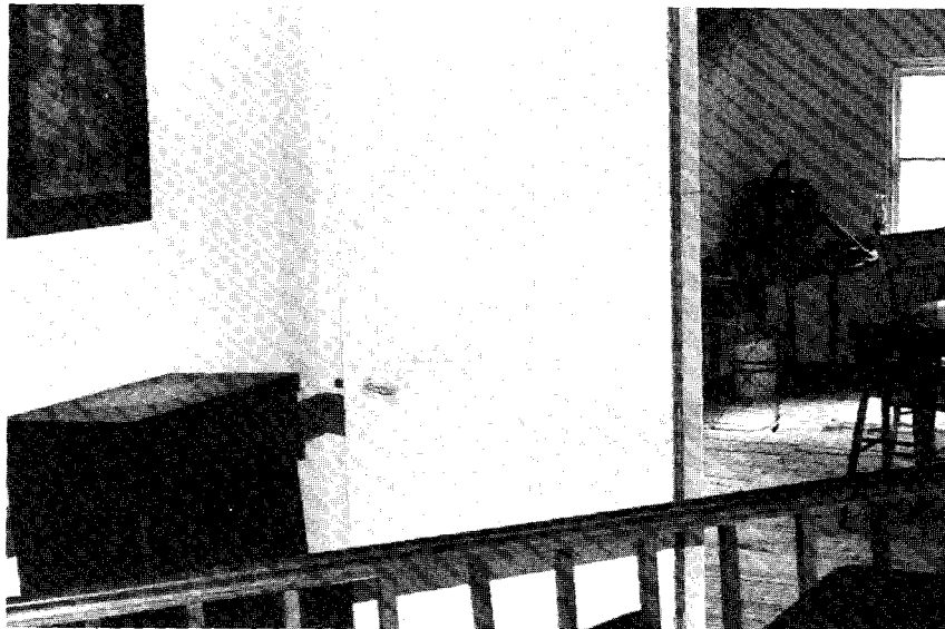
Northwest Corner - Room 105
