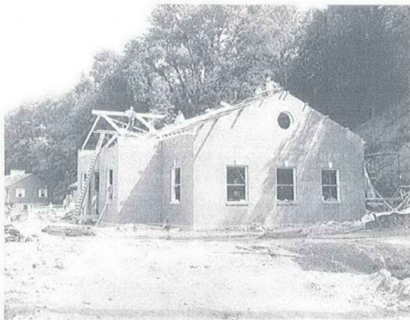
Figure 7: Wright Hall under construction, 1948-50 (Carillon Park Archives)
