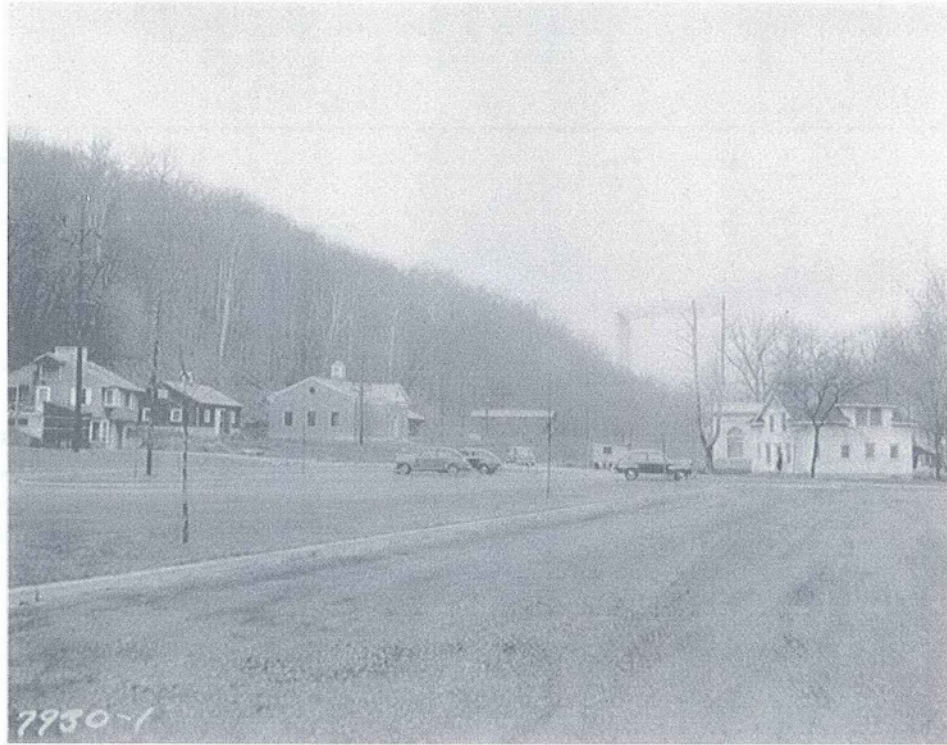
Carillon Historical Park during the construction of Wright Hall, ca. 1948-50 (CHP Archives)
