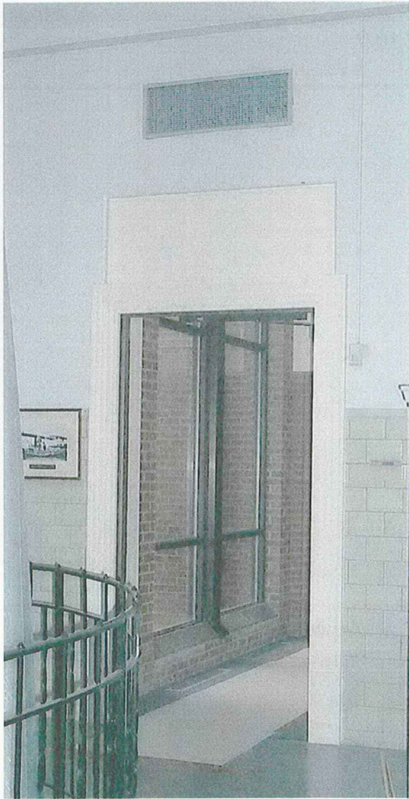
Wright Hall, interior, opening to new connector building (QE\A 2000)
