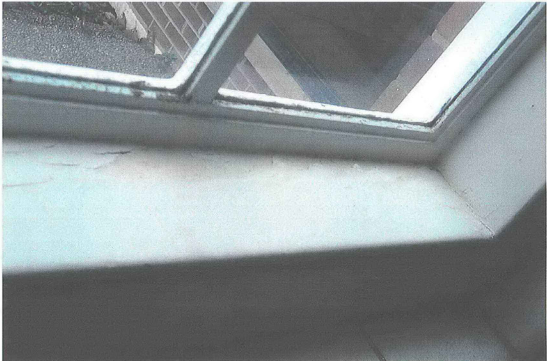
Wright Hall interior, typical window condition (QE\A 2000)
