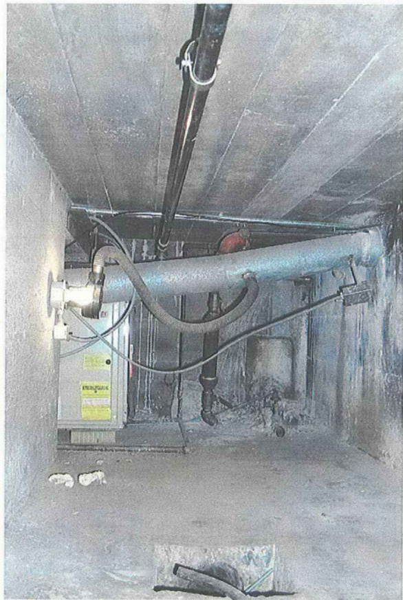
Wright Hall east plenum, looking south (QE|A 2000)
