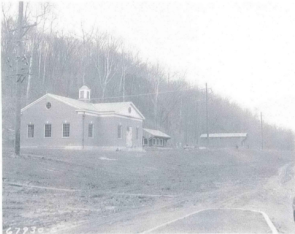
Wright Hall from the northeast, under construction, ca. 1948-50 (CHP Archives)
