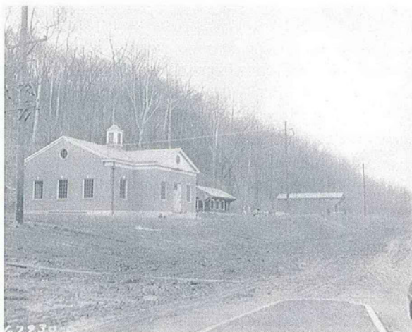
Figure 8: Wright Hall under construction, 1948-50 (Carillon Park Archives)
