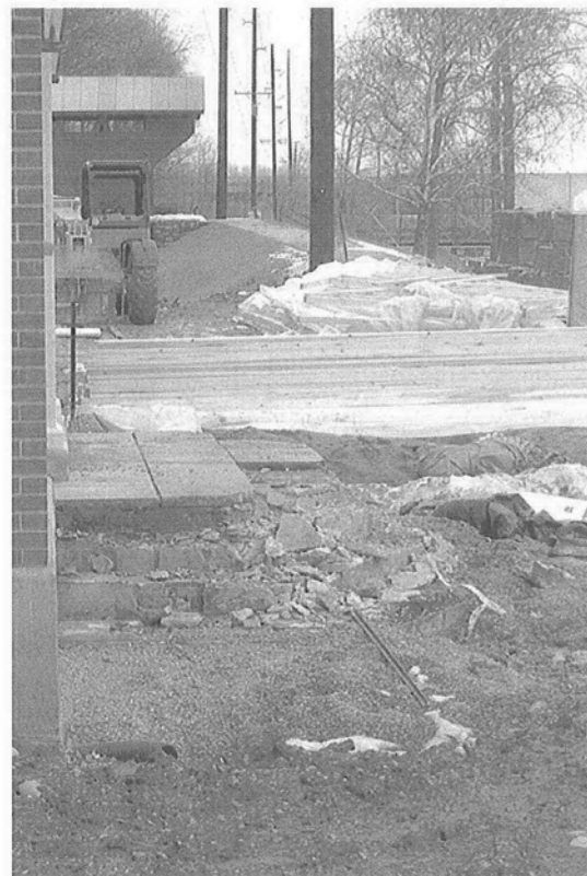
Figure 27: Dismantled front steps.
