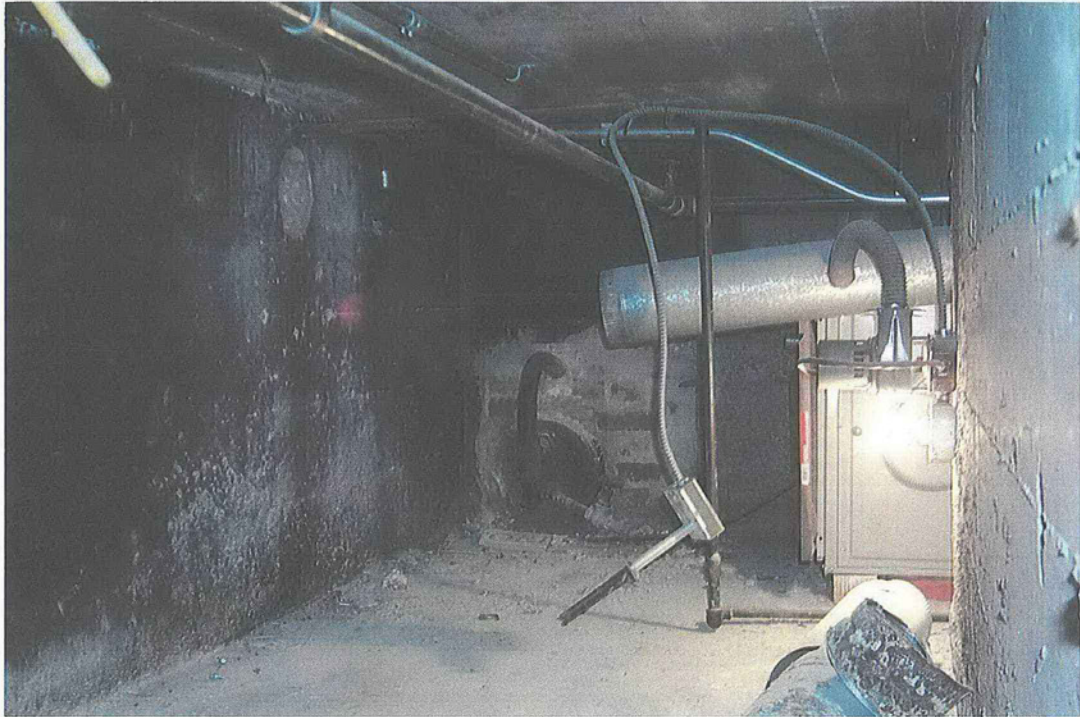
Wright Hall south plenum, looking west (QE\A 2000)
