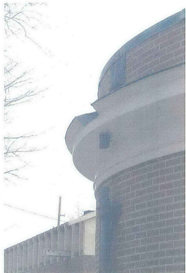
Wright Hall apse exterior, cornice detail, looking west (QE|A 2000)
