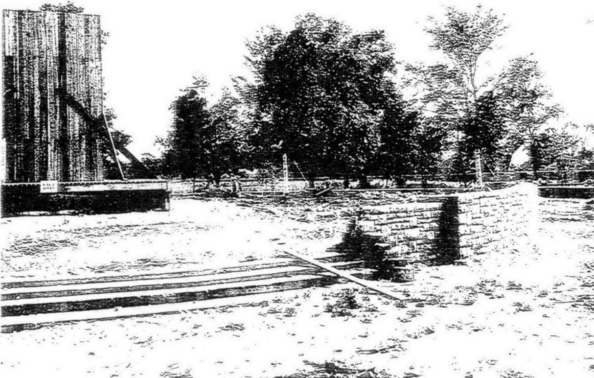
Photo 6: Memorial Plaza under construction, circa 1939-40. (Courtesy of Miami Conservancy District.)
