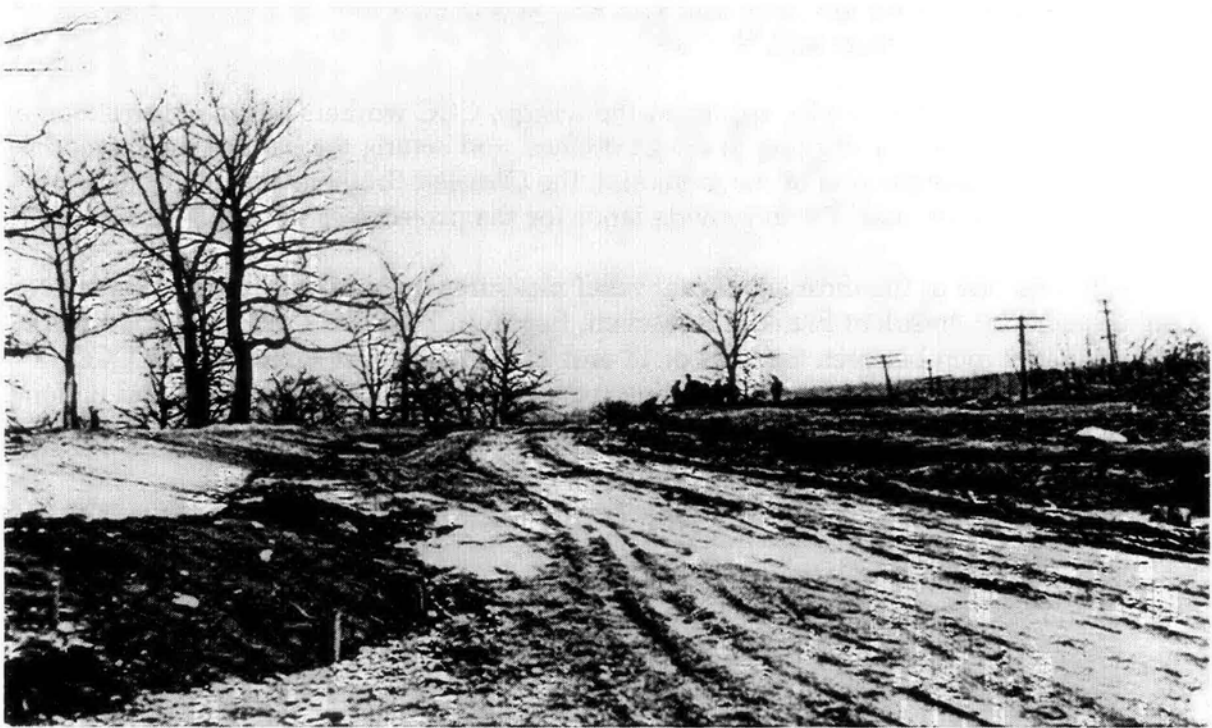
Photo 3: Entry road under construction, circa 1938. (Courtesy of Miami Conservancy District.)
