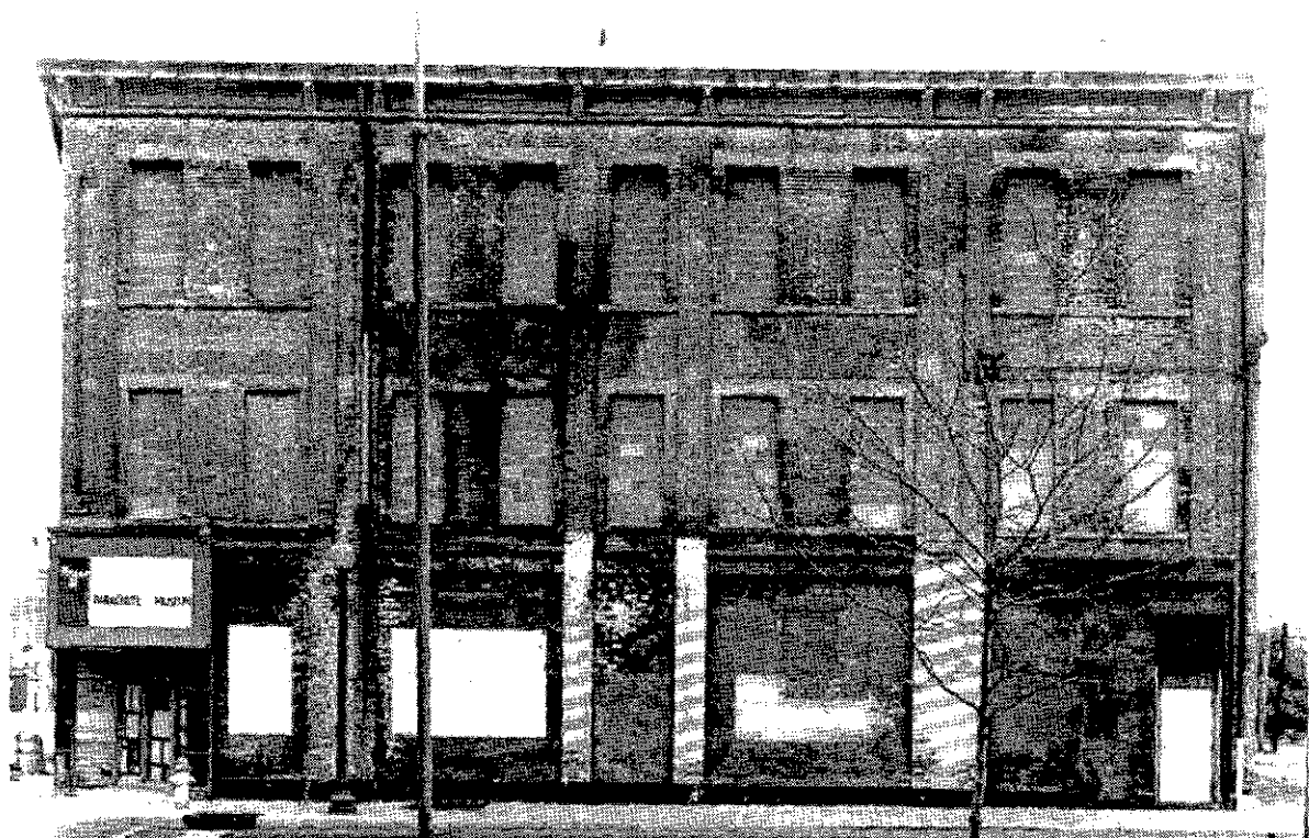
Figure 23 View of the west elevation of the Hoover Block (J. Miles Wolf, 1995).
