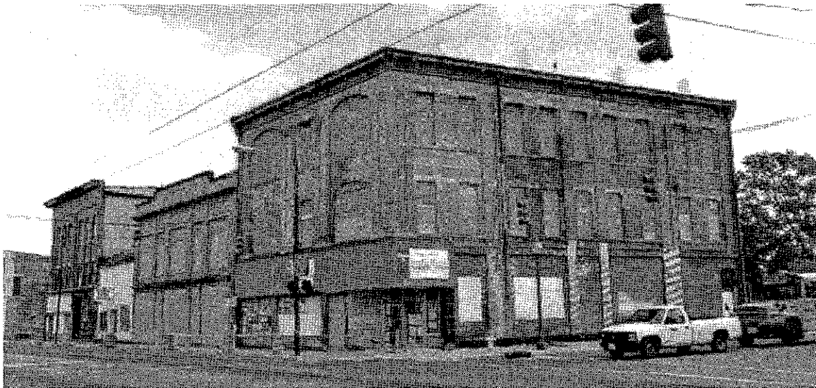
Figure 7 View looking southeast from the northwest corner of the intersection of West Third Street and South Williams Street. The Hoover Block is at the corner, and the Setzer Building is next door, now with a brick facade. (Quinn Evans/Architects, 1995)
