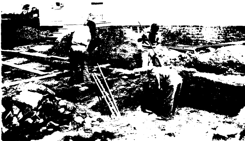
Excavating an old marl cellar pertaining to a house which probably ante-dated the present house
