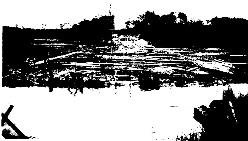
King Creek Bridge under construction, looking east
