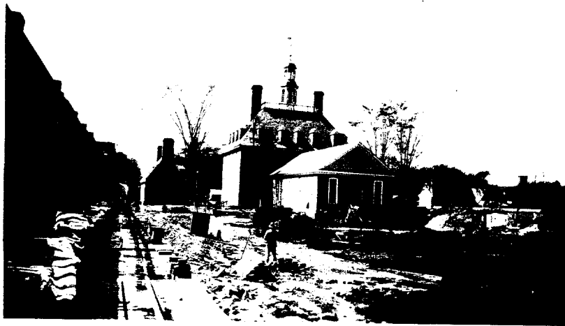
Governor's Palace - Restoration work underway (III,ii,B)
