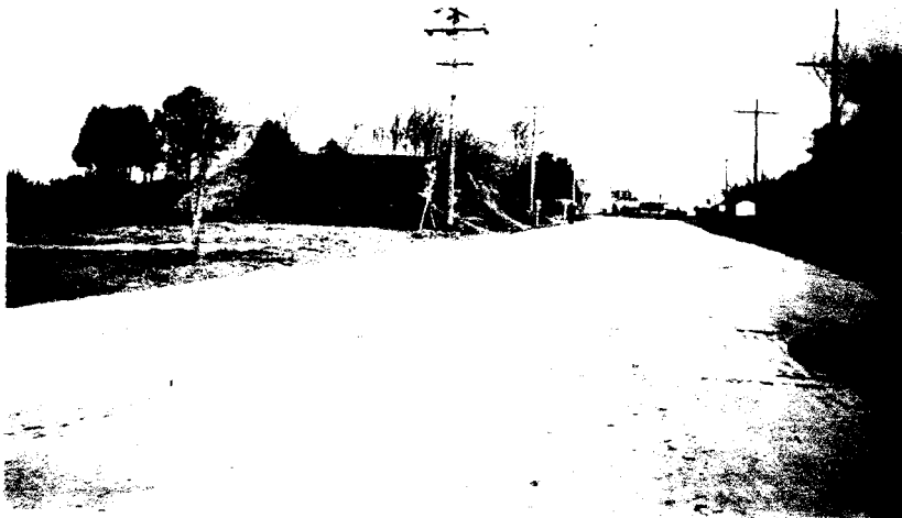
Exterior, looking in, northward
