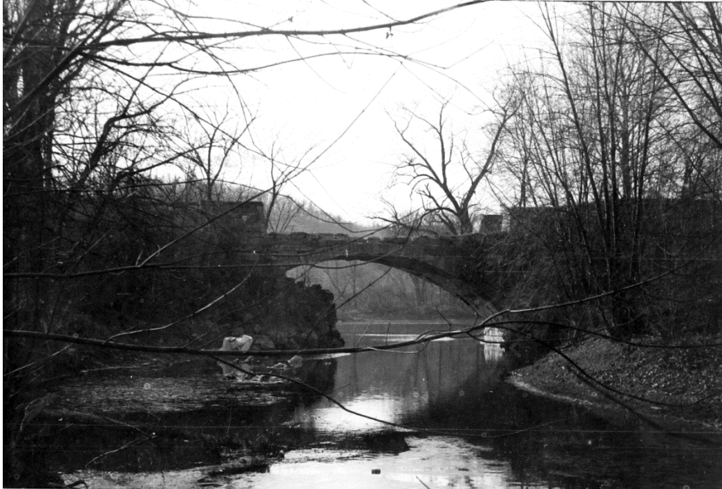
5: Tonoloway Aqueduct, November 1965, HABS Photo by C. R. Parkinson. This is Photograph 3 only taken a little further back to give perspective. This seems to be identical to Plate IV on page 29, except for the data.
