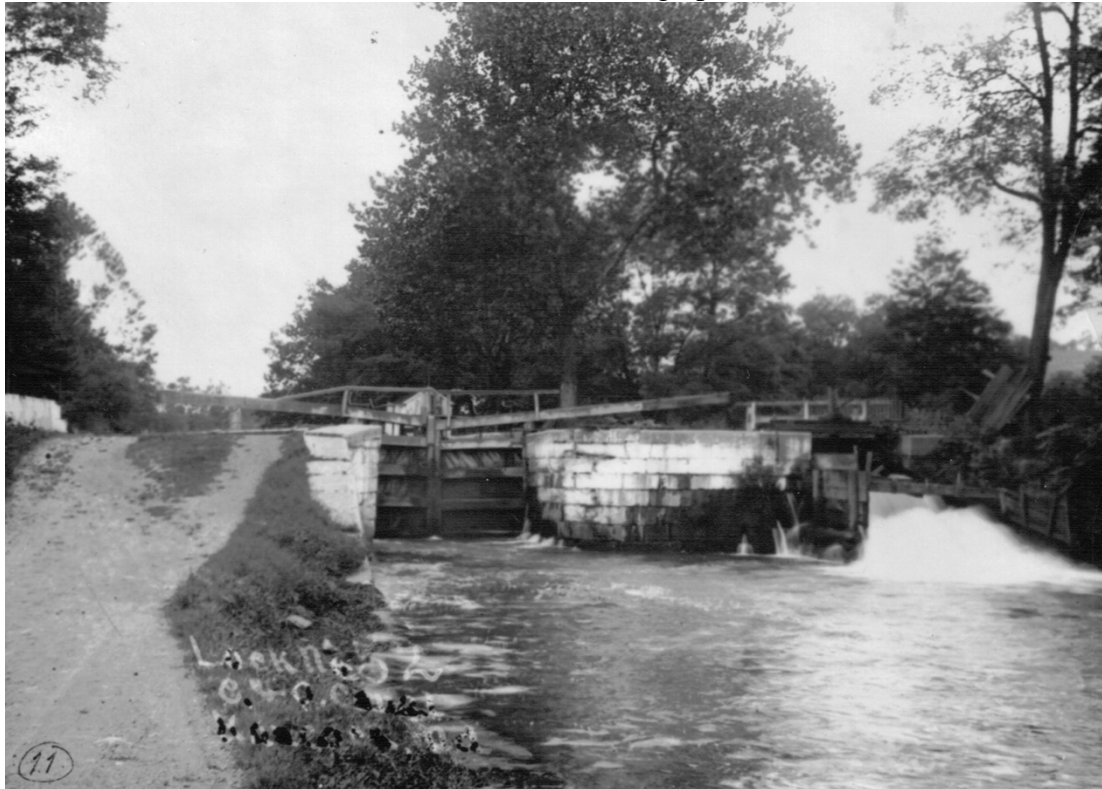
6: Lock 52, ca 1900, looking upstream.
