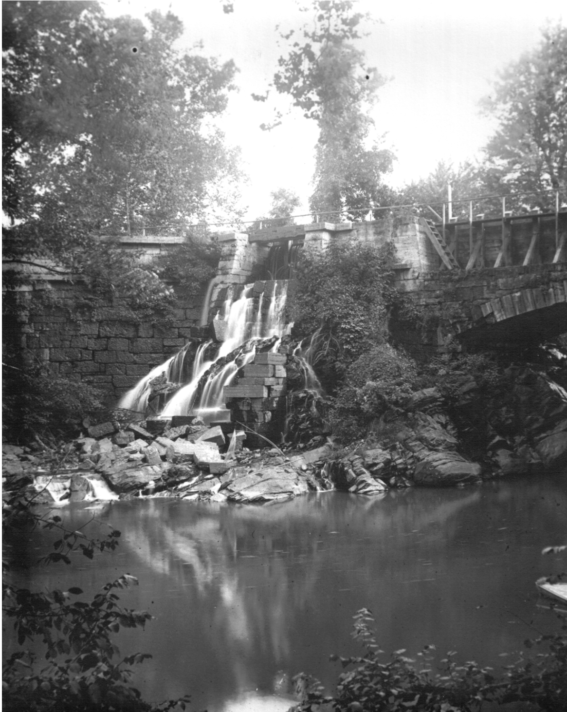
1: Tonoloway Aqueduct waste weir, mid-1930's. Note that the berm side wall has washed out and the wooden trunk is in place.
