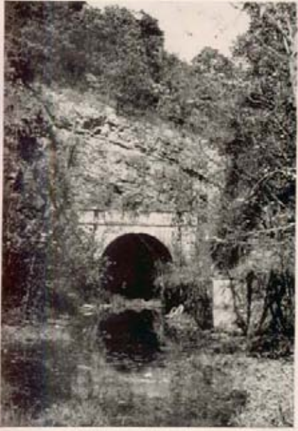
Canal formed by Fall Dam, north pier.
