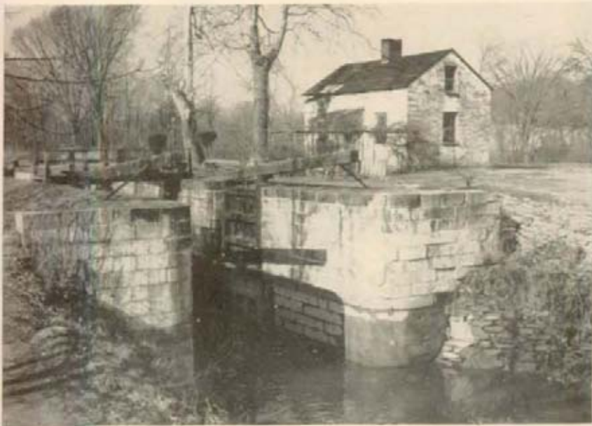
Typical lock house and lock.
