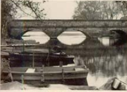
Canal aqueduct across the Seneca River.
