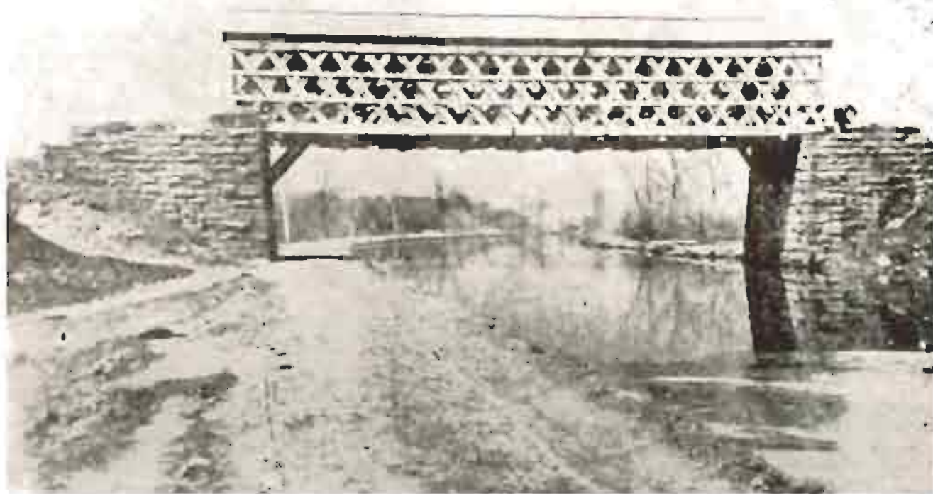
OLD COVERED BRIDGE —Here is a picture of an old wooden bridge over the C&O Canal near Cumberland. Note the stone work and the fancy framework of this old structure.
