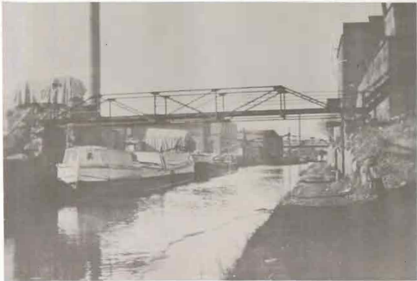
IV. Pedestrian Bridge East of the Georgetown Market at Potomac Street, Looking West. This photograph was made about the turn of the century, after the wooden bridges were replaced by a steel structure.
