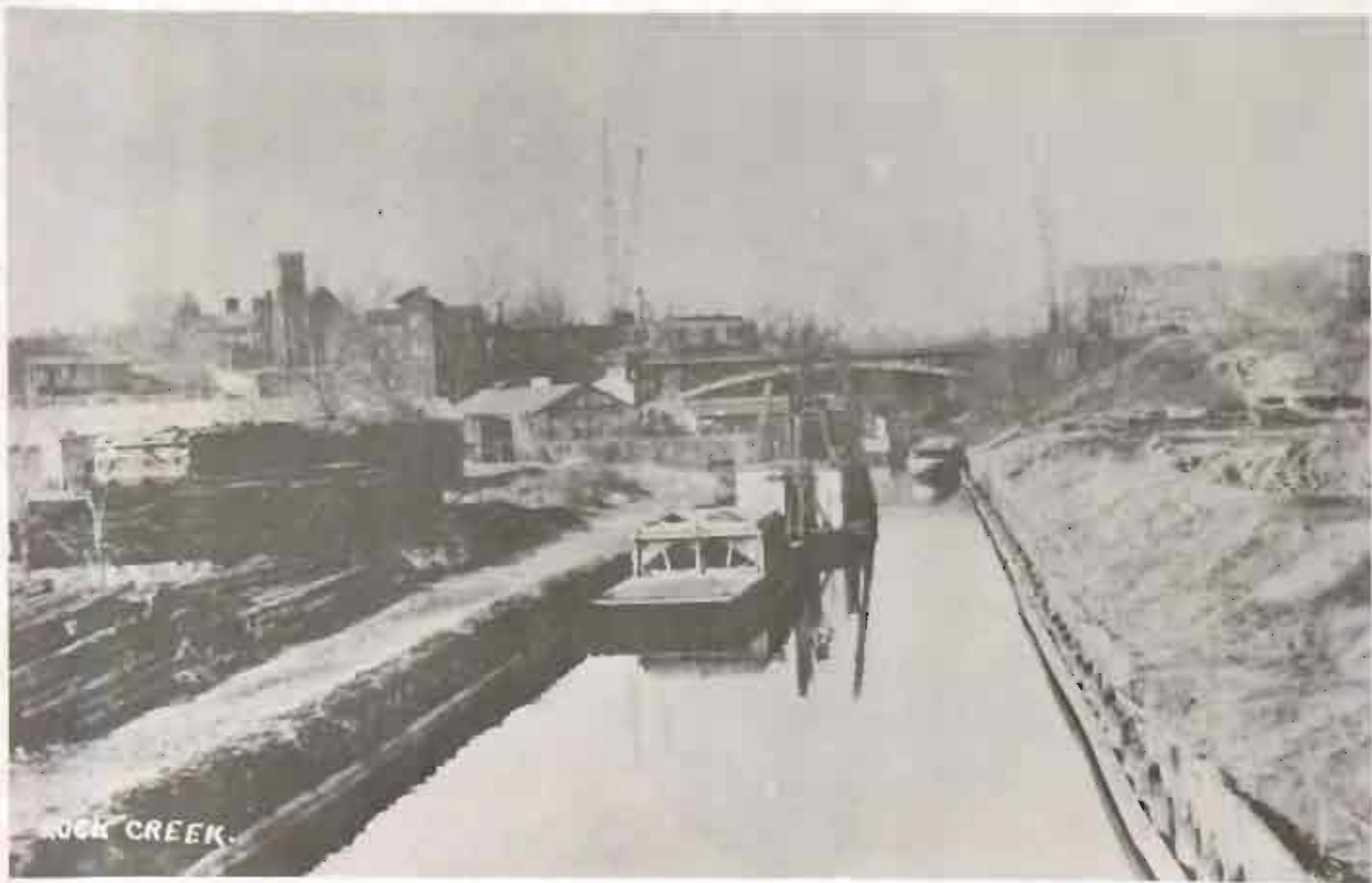
III. K Street Bridge Across Rock Creek, Circa 1861-1865, Brady-Handy Photograph, Library of Congress Collection.
