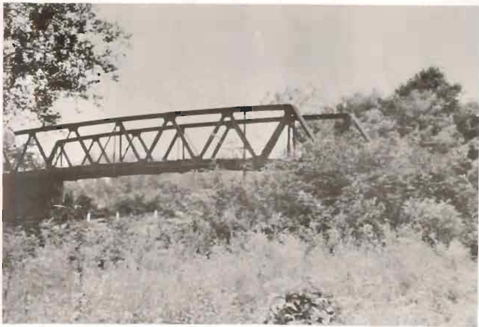
XV. Iron Bridge at White's Ferry, built in 1876. Photograph from files C&O Canal National Monument.
