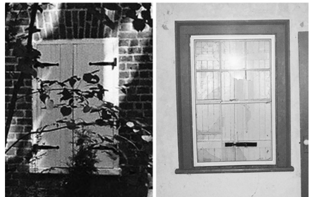
Window 2, exterior and interior
