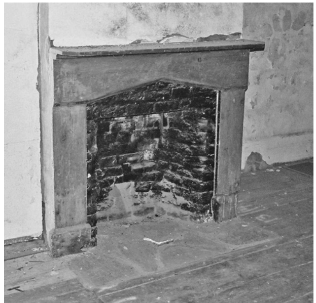
FIGURE 67. Fireplace in Room 107.
