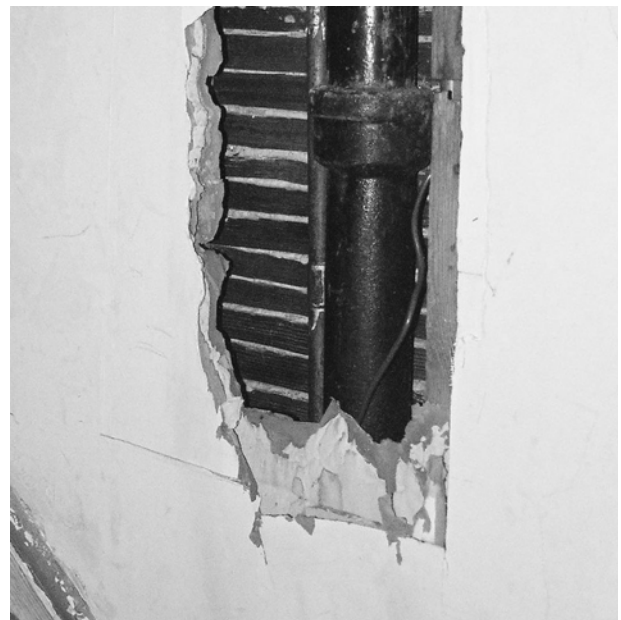
FIGURE 22. East wall of stairwell in Room 102. Note gypsum board wall finish.
