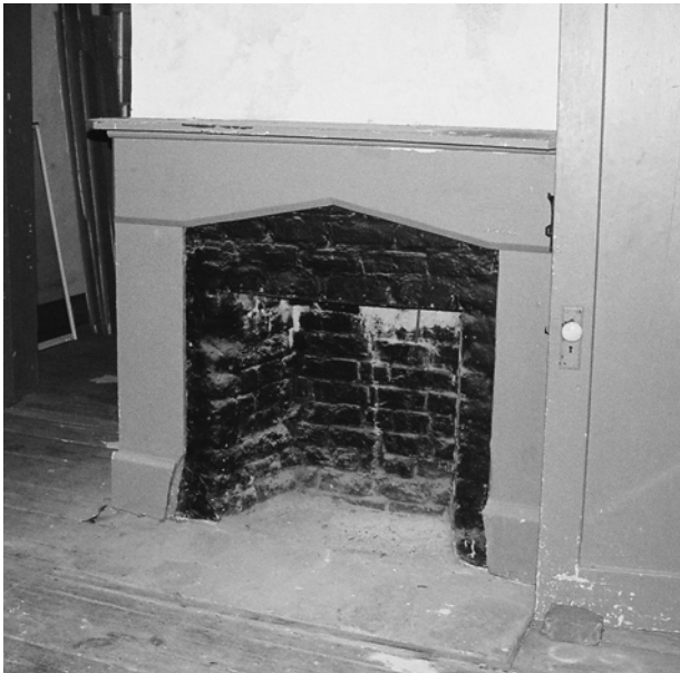
FIGURE 60. Fireplace in Room 104.
