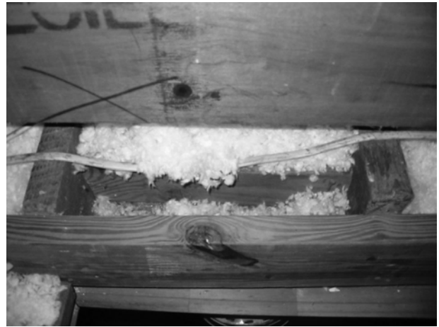
FIGURE 20. Floor joists in attic.
