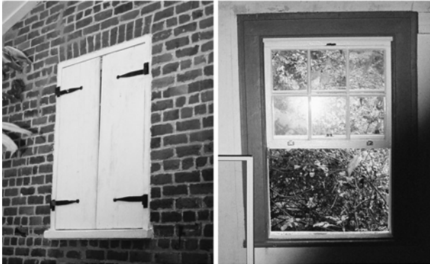
Window 7, exterior and interior
