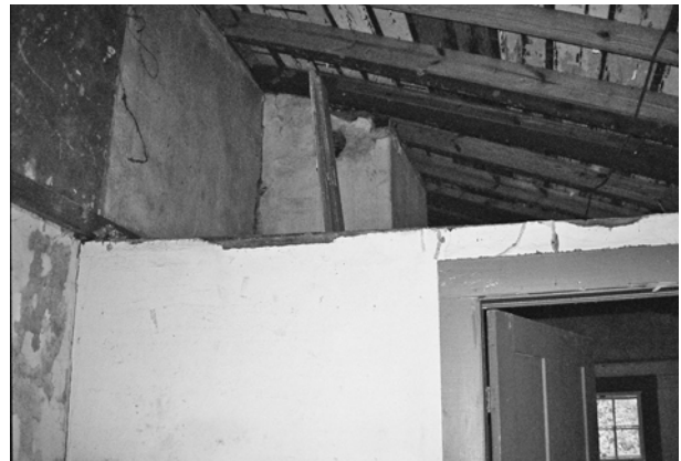
FIGURE 63. Detail of truncated west wall in Room 105, looking towards Room 107.
