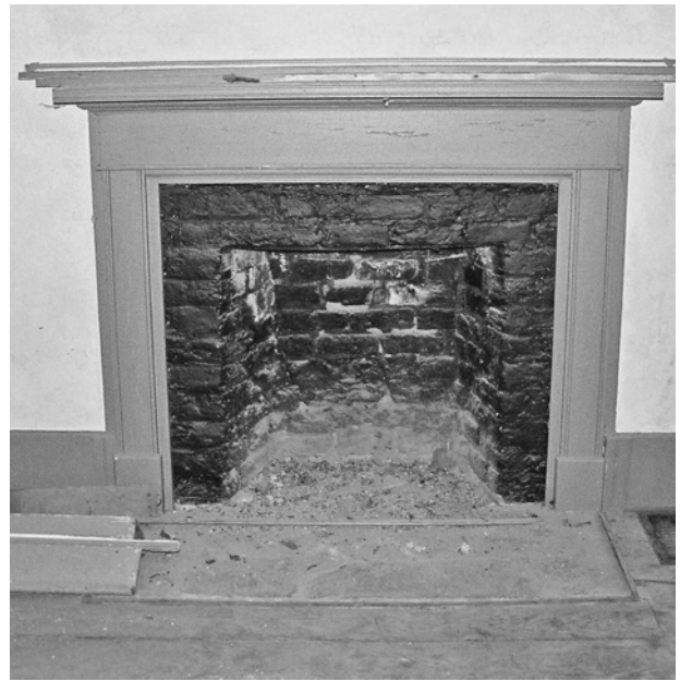
FIGURE 51. Fireplace in Room 101.
