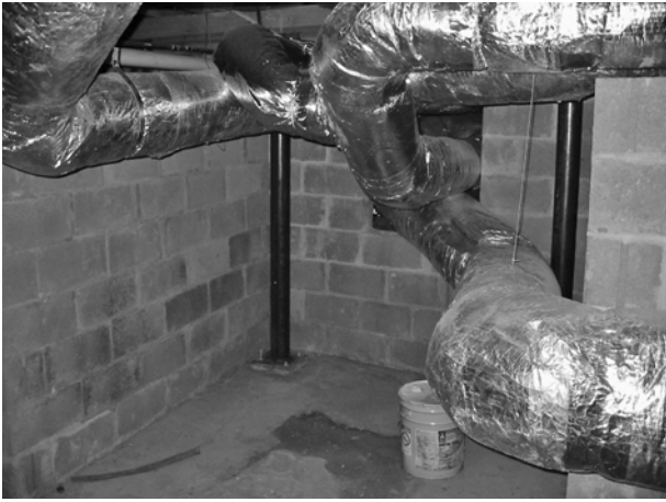
FIGURE 17. Concrete block retaining wall along south side of excavated basement.
