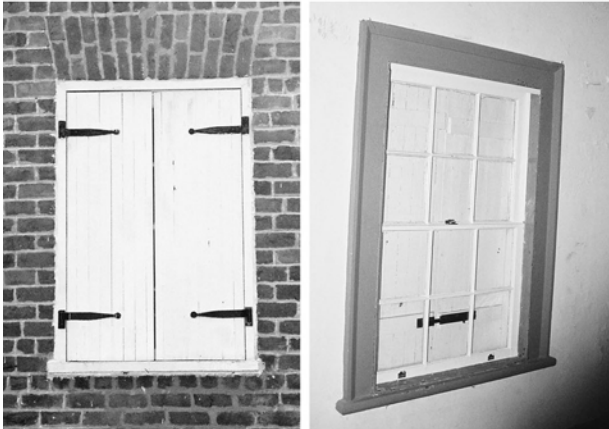
Window 8, exterior and interior
