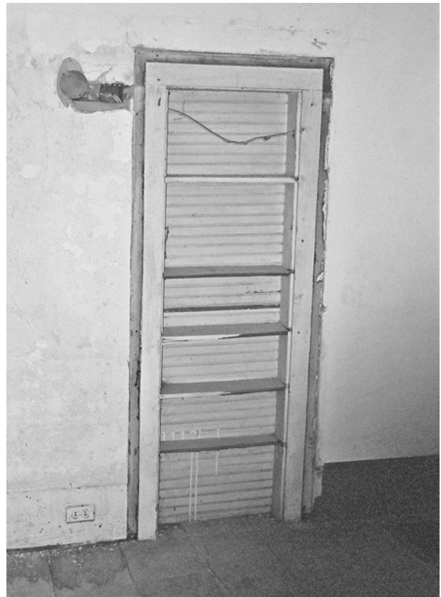
FIGURE 56. Built-in case on west wall of Room 103.
