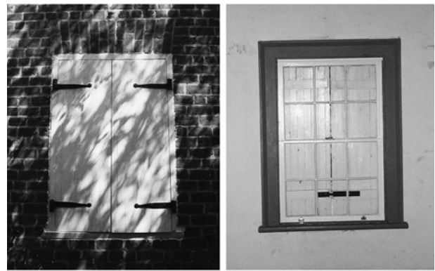
Window 1, exterior and interior
