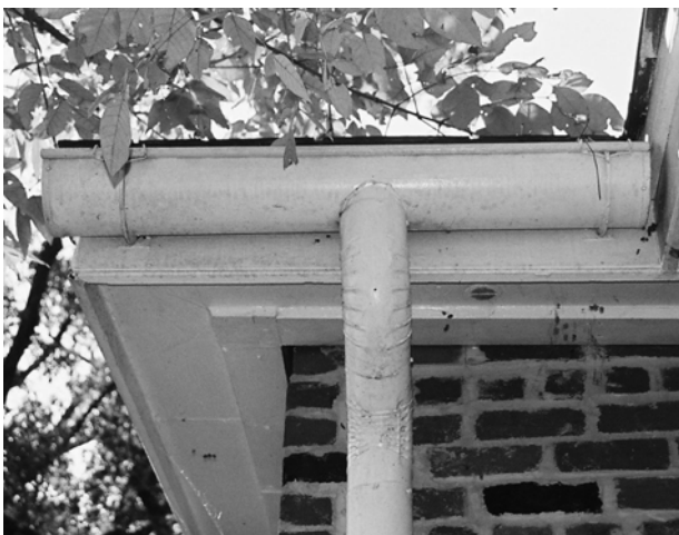
FIGURE 34. Gutter and downspout at northeast corner.
