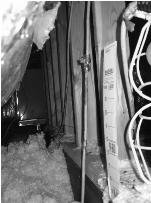
FIGURE 23. Posts and beam providing central support to hipped roof.
