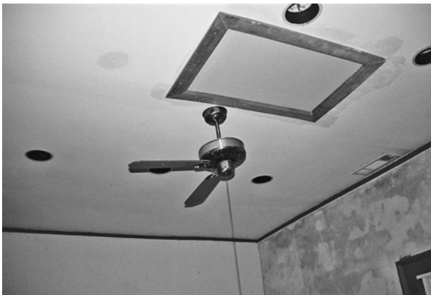
FIGURE 78. Ceiling in Room 114.
