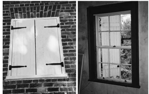
Window 12, exterior and interior
