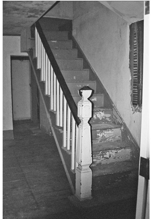
FIGURE 52. View of staircase in Room 102.
