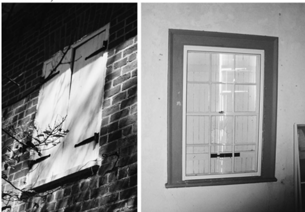
Window 9, exterior and interior
