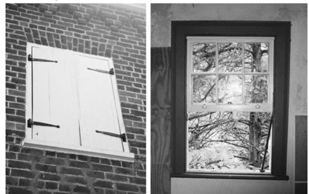
Window 13, exterior and interior
