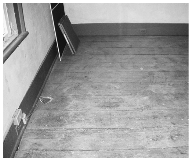
FIGURE 76. Flooring in Room 114.
