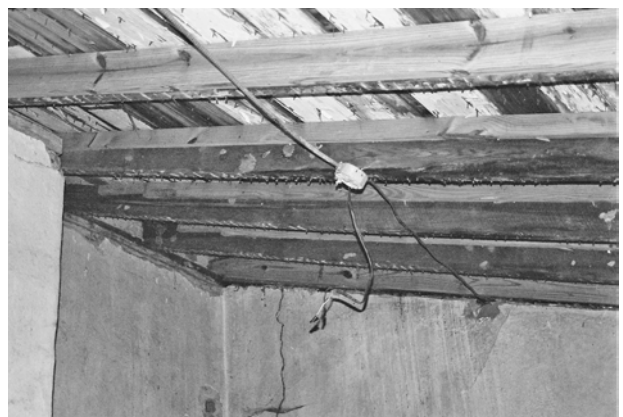
FIGURE 68. View of exposed roof framing in Room 107.
