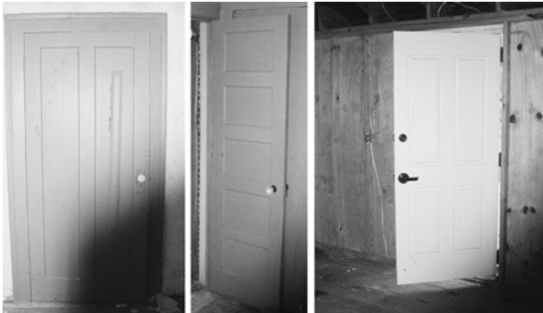
FIGURE 59. Doors 5, 6, & 7 in Room 104.
