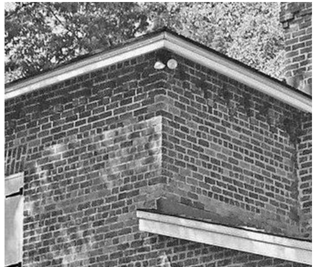
FIGURE 30. View of southeast corner.
