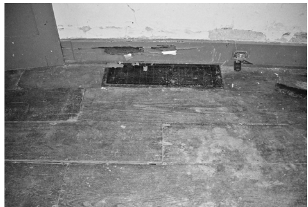
FIGURE 57. Flooring in Room 103.
