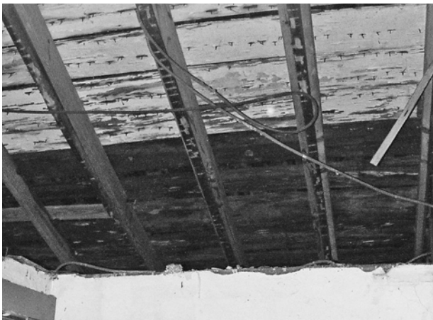
FIGURE 24. Shed roof framing as seen from Room 106.
