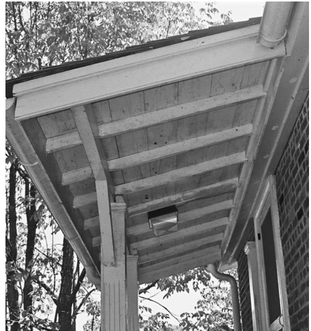
FIGURE 25. Framing for shed roof at rear stoop.
