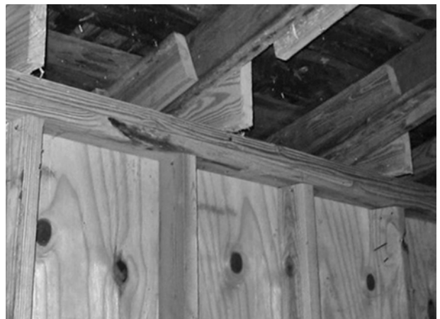
FIGURE 21. New north wall framing in Room 104.
