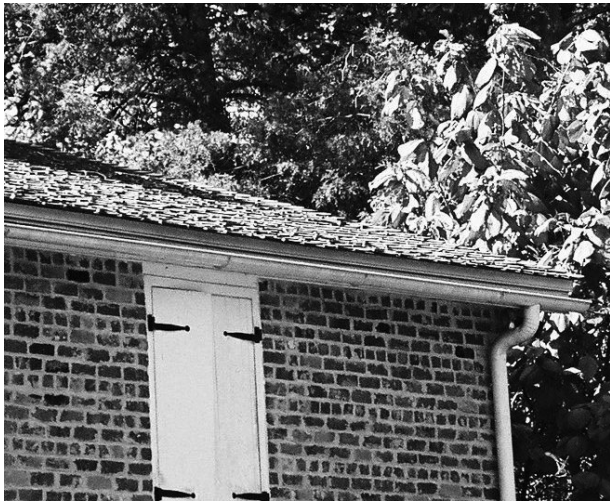
FIGURE 33. Cedar shingle roofing on shed-roofed addition.
