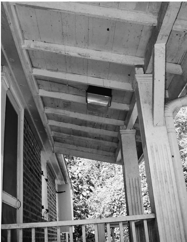
FIGURE 28. Stoop located at rear entrance to house.
