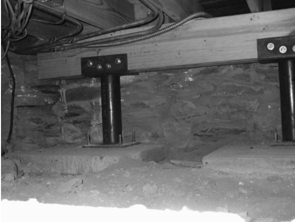
FIGURE 18. New 2" by 10" supplementary support beams at north, two-story wall.
