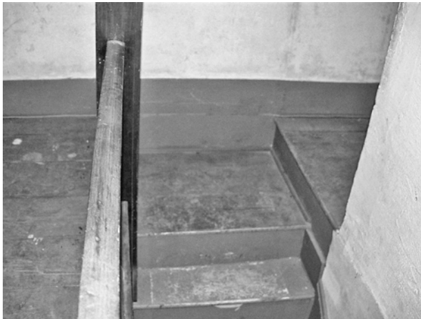
FIGURE 74. Over view of landing at top of stairs in Room 112.
