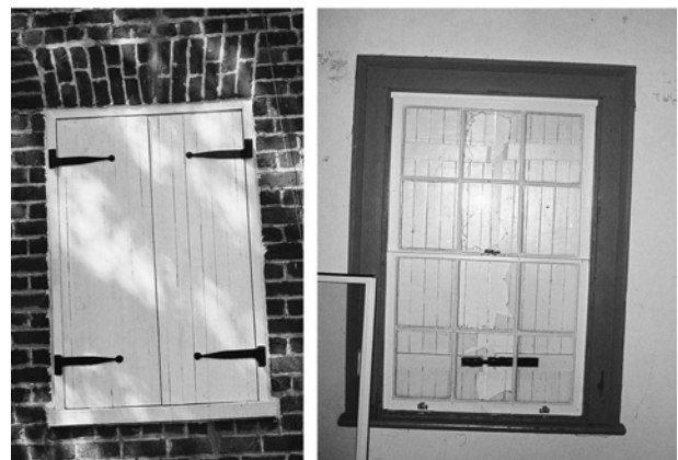
Window 3, exterior and interior
