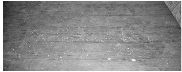
FIGURE 70. Flooring in Room 110.
