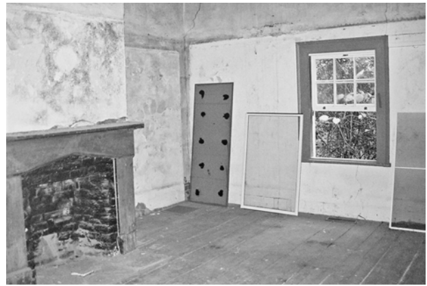
FIGURE 66. View of Room 107, looking west.
