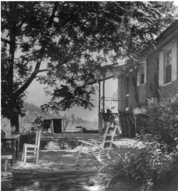
FIGURE 11. North elevation and rear yard, 1940. Source: Roswell Historical Society.
