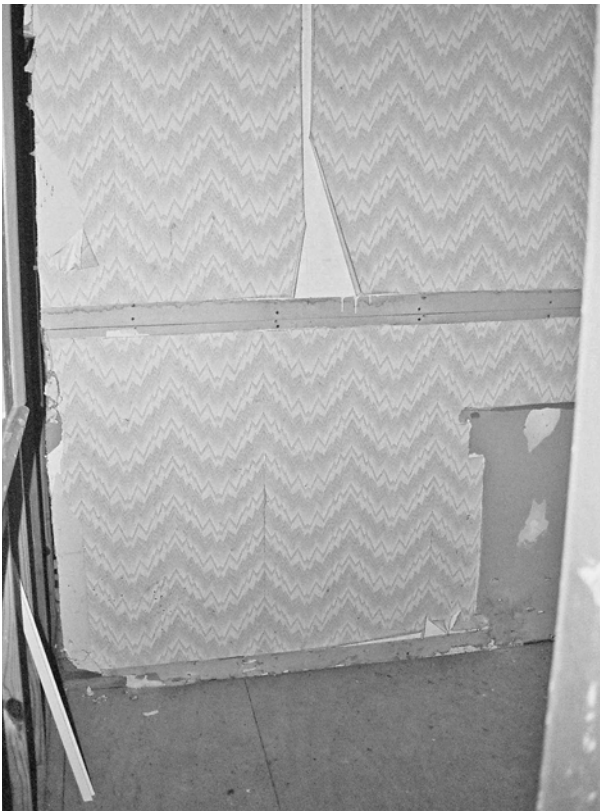
FIGURE 64. East wall in Room 106.
