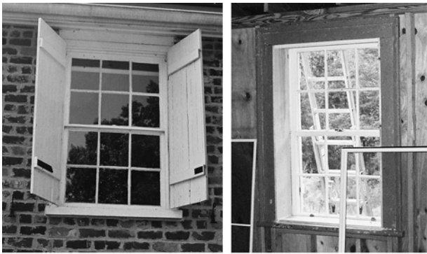
Window 6, exterior and interior
