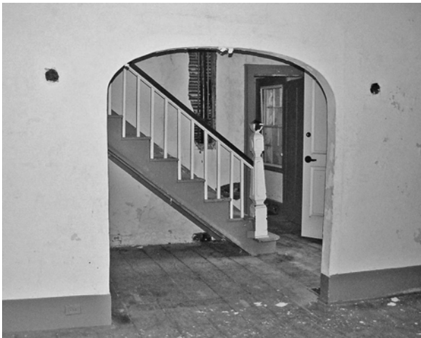
FIGURE 49. Arched opening in east wall of Room 101.
