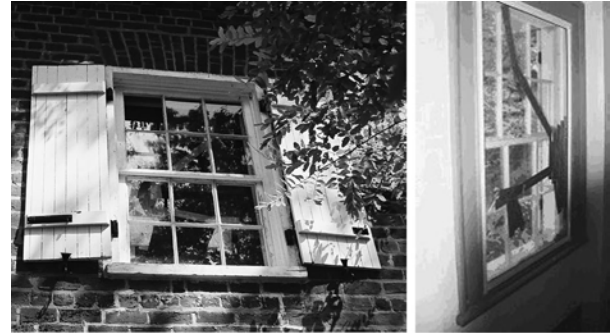
Window 10, exterior and interior
