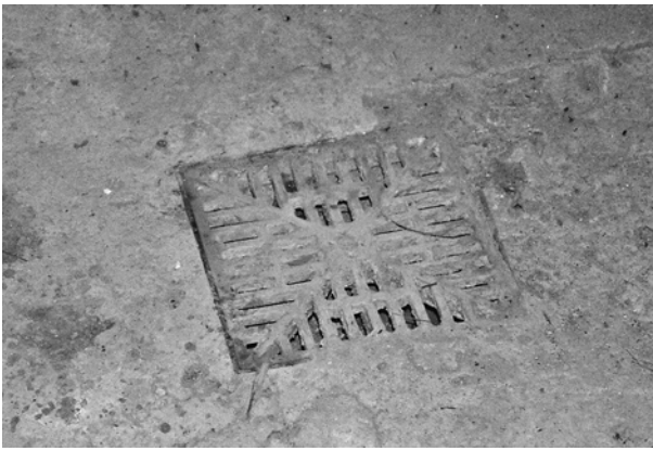
FIGURE 48. Grate in basement floor.
