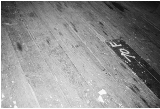
FIGURE 58. Flooring in Room 104.
