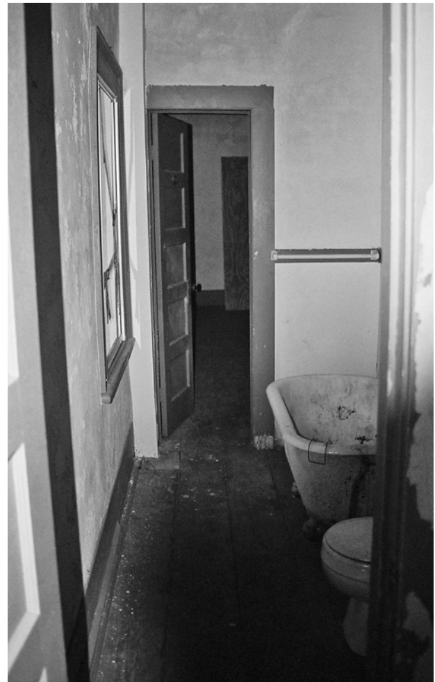
FIGURE 75. Overview of second-floor bathroom, Room 113.
