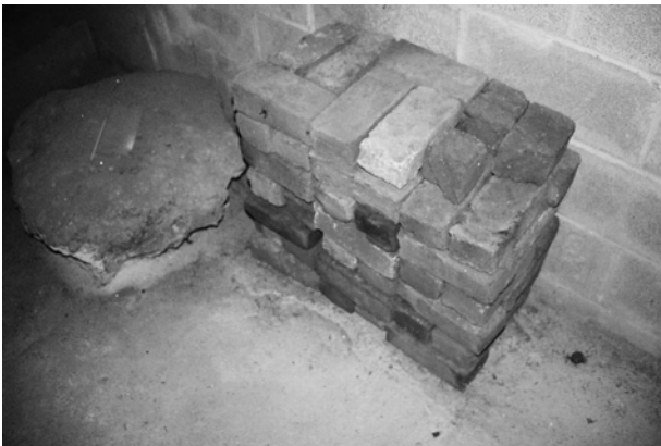
FIGURE 19. Bricks stacked in basement.
