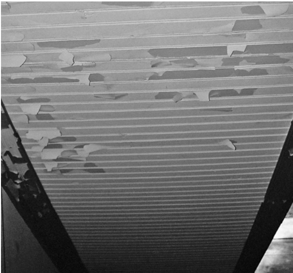
FIGURE 54. Beaded-board paneling on underside of staircase.
