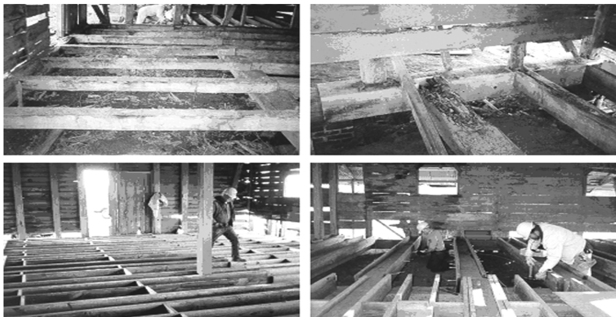
Figure 14. NPS rehabilitative work on the floor framing system of the Seed House, 1999. Note sistering of historically sloped floor beams to achieve level floor surface.
