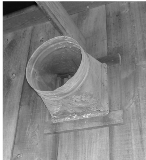
Figure 48. Transition fitting located on south elevation.
