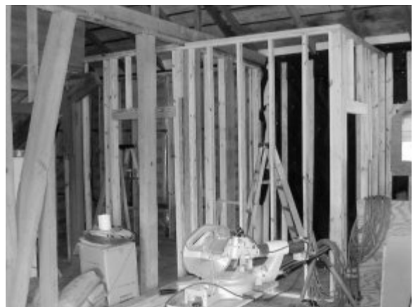
Figure 52. Framing for restroom and storage room in Seed House.
