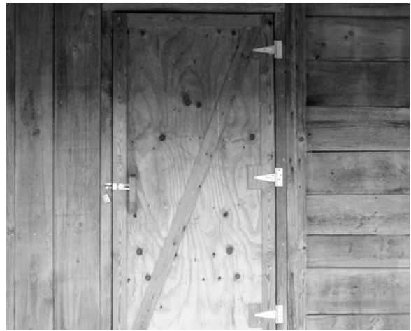
Figure 42. Detail of exterior siding, south elevation. Note the differing materials on either side of the door.
