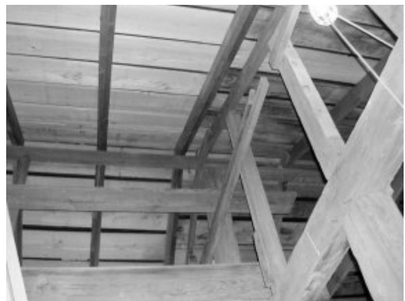
Figure 43. Detail of roof rafters and sheathing, west end.
