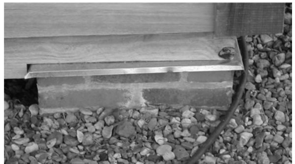
Figure 24. Typical perimeter Pier/ Post 1999.
